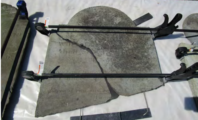
Above: The gravestone of Mrs. Ann Kiley before being conserved. Below: The two parts are glued together with an epoxy adhesive and clamped together while the epoxy cures.
