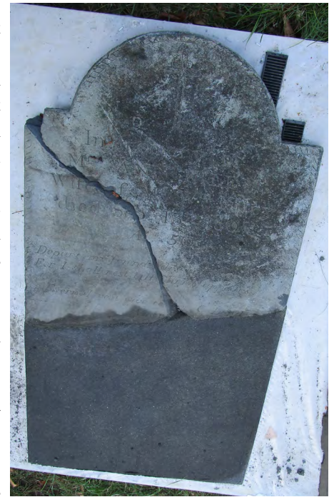
The missing bottom piece of the headstone is replaced with tinted concrete in order to reset it at the correct height in the ground.
