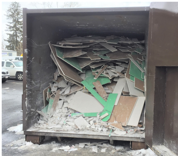
Collecting gypsum wallboard in a separate, covered container helped recycle 20 tons of this material.
