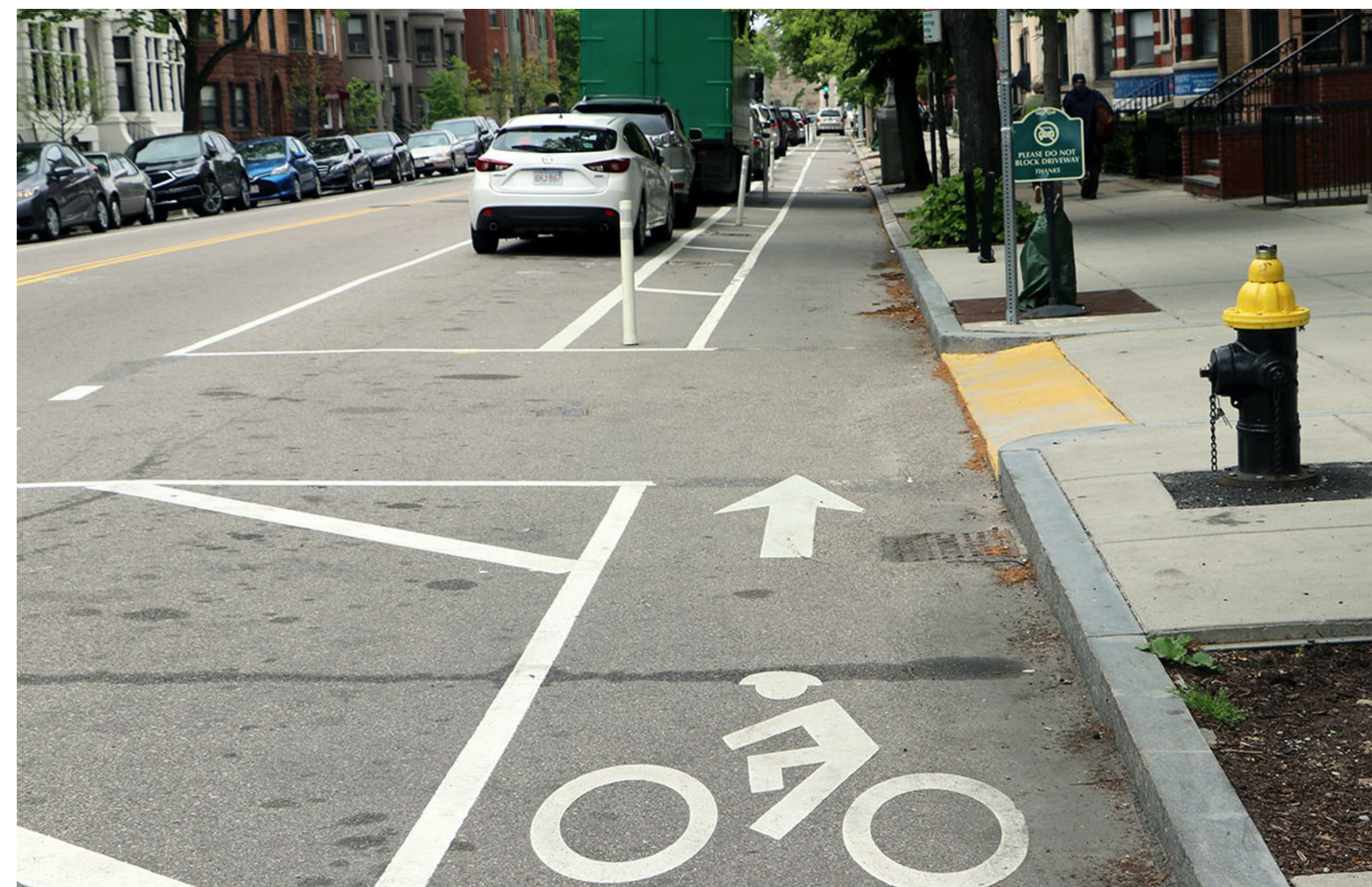
Parking protected bike lane (Beacon Street).
