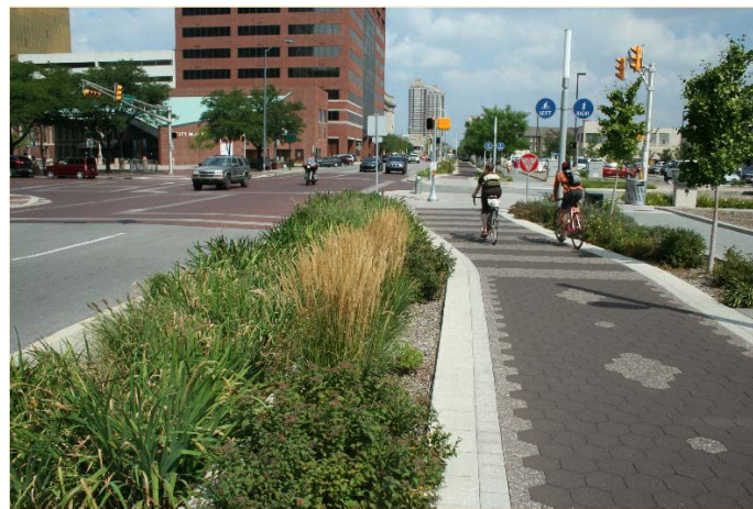
Stormwater Planters Image Source: Clark Wilson, USEPA
