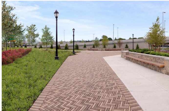
Pervious Paving GREEN INFRASTRUCTURE
