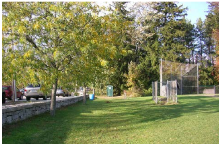
Dry Swale Adjacent to Ball Field Image Source: Horsley Witten
