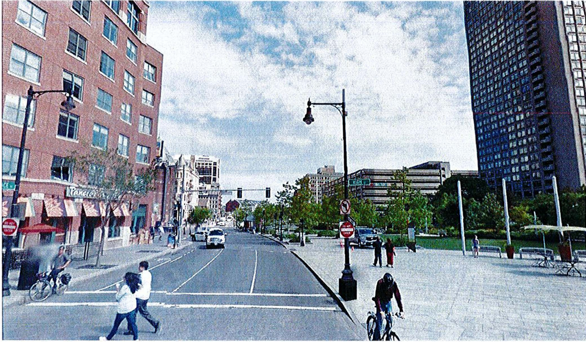
Example of pendant light pole with approved wireless facility installed
