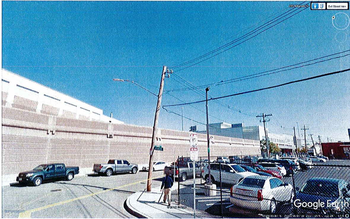
Example of wood utility pole (side mount)
