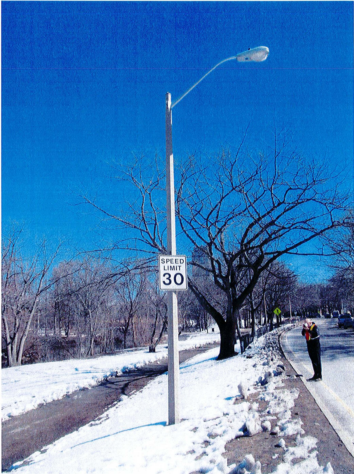
Example of standard steel light pole
