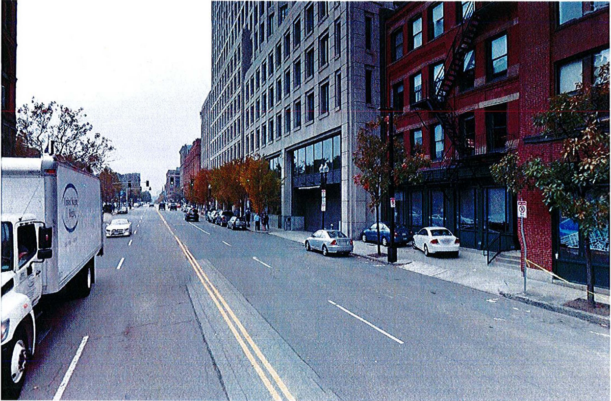
Example of aeriata steel light pole with approved wireless facility installed
