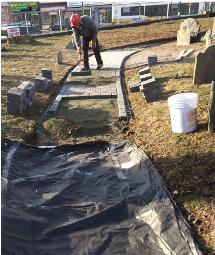
A workman installing the new concrete pavers in the pathway.
