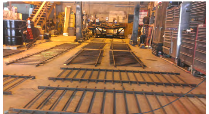
Individual fence panels are laid out in the contractor's shop for inspection before proceeding to sandblasting for paint removal.
