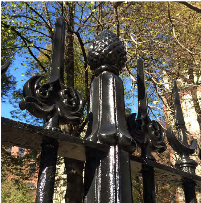
A detail of the fence after restoration.
