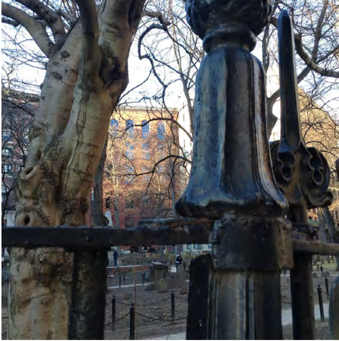
A detail of the fence before restoration.
