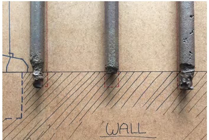
Some pickets were long enough to be reset into the wall and some needed to be lengthened.
