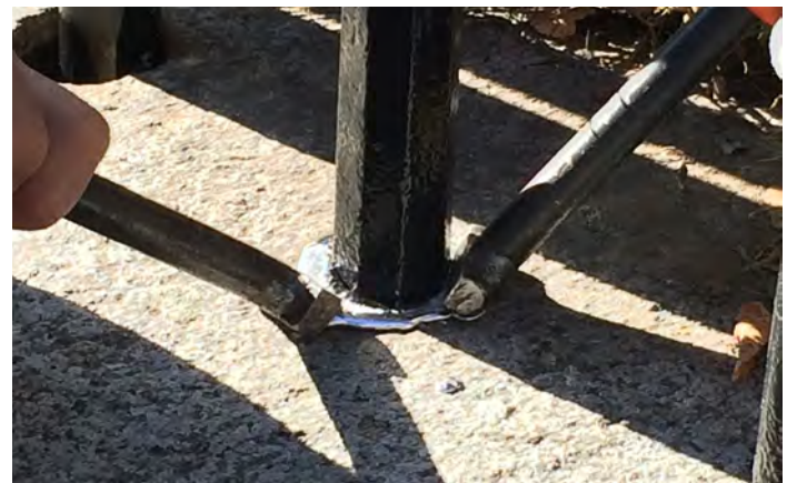
Next the molten lead is tamped down with special tools.
