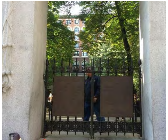
A workman reinstalls the gate at the Granary after restoration work.
