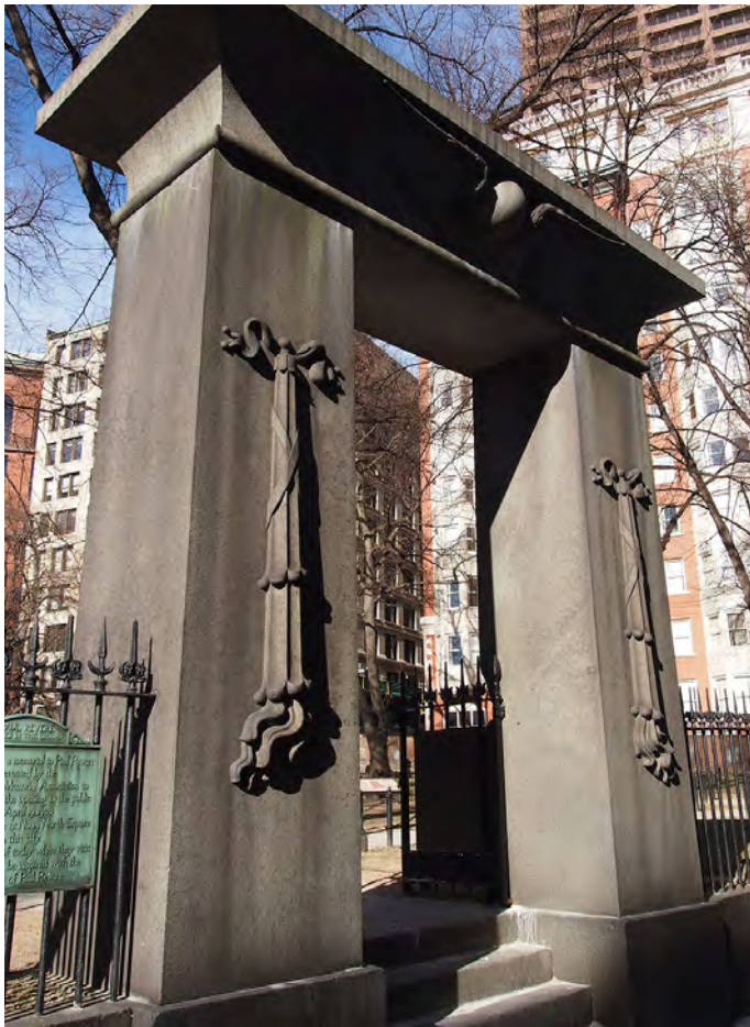
Granary entrance gate before cleaning.
