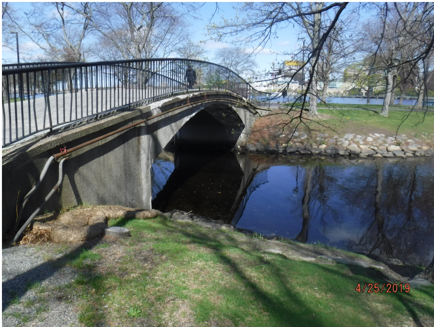
Photograph 4: View of bridge where proposed conduit will be located (typical).
