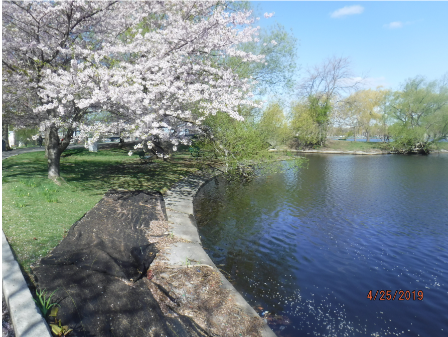
Photograph 5: View of Inland Bank along inner lagoon (typical).
