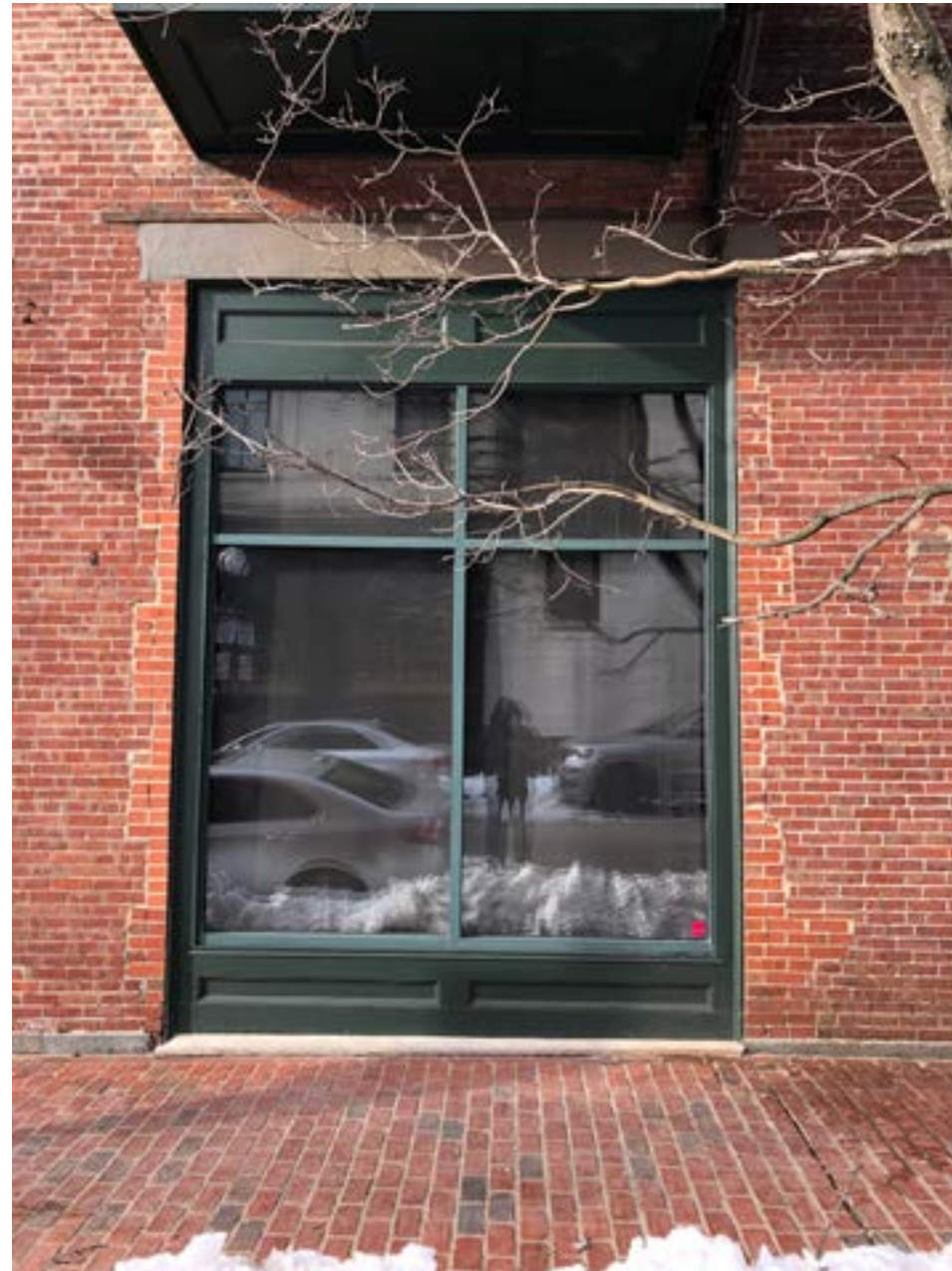
● Street elevation view looking at existing window
