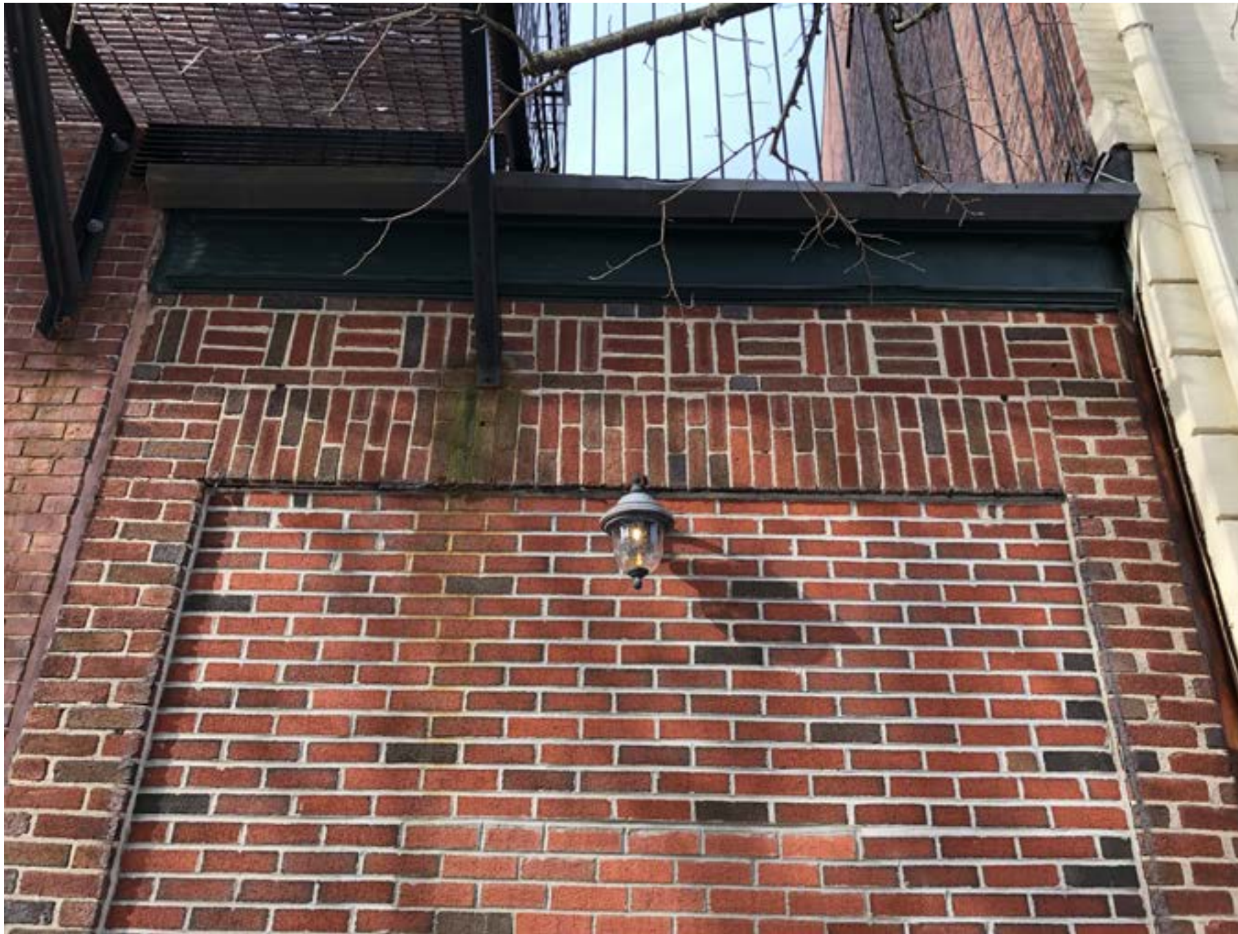
● Detail view of header on new window location
