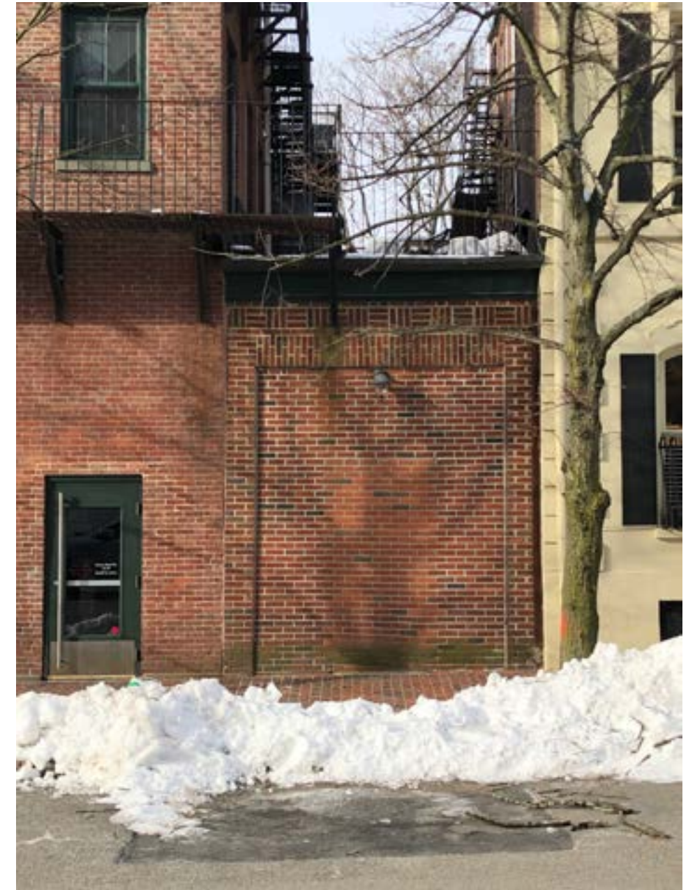
● Street elevation view looking at the new window location
