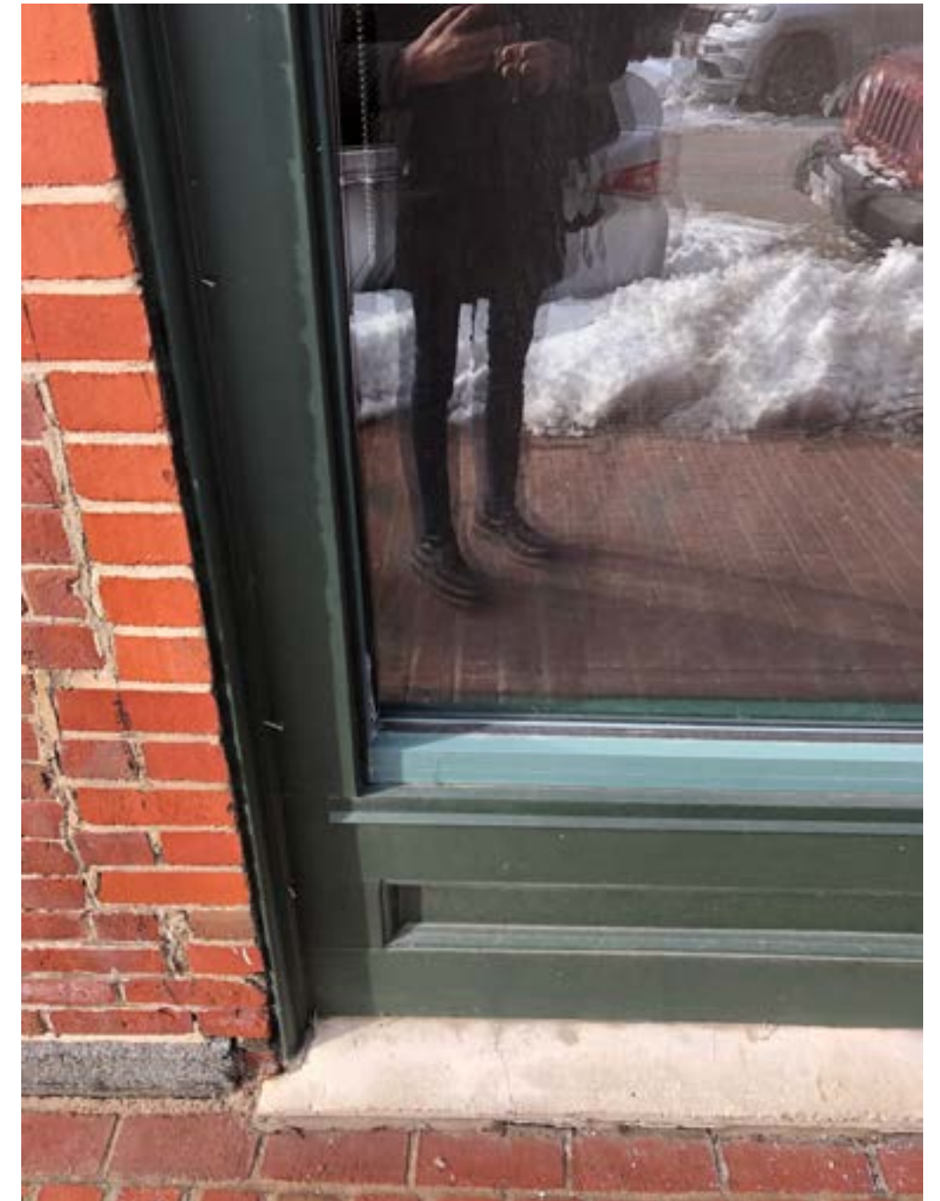
● Detail view of existing window woodwork and mullian
