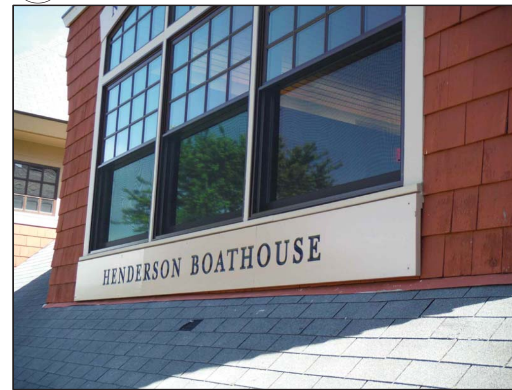
SIGN AT FLASHING ON SOUTH ELEVATION
