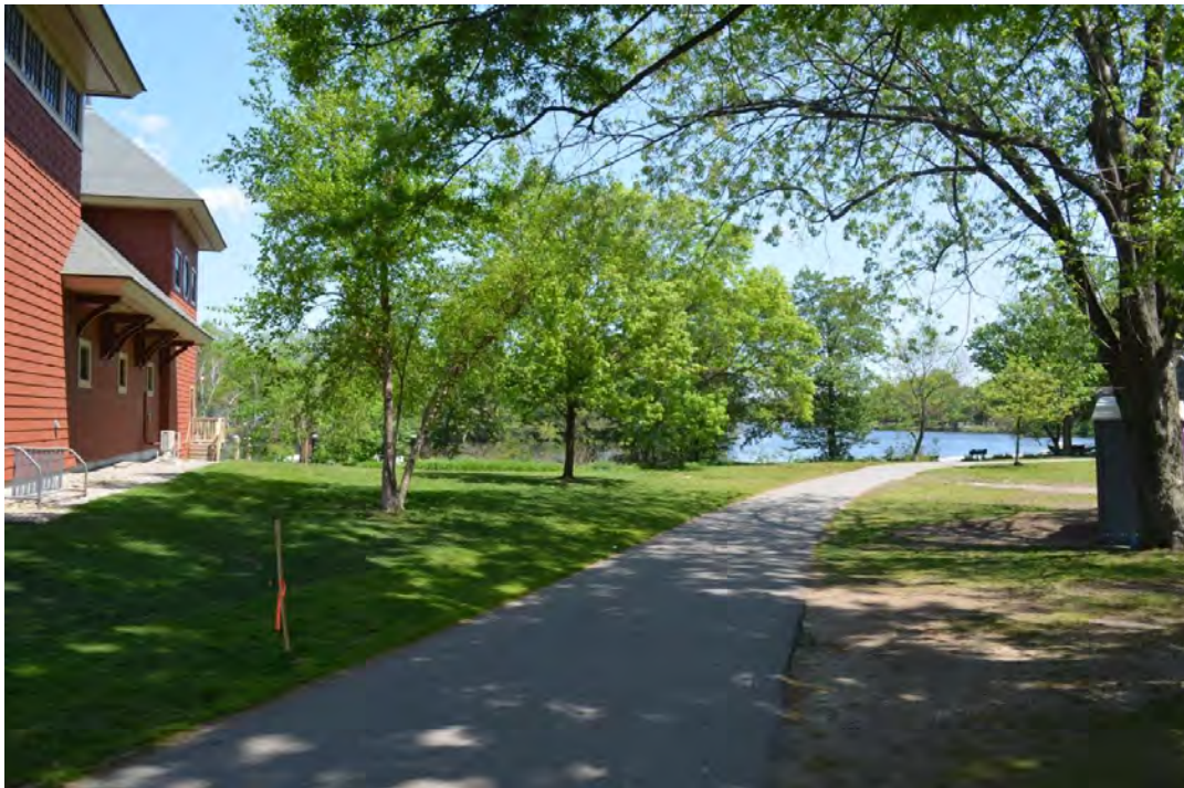
Photo 5: East side of Boathouse and Bike Path
