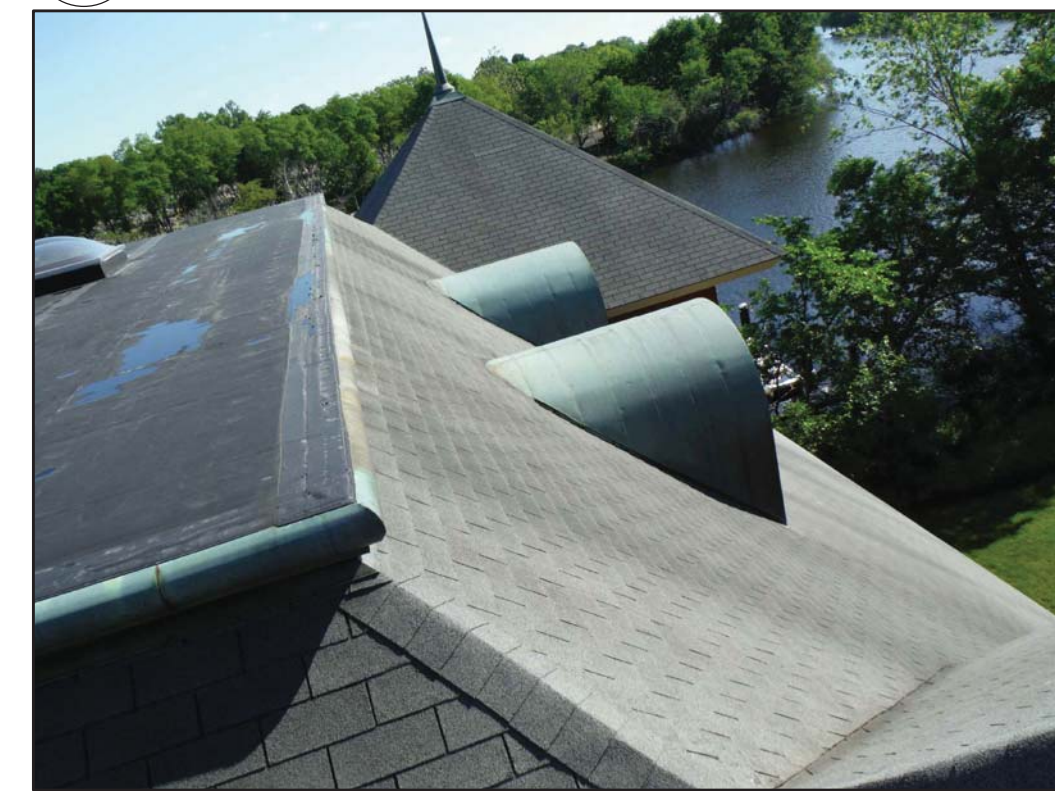
VIEW OF DORMERS OF EAST ROOF WITH COPPER CLADDING
