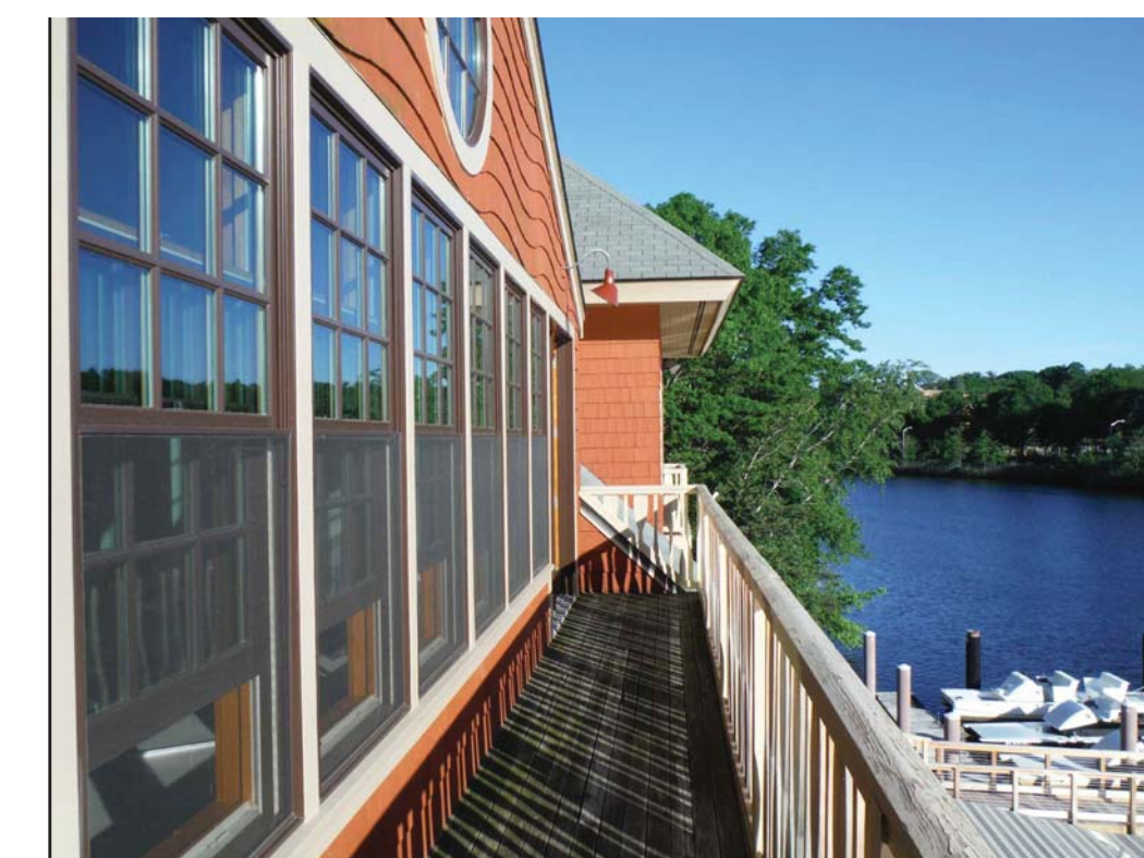
VIEW OF EXISTING WOOD DECK
