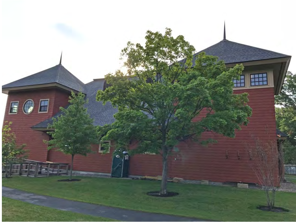
Photo 3: West side of the Boathouse
