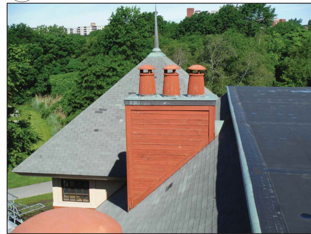
VIEW OF WEST CHIMNEY WITH WOOD CLADDING
