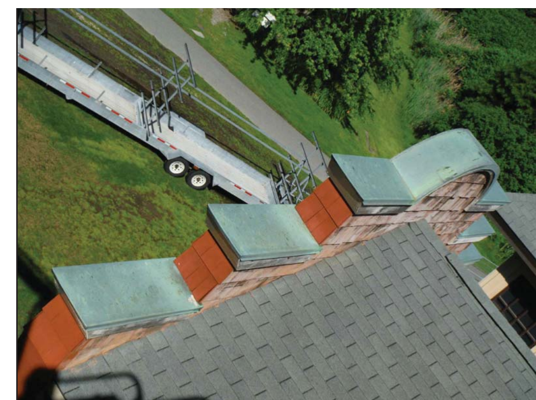
VIEW OF BACK SIDE OF SOUTH FACADE AND ASPHALT ROOF
