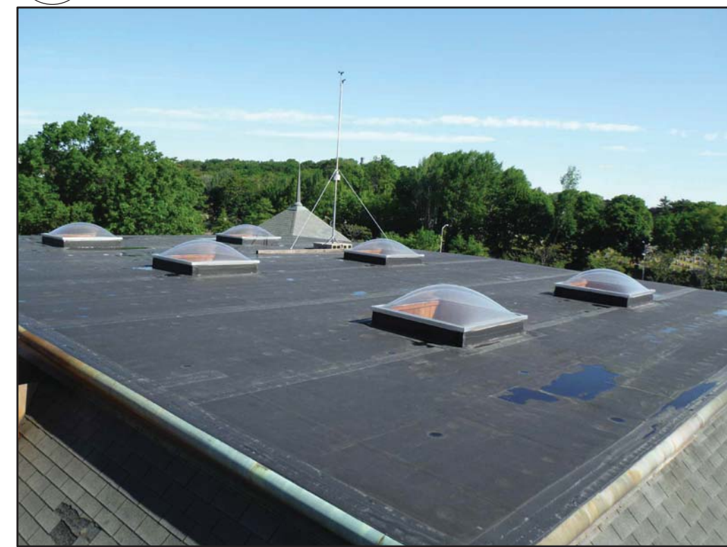
VIEW OF EXISTING EPDM FLAT ROOF
