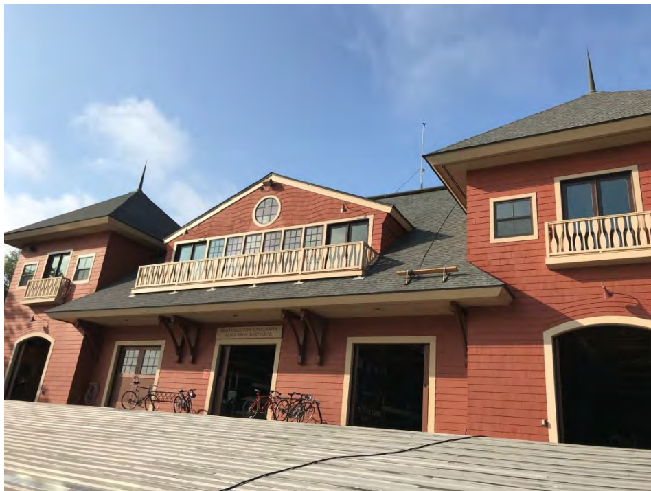
Photo 4: River side of the Boathouse
