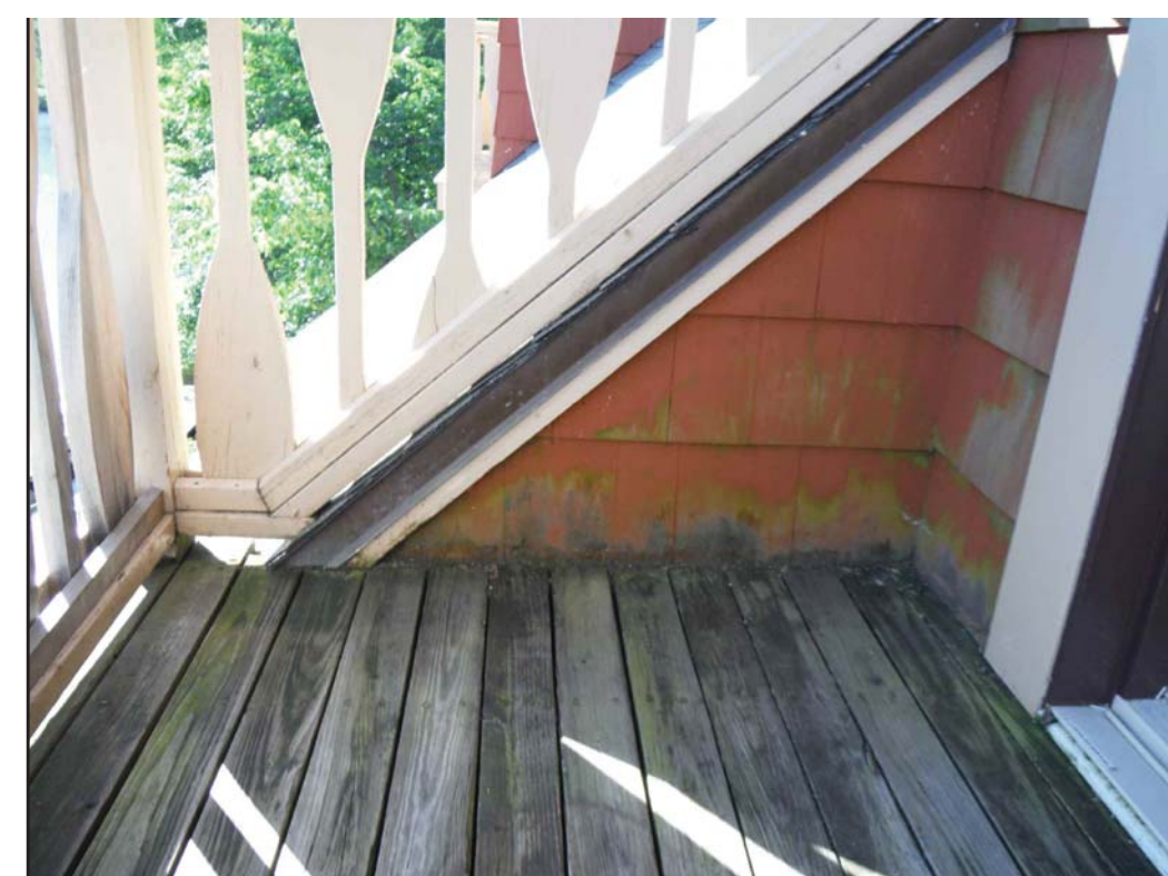
VIEW OF ROOF EDGE AT WOOD DECK ON NORTH ELEVATION
