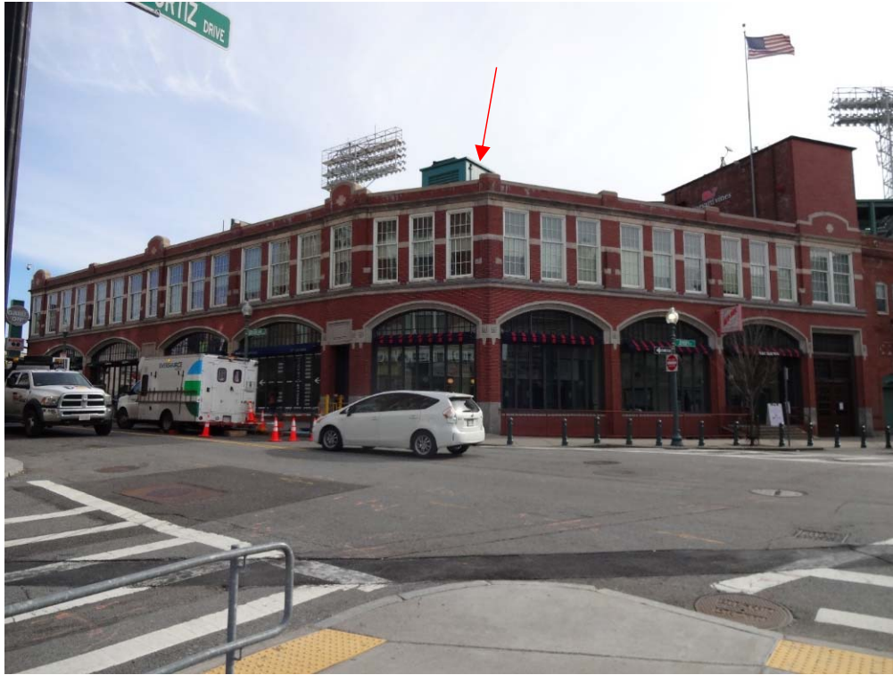
Photo 5: Proposed antenna location on Penthouse.
