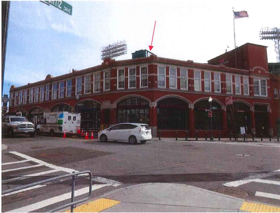
Photo 5: Proposed antenna location on Penthouse.
