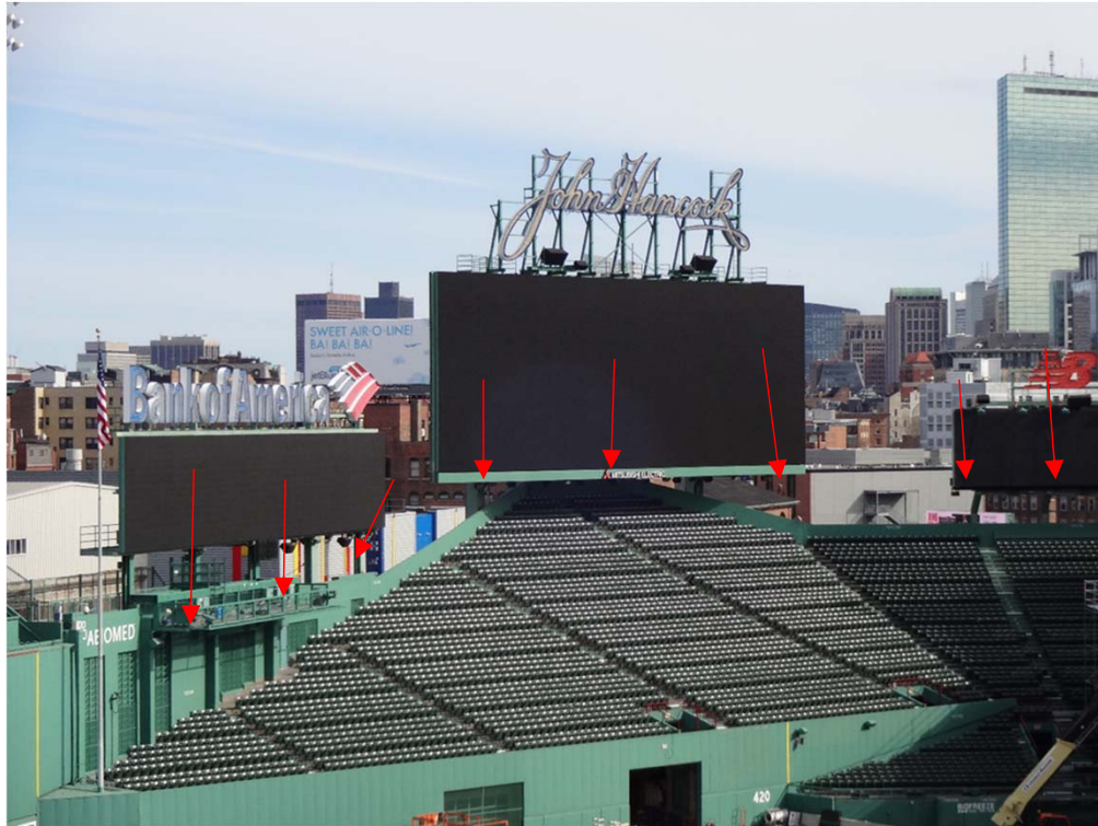
Photo 9: Proposed antenna locations on scoreboards, in the outfield
