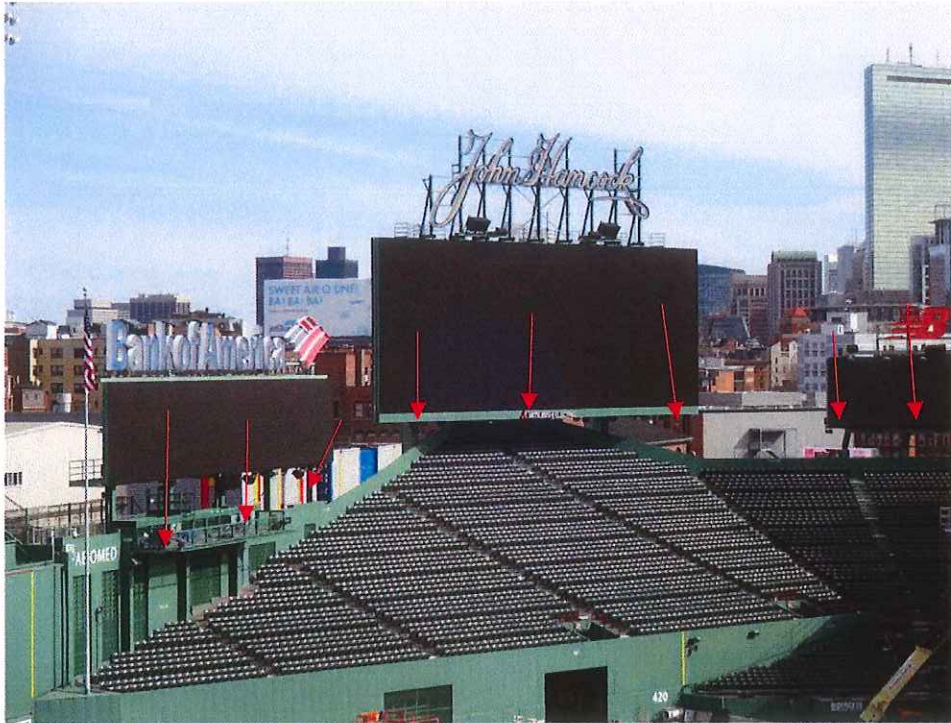
Photo 9: Proposed antenna locations on scoreboards, in the outfield
