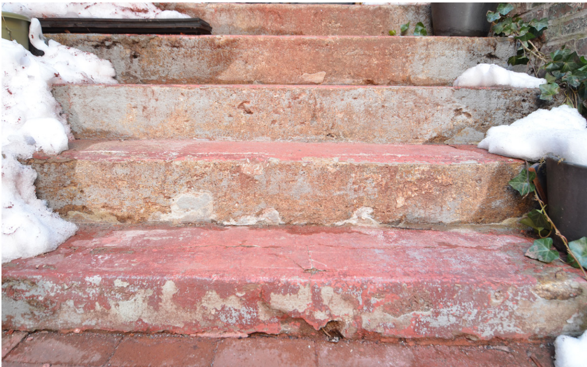
5. CONDITION OF STAIR
