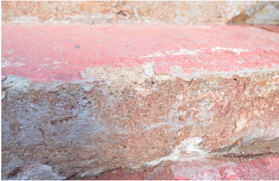
8. CONDITION OF STAIR
