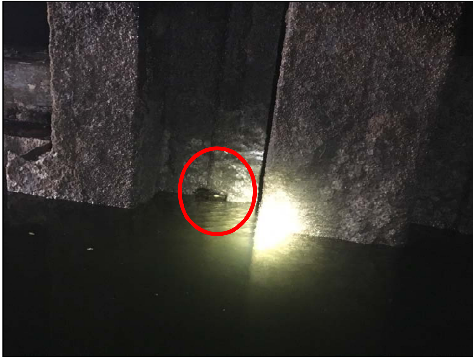
Photo No. 11: Location of a 5" diameter hole east of the culvert opening.
