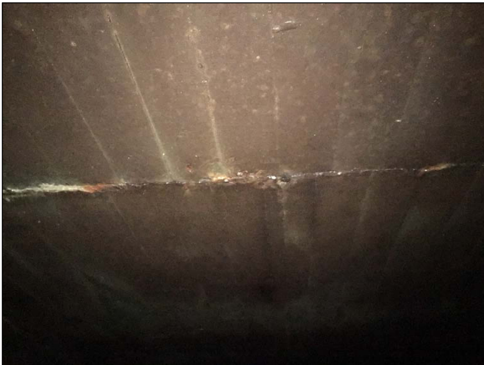
Photo No. 14: Overview of typical culvert ceiling joint.
