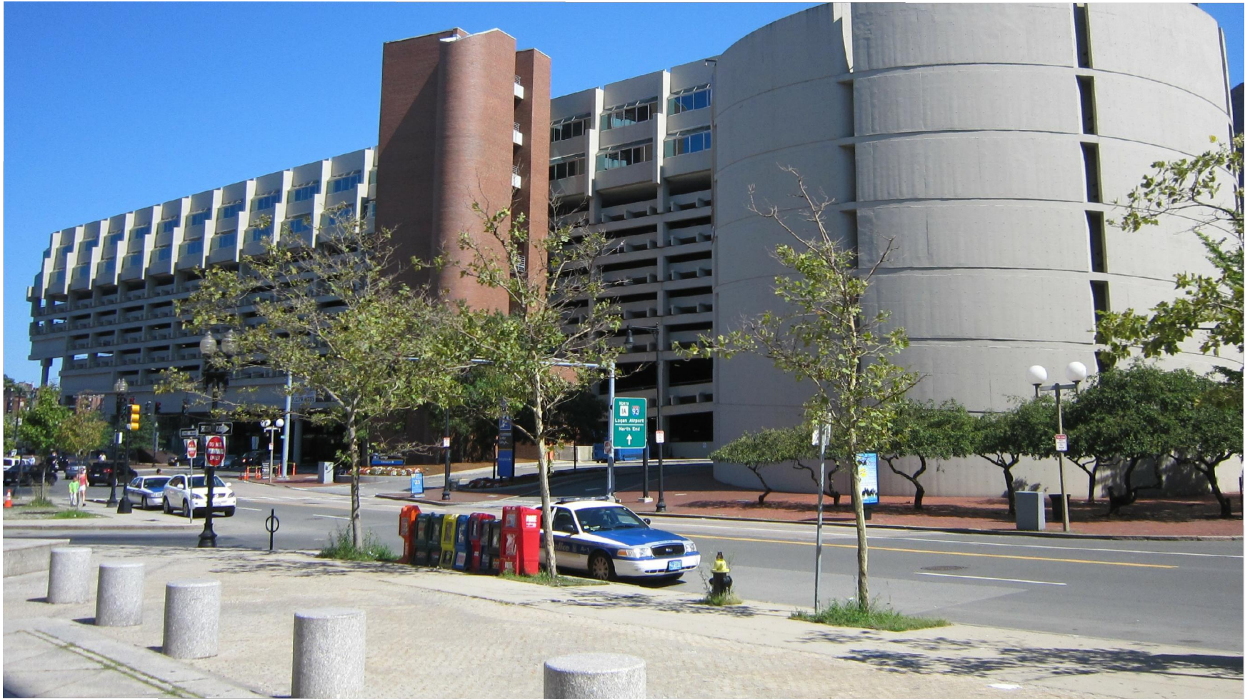
View of New Chardon Street and Existing Garage Looking South
