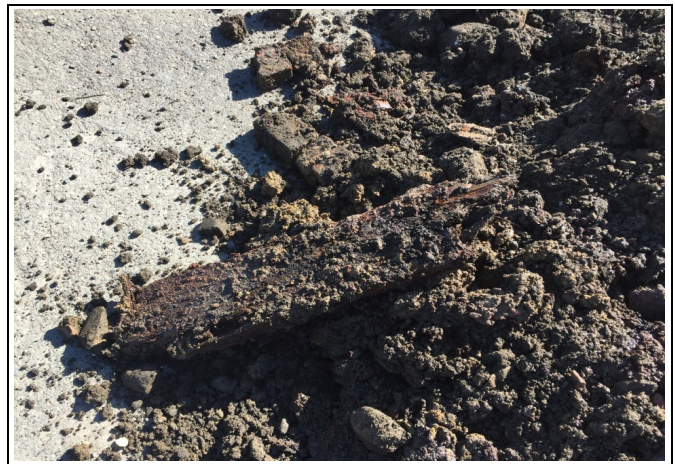
Photo 4 - Wood (dimensional lumber) removed from test pit.
