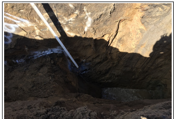
Photo 4 - West sidewall of test pit exposing concrete wall.
