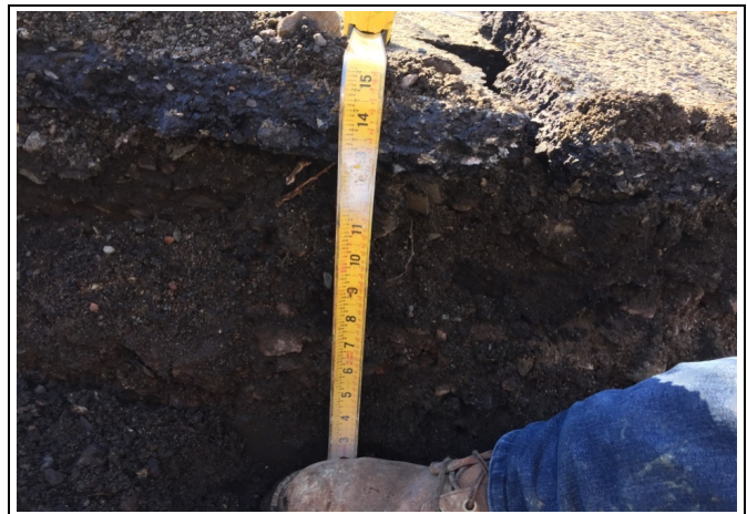
Photo 4 - Cobblestone pavement approximately 14 inches below ground surface.
