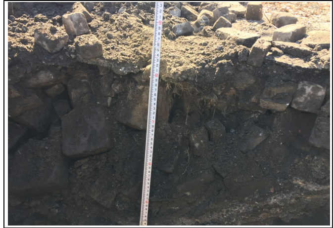
Photo 2 - Granite blocks and cobblestones beneath pavement.
