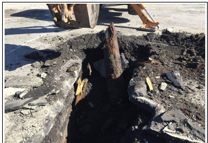
Photo 4 - Dimensional lumber removed from test pit at depth of approximately 4 ft.
