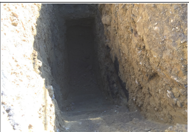
Photo 5 - Bottom of test pit.
