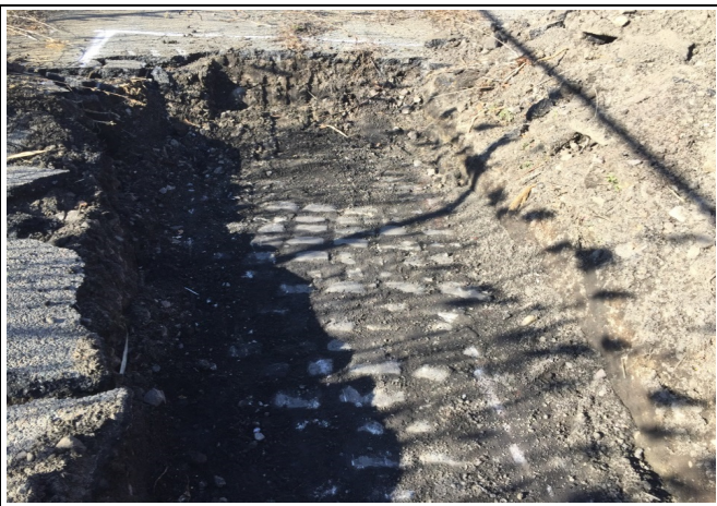
Photo 3 - Bored cobblestone pavement.
