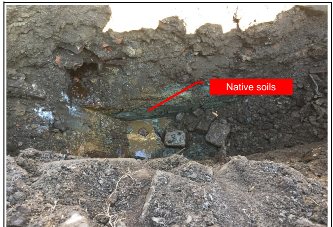
Photo 6 - North sidewall of test pit.
