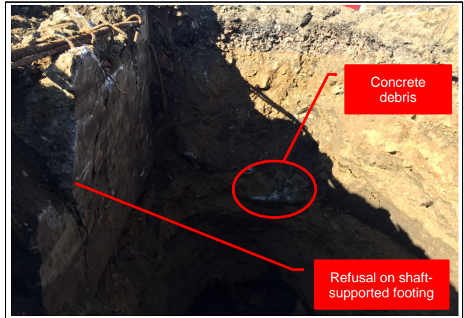
Photo 2 - Upper half of test pit looking west.
