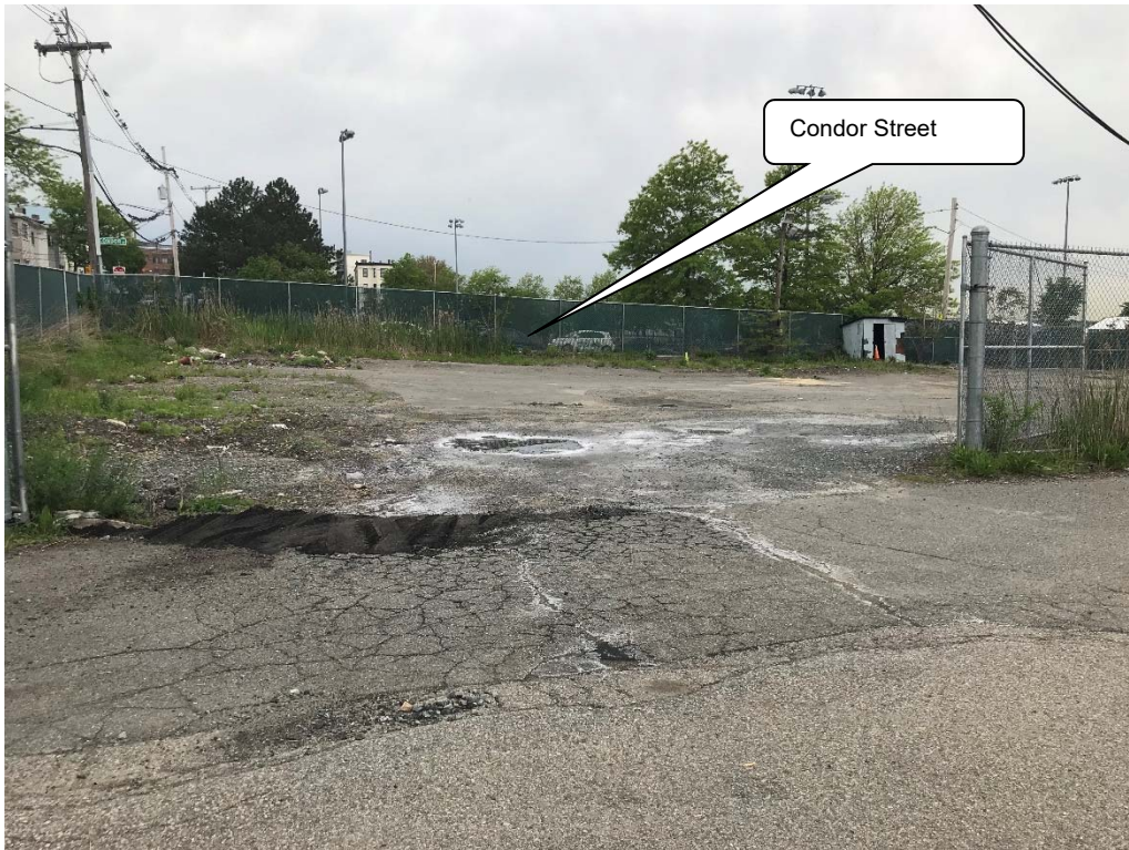
Photo 11 – Looking west at the southwest corner of the parcel
