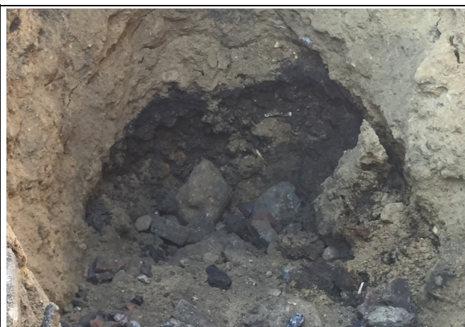
Photo 5 - Close up of debris layer encountered below a depth of 8 ft.
