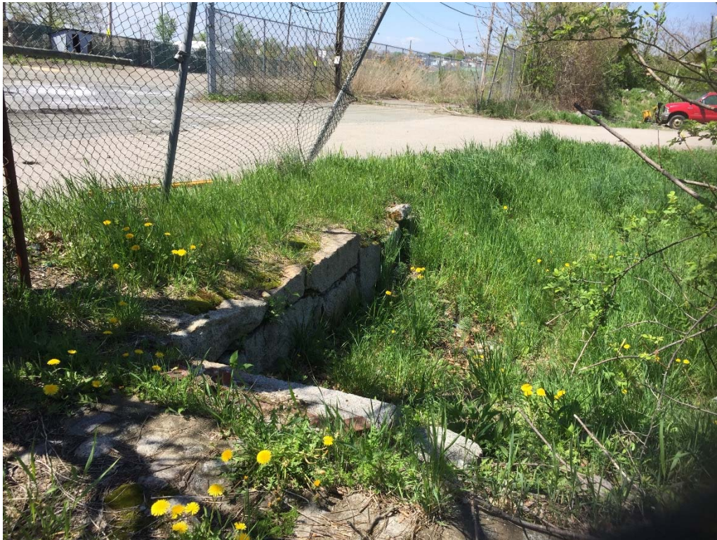
Photo 13 – Existing retaining wall adjacent to East Eagle Street
