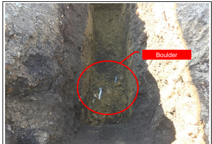
Photo 4 - Excavation refusal on boulder at least 7 feet in diameter.
