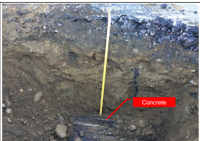
Photo 5 - North sidewall of test pit.
