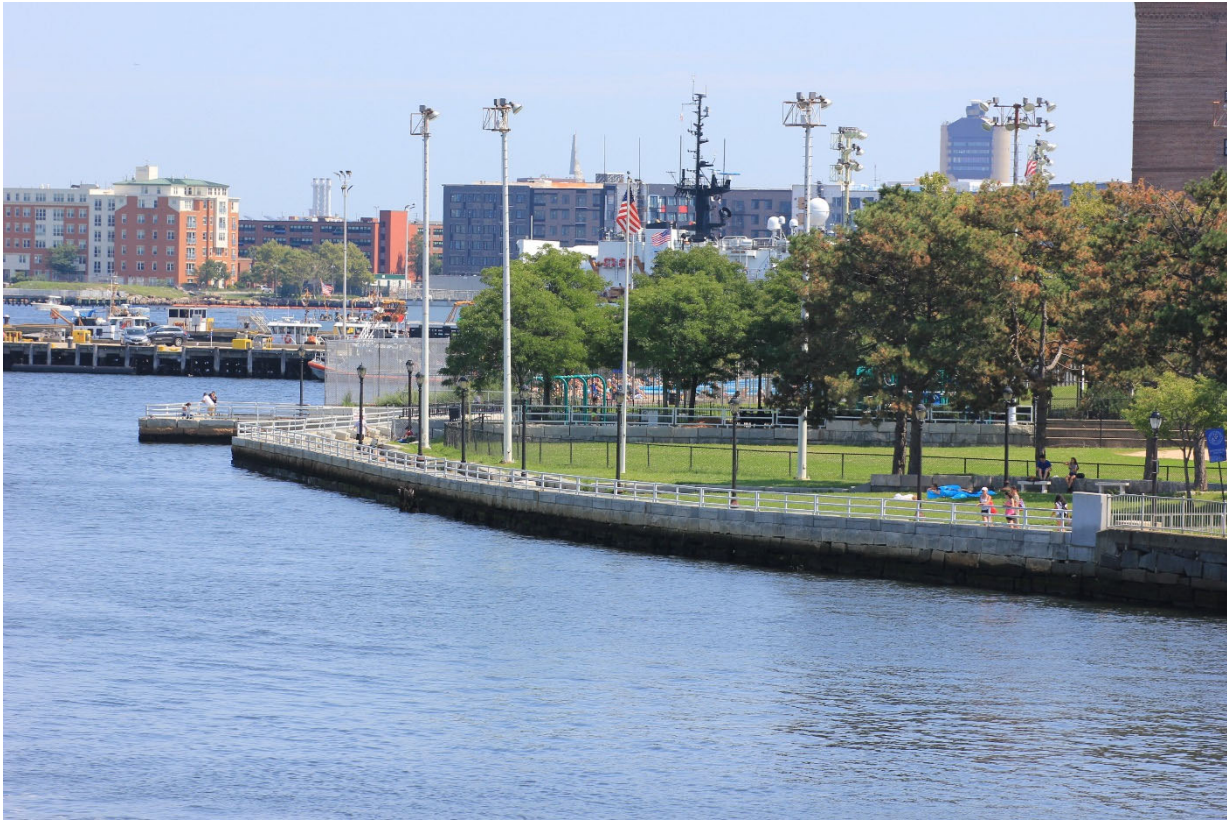
6. Seawalls from North Washington Bridge
