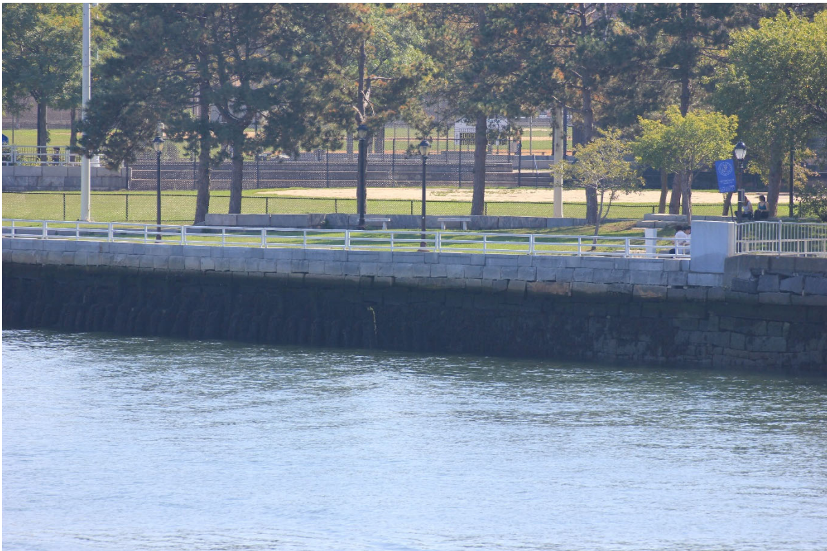
7. Seawall at Low Tide
