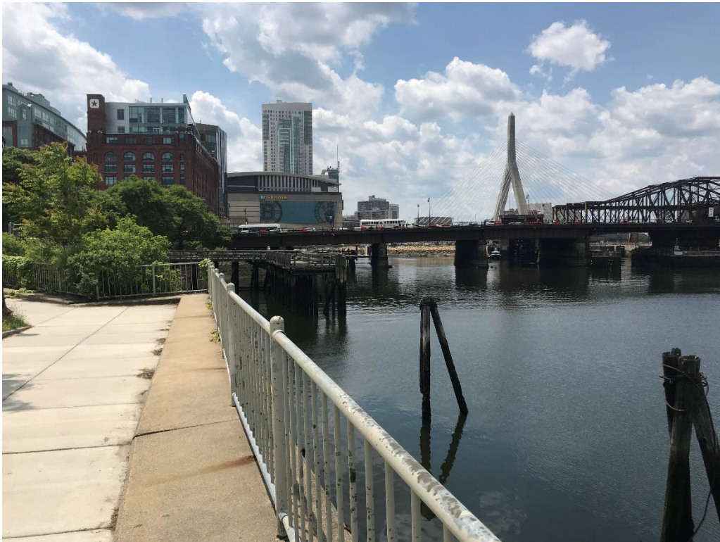
4. Top of sea wall, overlooking Boston Harbor.
