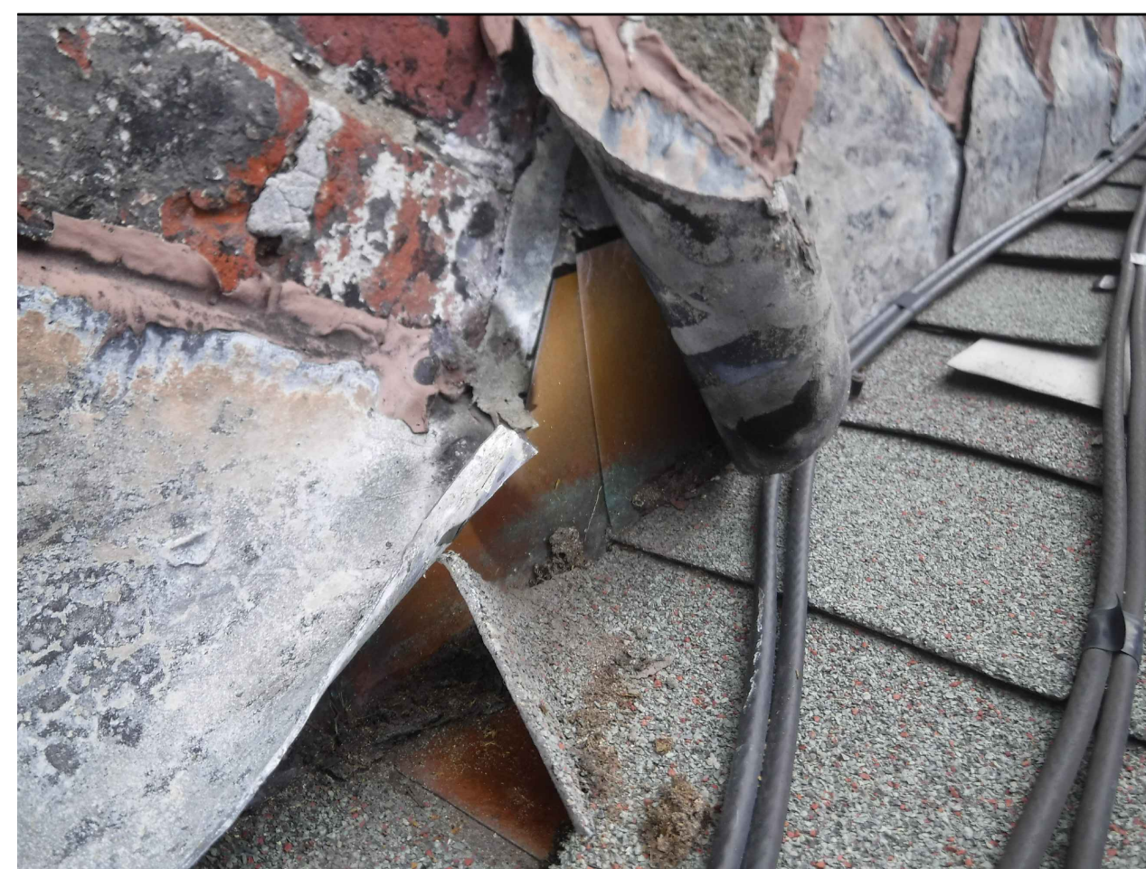
7 EXISTING AT STEP FLASHING CONDITION AT ASPHALT ROOFING
