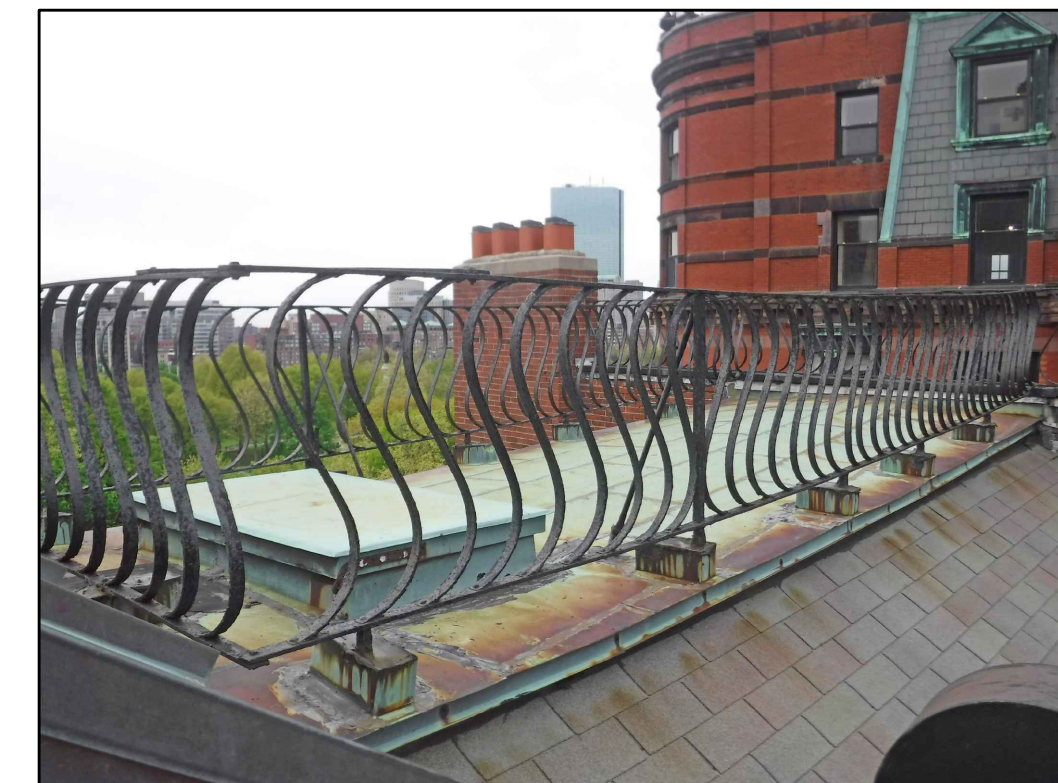
FLAT PORTION OF ROOF
