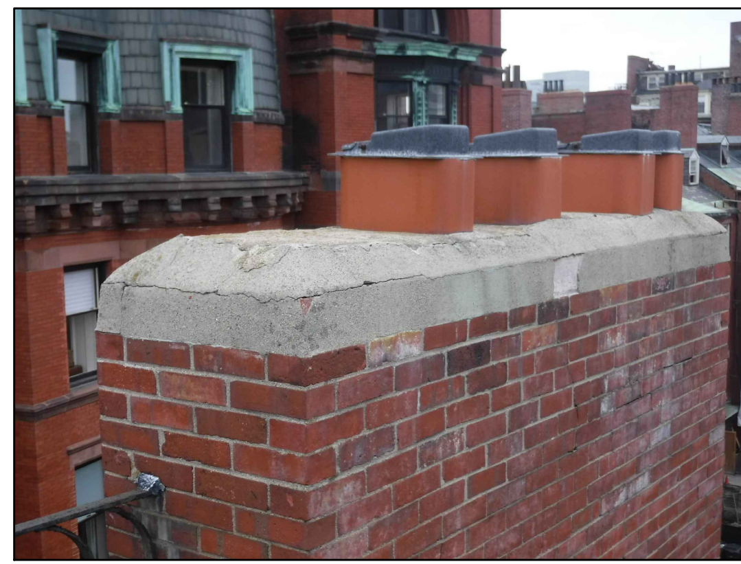
NORTH EAST CHIMNEY CAP 13 EXISTING CONDITIONS - PHOTO 13 SCALE: NOT TO SCALE
