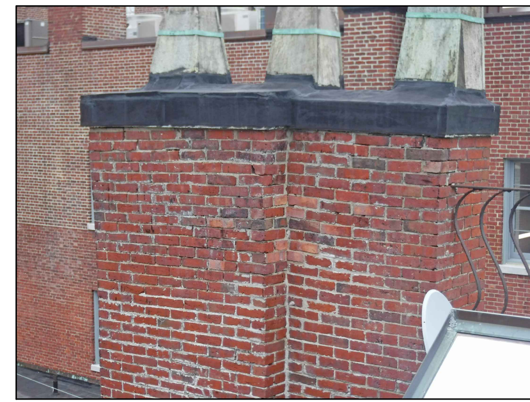
NORTH EAST CHIMNEY 15 EXISTING CONDITIONS - PHOTO 15 SCALE: NOT TO SCALE
