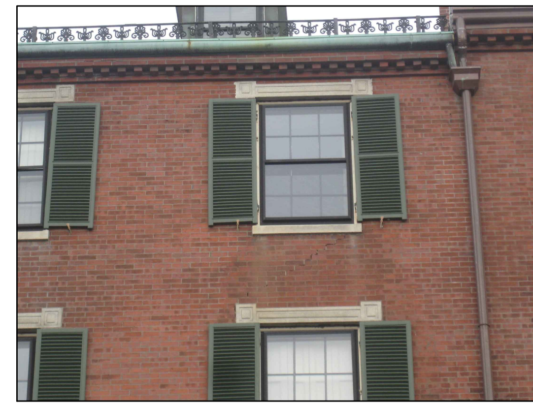
SOUTH ELEVATION WINDOW 17 EXISTING CONDITIONS - PHOTO 17 SCALE: NOT TO SCALE
