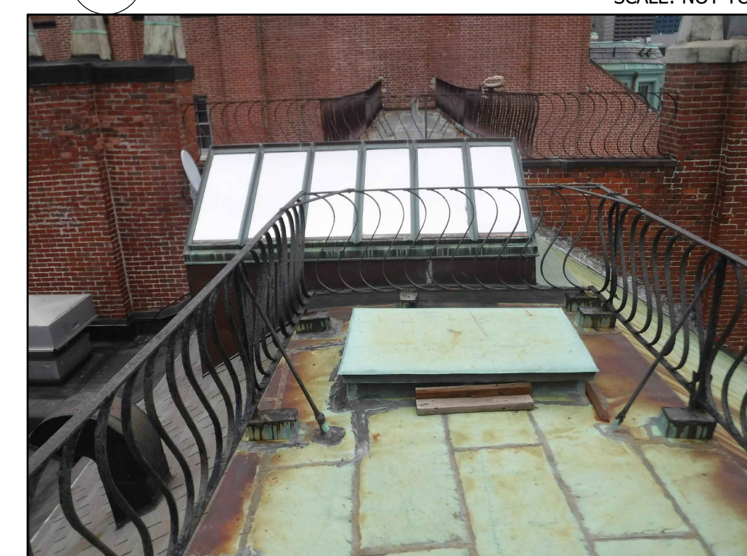
PORTION OF FLAT ROOF
