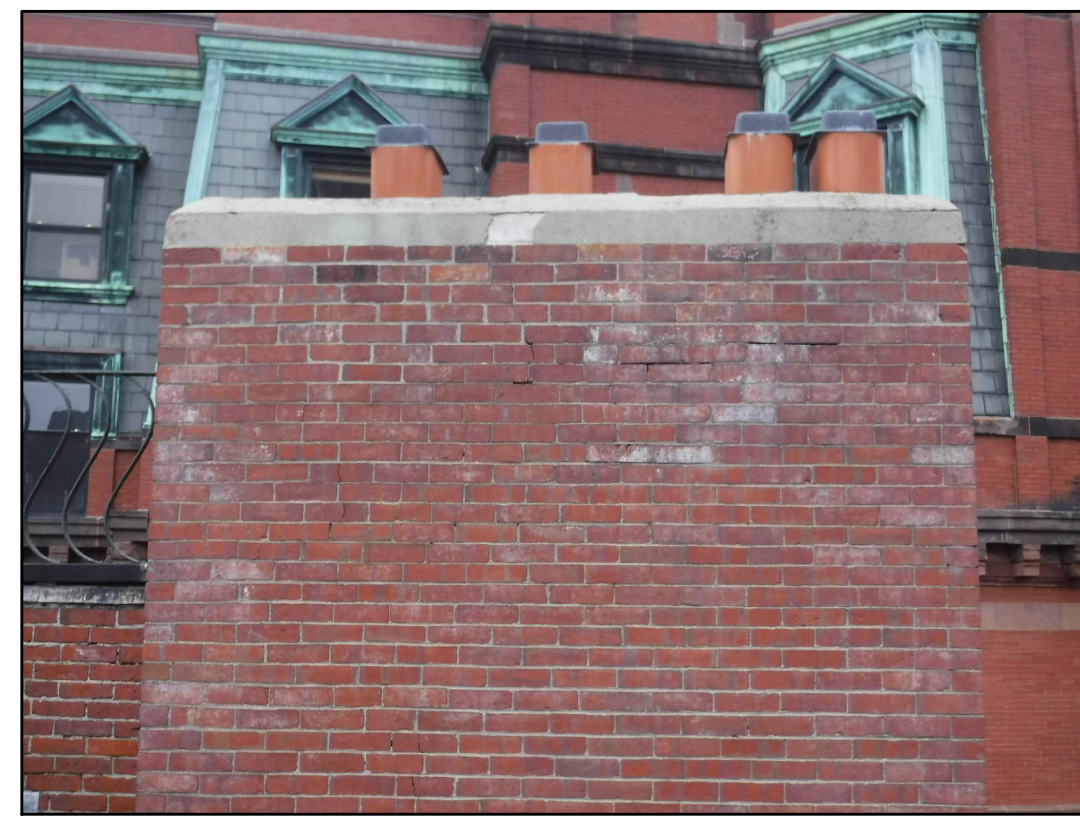
NORTH WEST CHIMNEY 8 EXISTING CONDITIONS - PHOTO 8 SCALE: NOT TO SCALE
