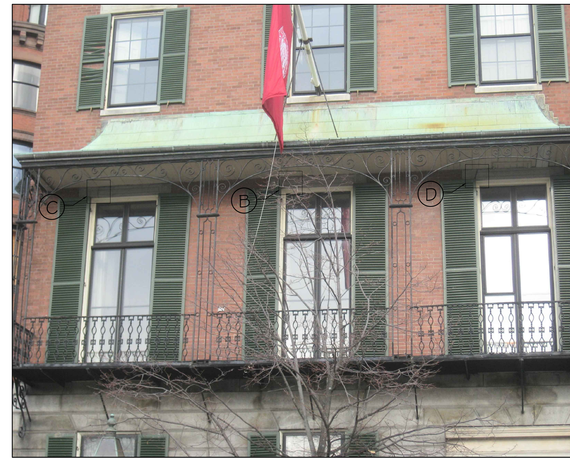
D EXISTING CONDITIONS - PHOTO 4 NOT TO SCALE
