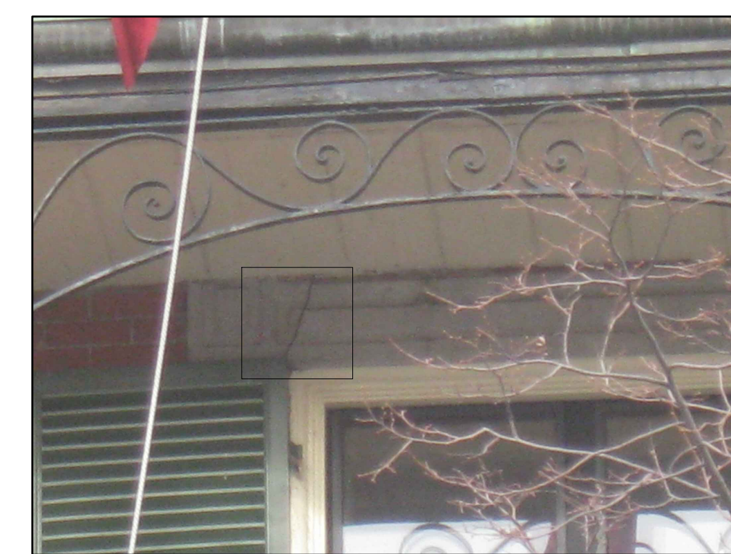
B EXISTING CONDITIONS - PHOTO 2 NOT TO SCALE
