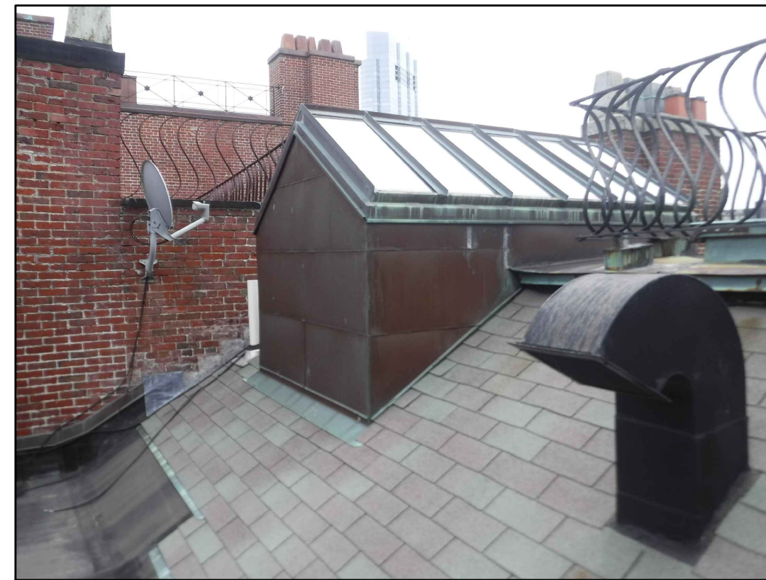
NORTH ROOF LOOKING EAST 26 EXISTING CONDITIONS - PHOTO 26 SCALE: NOT TO SCALE
