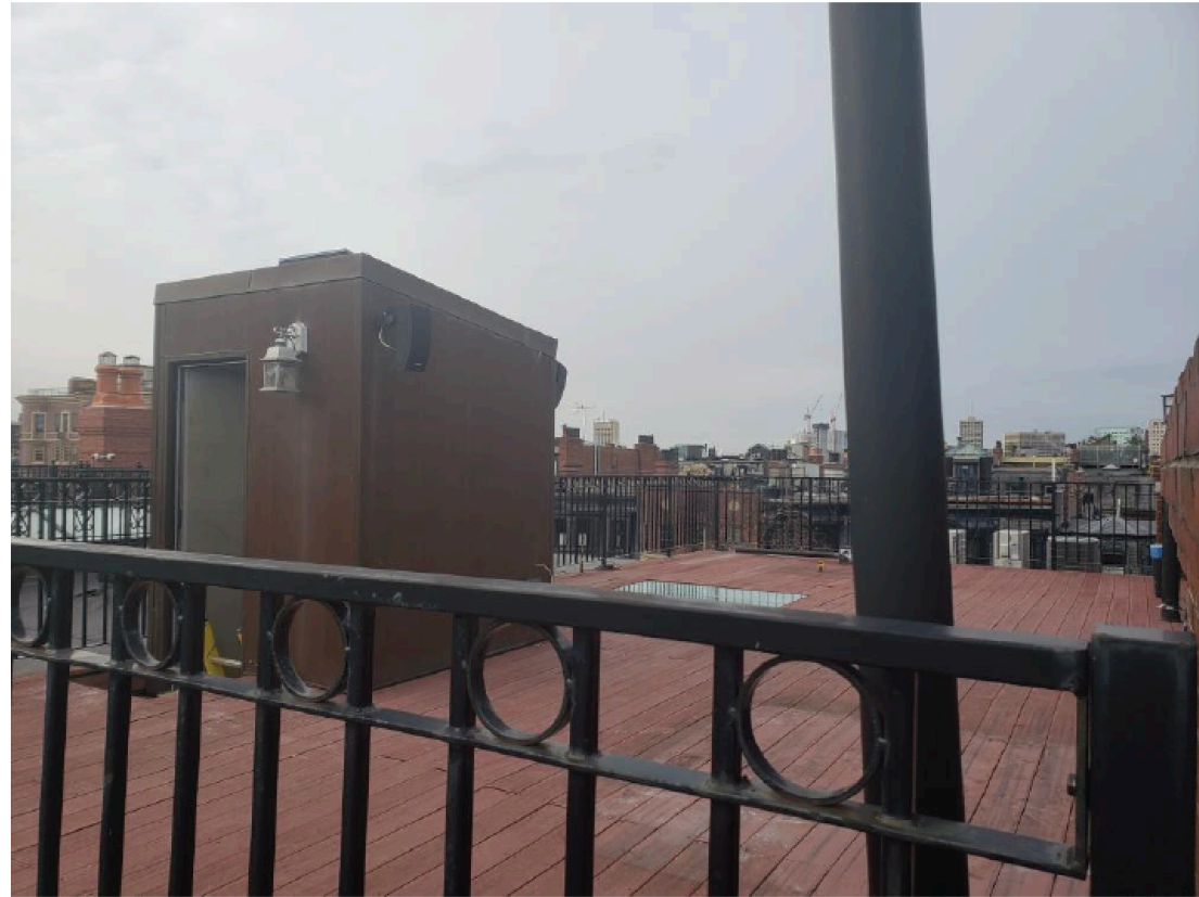
EXISTING ROOF DECK + HEADHOUSE
