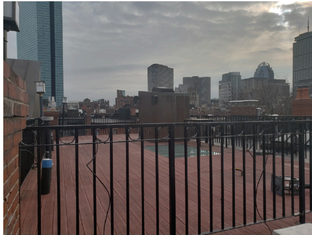
EXISTING ROOF DECK + HEADHOUSE
