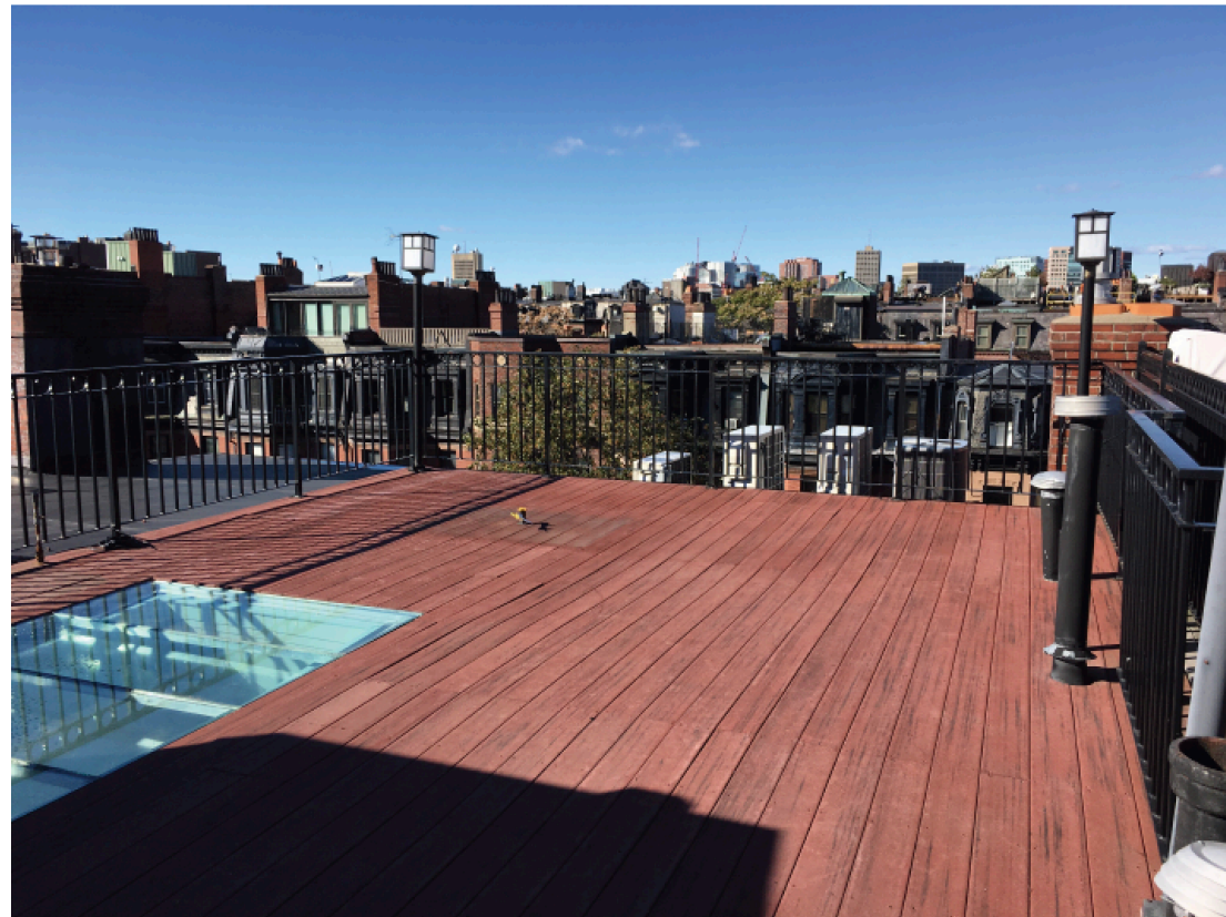
EXISTING ROOF DECK + SKYLIGHT
