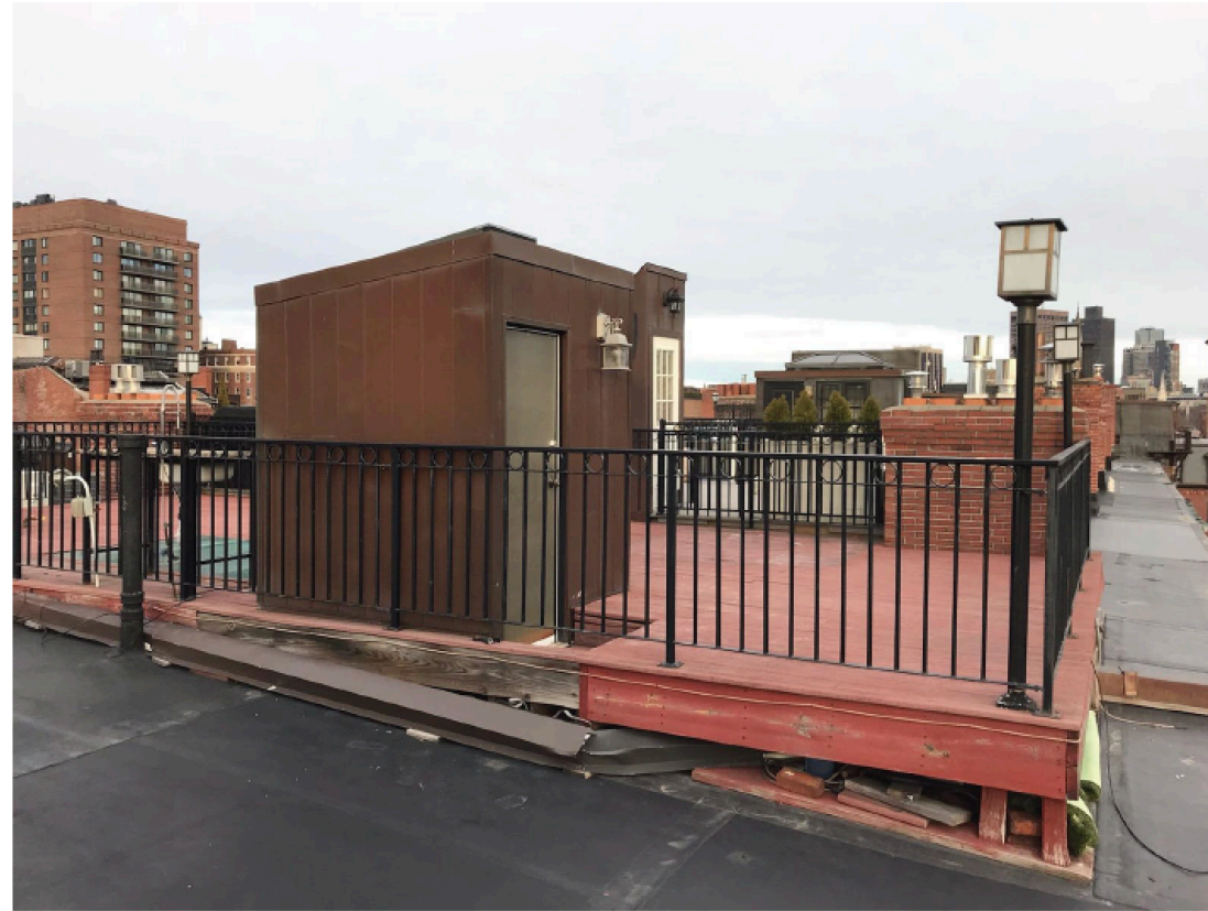
EXISTING ROOF DECK + HEADHOUSE
