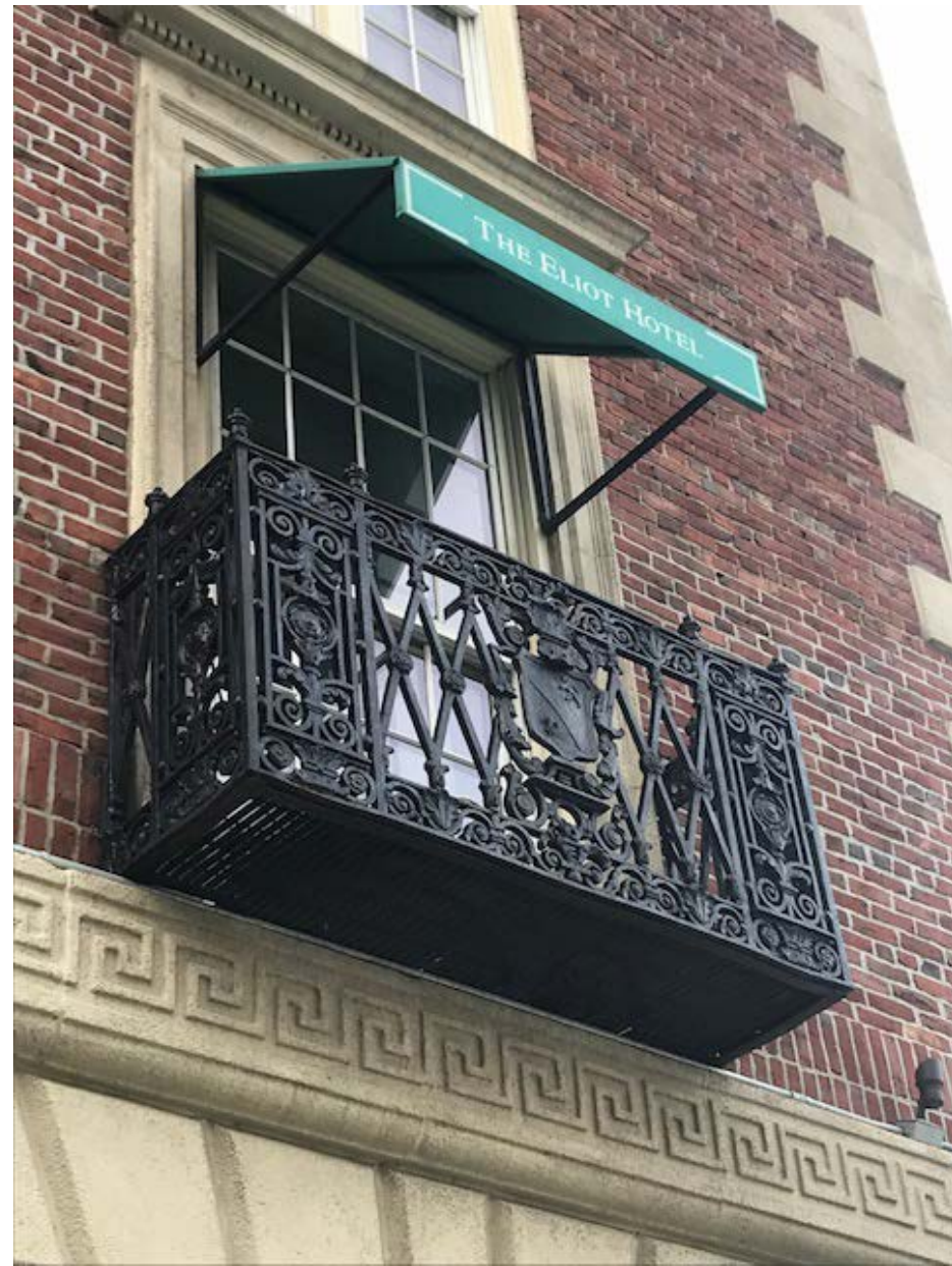
IMAGE AT EXISTING AWNINGS & FRAME - MASS AVE.
