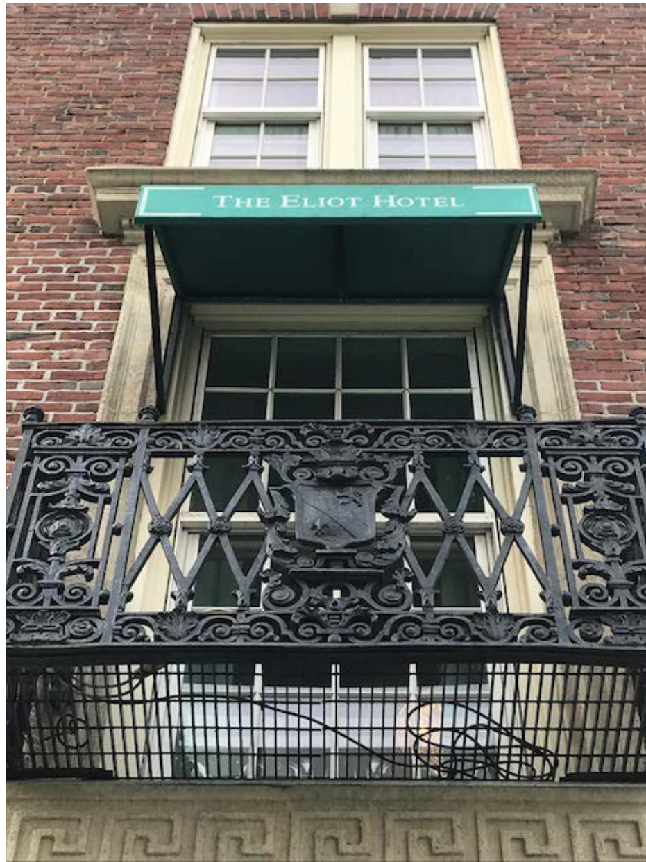
IMAGE AT EXISTING AWNINGS & FRAME - MASS AVE.
