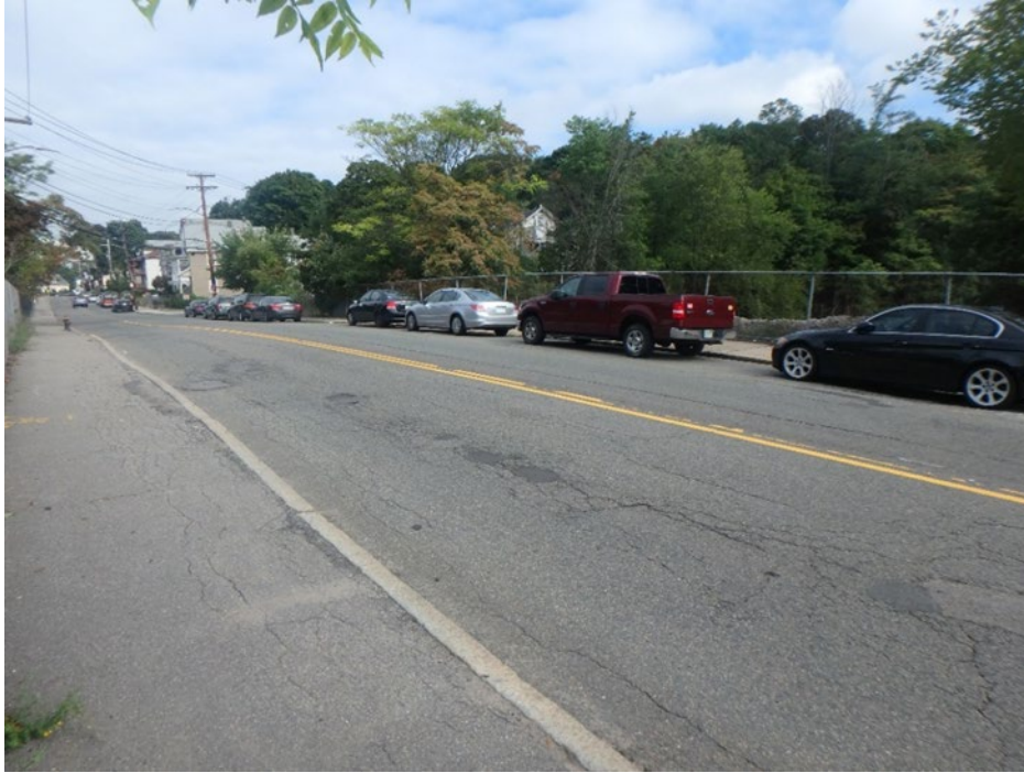
Photo 19: South approach looking at top of Dana Avenue Bridge along Dana Avenue, Hyde Park, Boston, MA.
