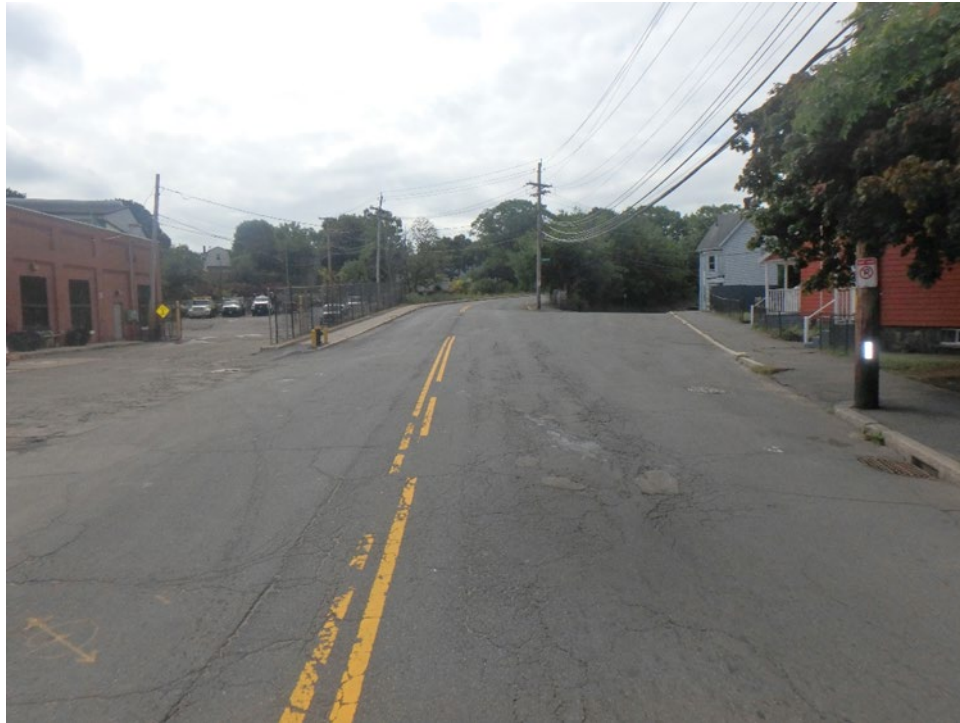
Photo 12: South approach looking south along Dana Avenue, Hyde Park, Boston, MA.
