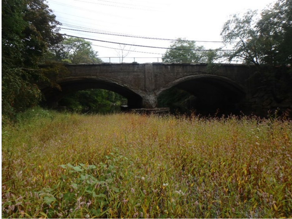
Photo 13: Upstream looking downstream along Neponset River, Hyde Park, Boston, MA.
