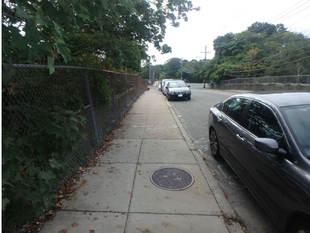
Photo 5: North approach looking at east sidewalk along Dana Avenue, Hyde Park, Boston, MA.
