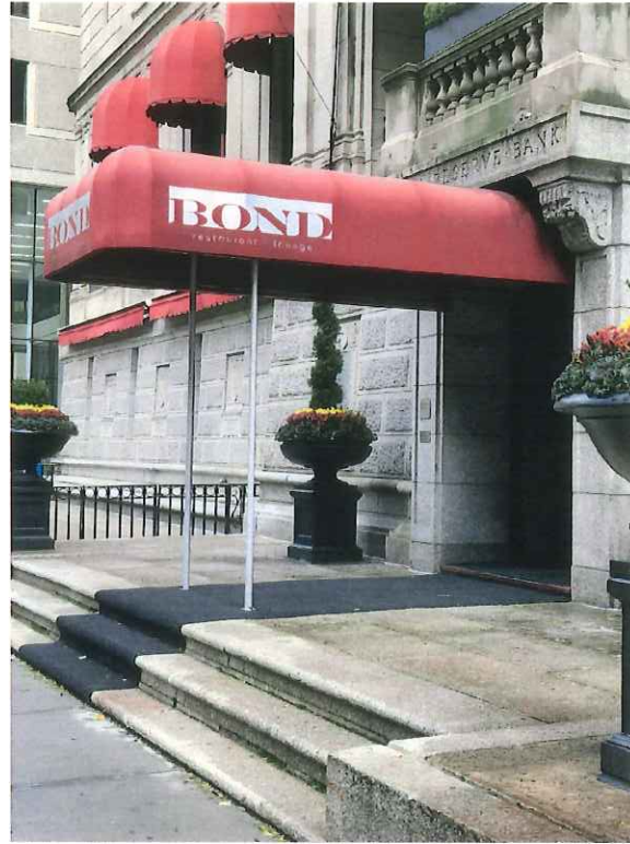
EXISTING PEARL STREET CANOPY
