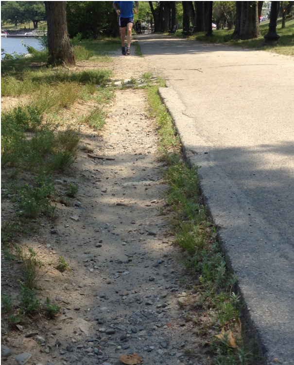
Runners compact the path edge. The proposed formalized runners' path will provide an un-paved path option while protecting the planted and natural areas.
