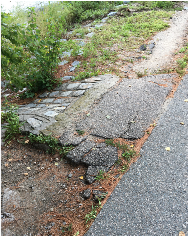
Compaction next to path edge makes cobblestone spillway ineffective. Grades will be adjusted to direct water to existing spillways, outfitted with sediment traps.
