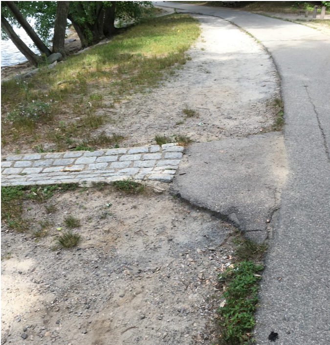
Example of the compaction typical along the perimeter pathway. The proposed formalized runners' path will provide an un-paved option for runners while protecting the planted and natural areas that are adjacent to the paths.
