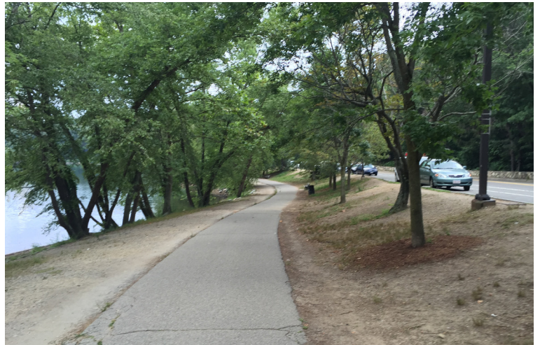
Perkins Street degraded slope and path edge will be decompacted and revegetated.
