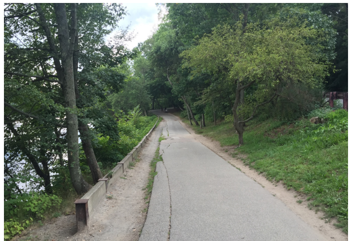
Timber wall and steep slopes along Francis Parkman Drive.
