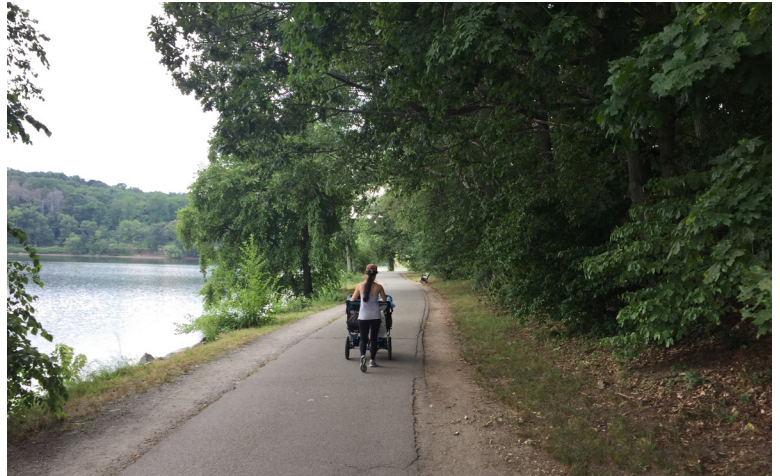
Where width permits, compacted trails currently form on both sides of paved path. A widened paved path, uphill swales, and the pondside runners' path will curb this damage.
