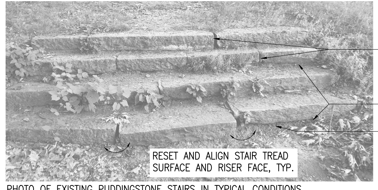
PHOTO OF EXISTING PUDDINGSTONE STAIRS IN TYPICAL CONDITIONS
