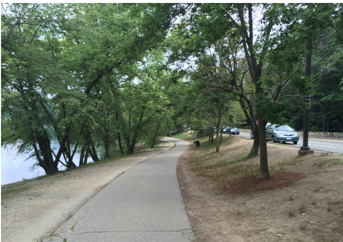
Paved path and degraded landscape along Perkins Street.
