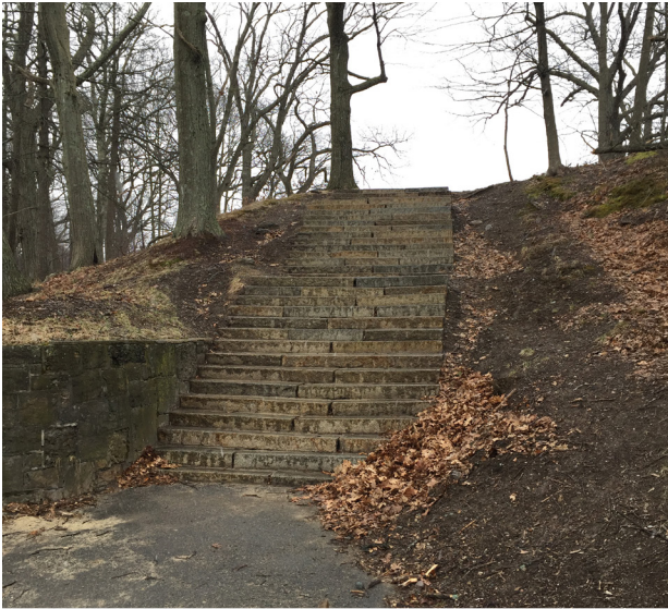
Side slopes of stairs will be planted with shrubs to hold slope and deter off-path walking.
