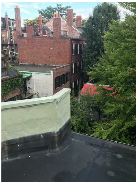
EXISTING COPPER CLADDING ON PARAPET
