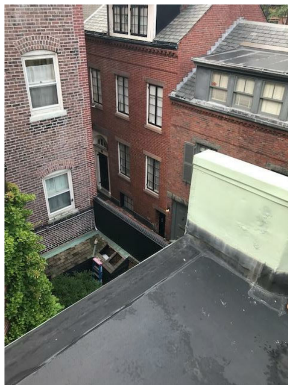
EXISTING COPPER CLADDING ON PARAPET
