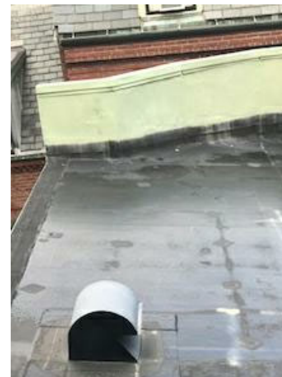
EXISTING COPPER CLADDING ON PARAPET
