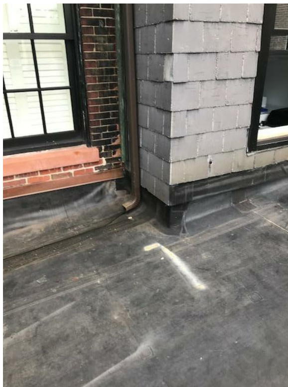
EXISTING FAUX SLATE AND RUBBER ROOF
