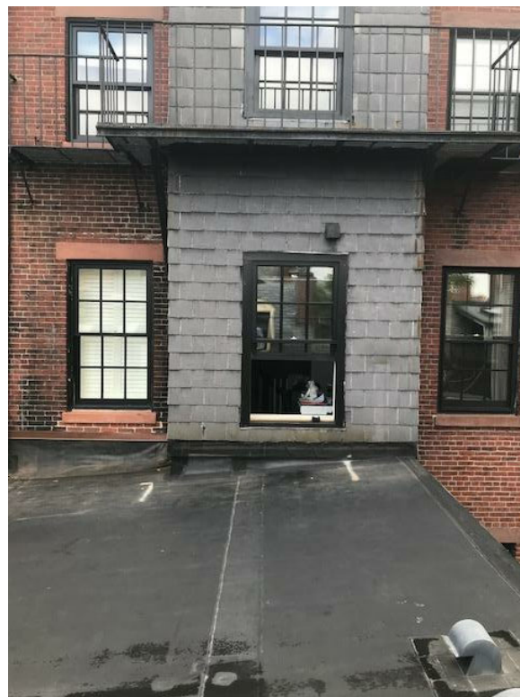
EXISTING FAUX SLATE AND RUBBER ROOF
