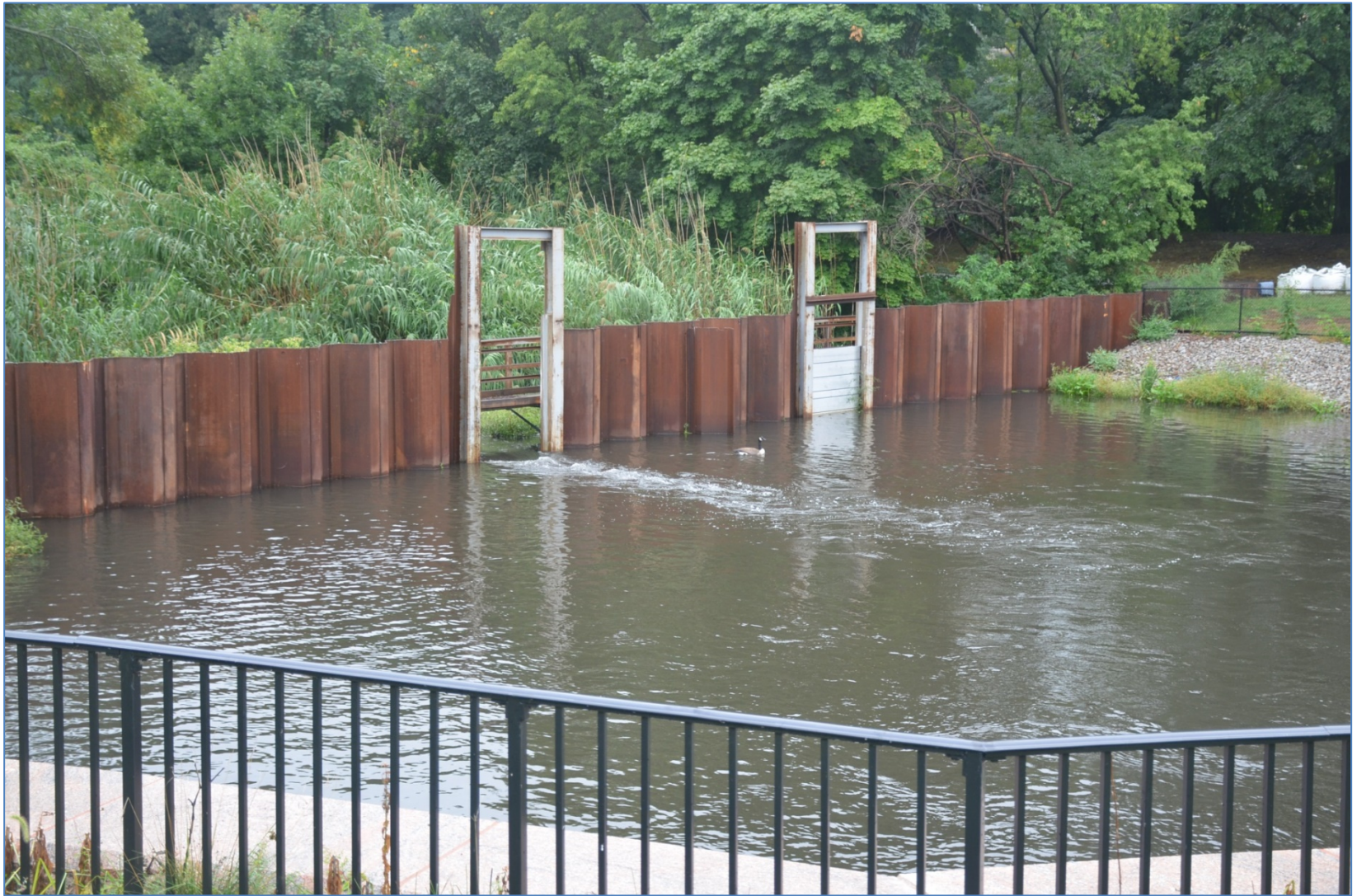
Photograph 2: FRCS near Park Drive.
