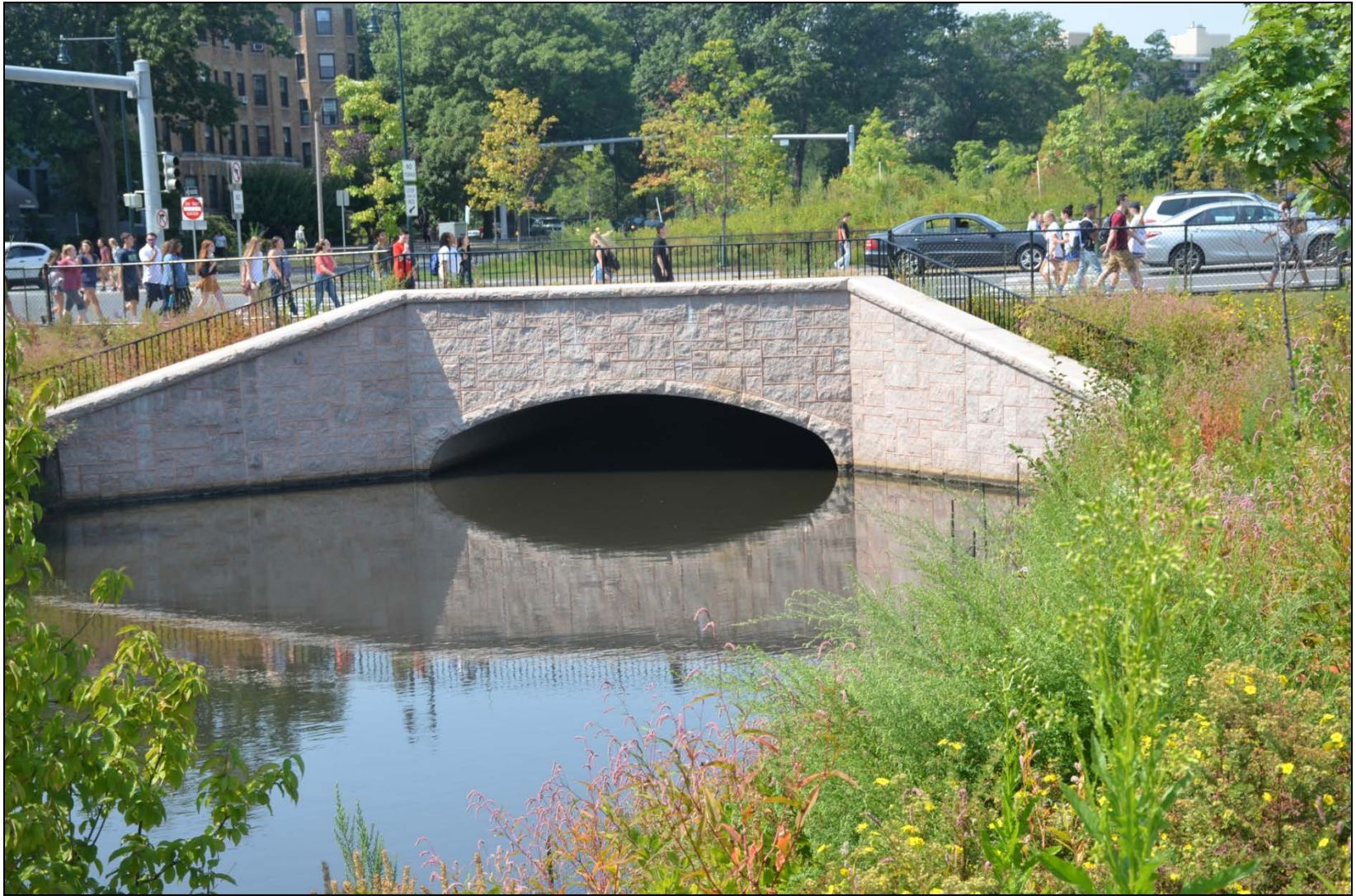
Photograph 21: Brookline Avenue culvert installed during Phase 1.
