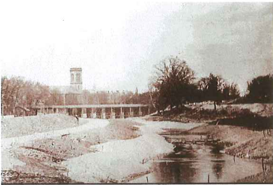
Muddy River Improvement in construction
