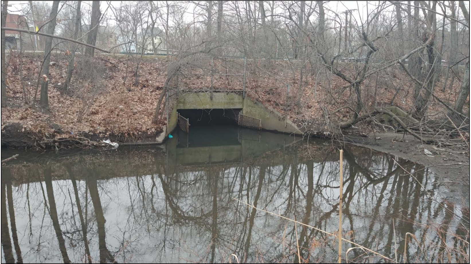
Photograph 6: Tannery Brook storm drain at Work Area 2.
