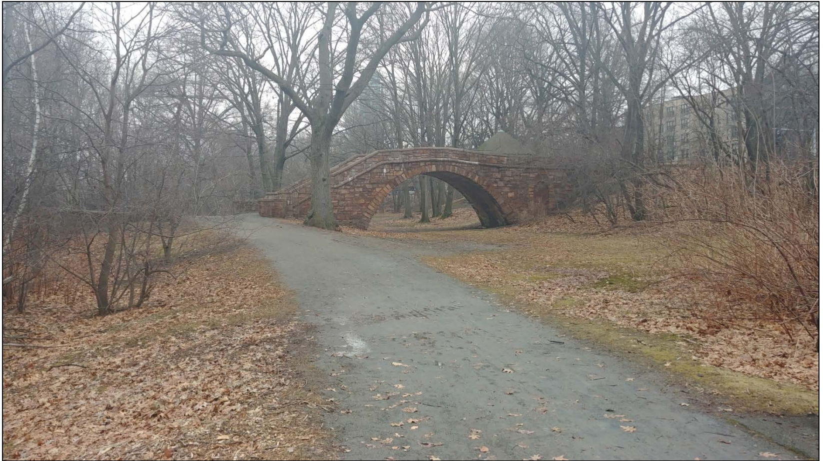
Photograph 4: Riverway walking path and footbridge near Work Area 5.
