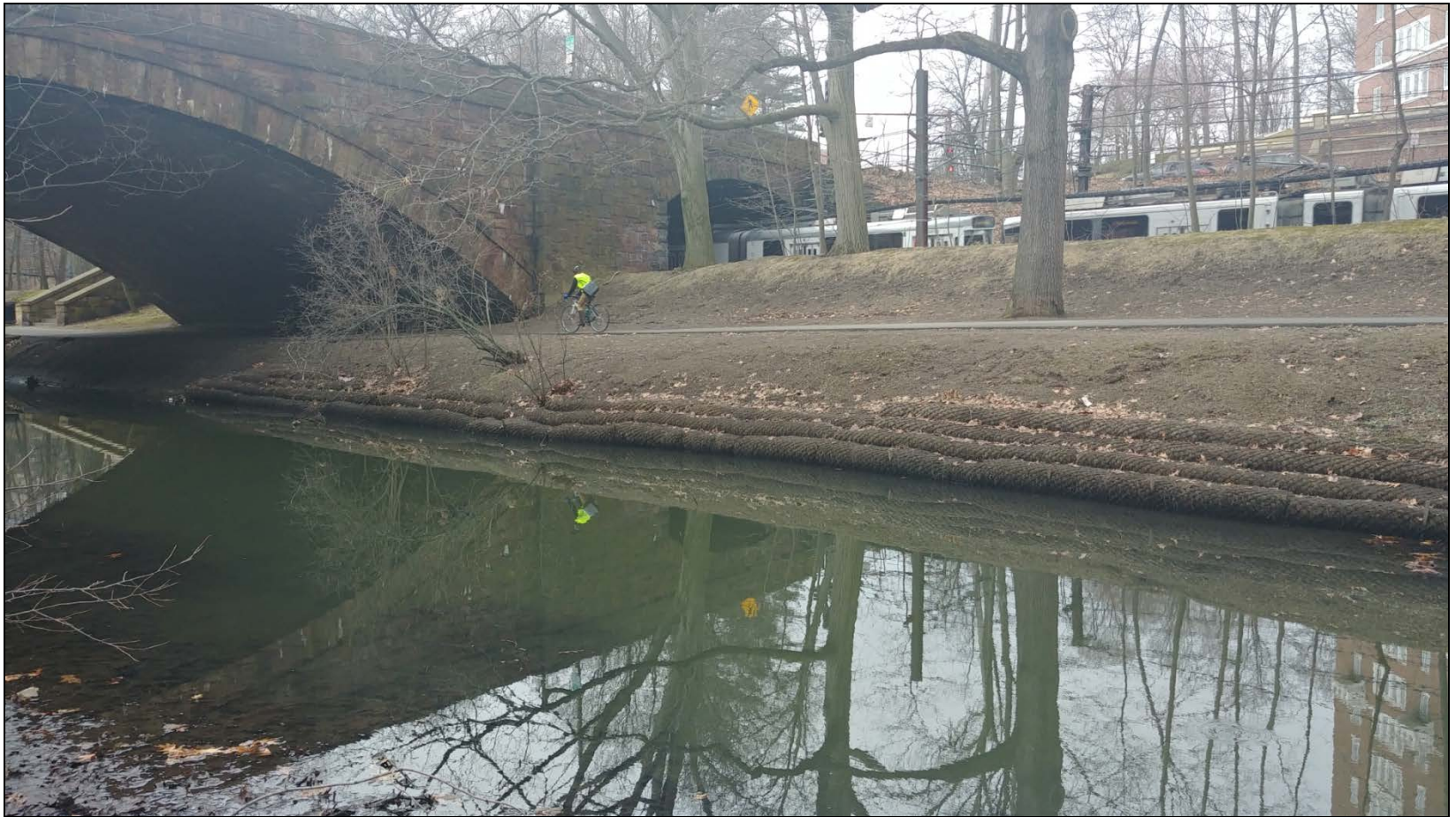
Photograph 8: Erosion control downstream of the Longwood Avenue Bridge.
