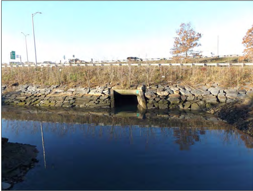
Photo No. 5 - Culvert Outfall (looking west)
