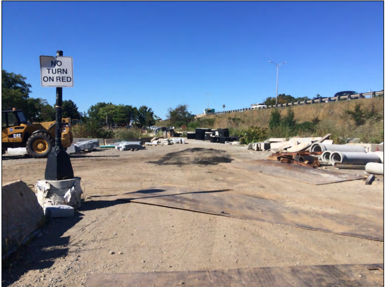
Photo 1: Gravel lot (Study Area) located in Dorchester. I-93 south is visible on the right side of the photo and the depression is visible behind the loader and jersey barriers on the left side of the photo. Stantec. September 13, 2016.
