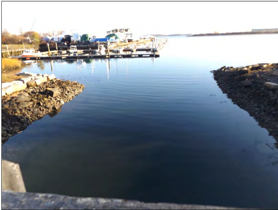
Photo No. 6 – Culvert outfall (looking east) at Neponset River/Marina Bay
