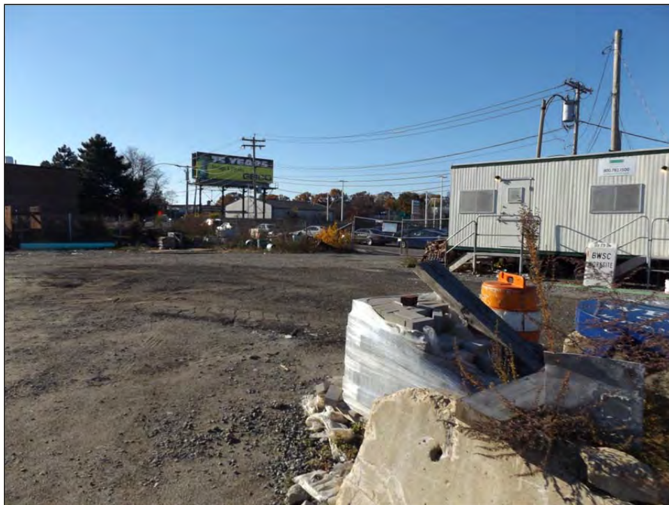
Photo No. 2 – Looking south at site
