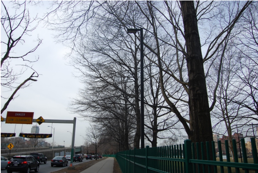
Existing Lights Photos – 1
