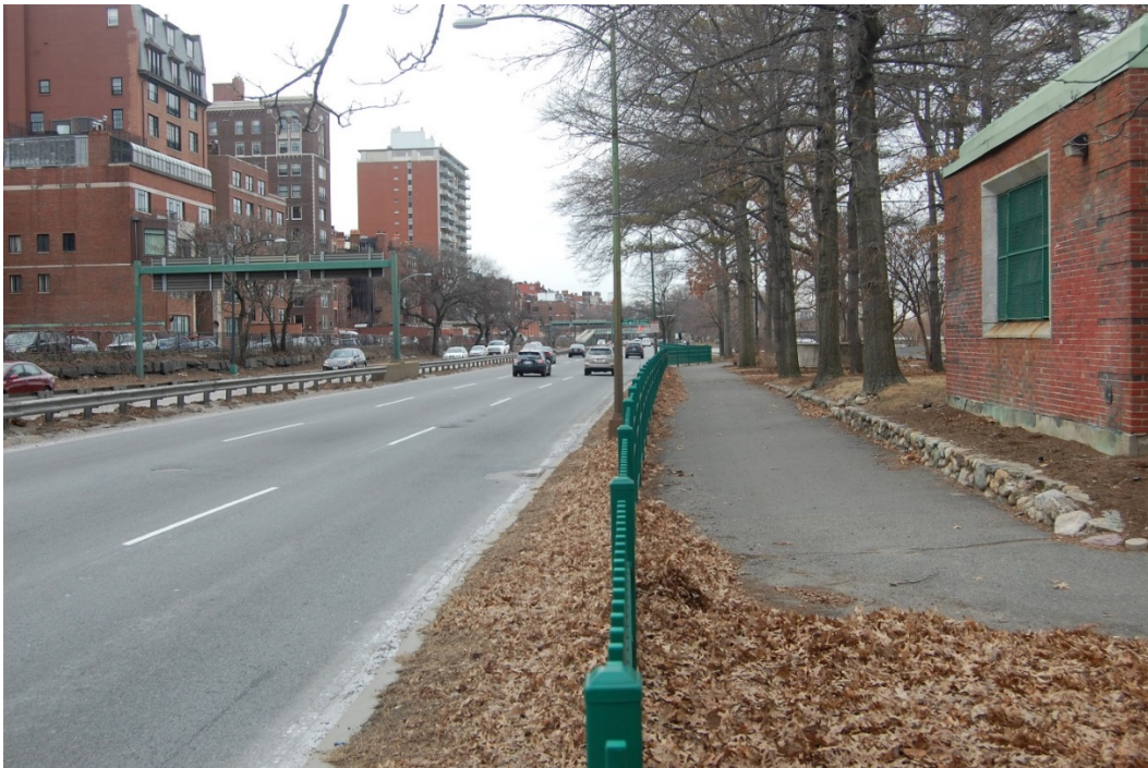
Existing Lights Photos – 2
