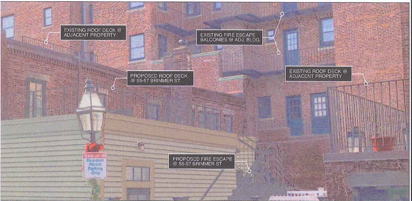
Notes Regarding Ironwork at Existing and Proposed Roof Decks and Fire Escapes
