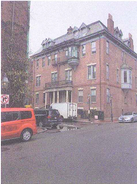
Northwesterly View of Otis Place & Brimmer Street
