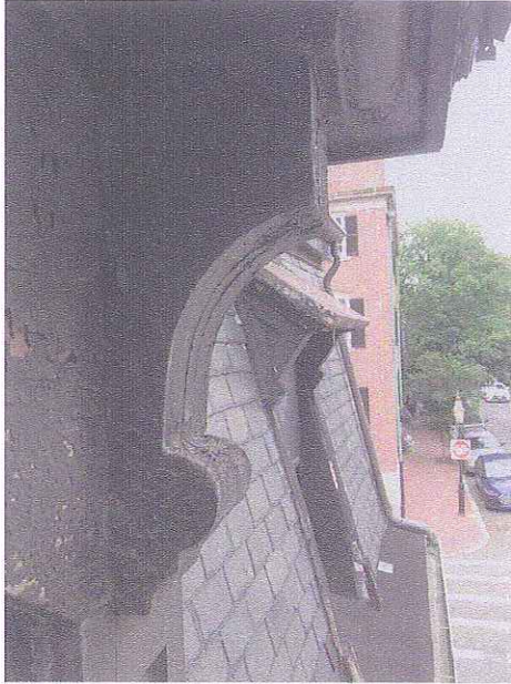
Gable Dormer Bracket in Foreground with Shed Dormer in Background
