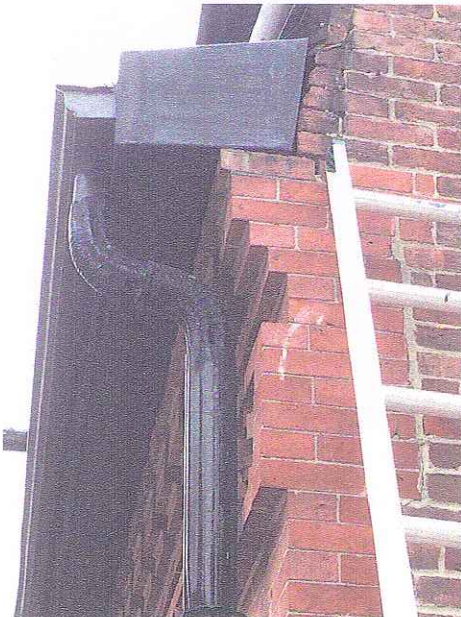
Corbeling Detail at Southeast Corner of Facade
