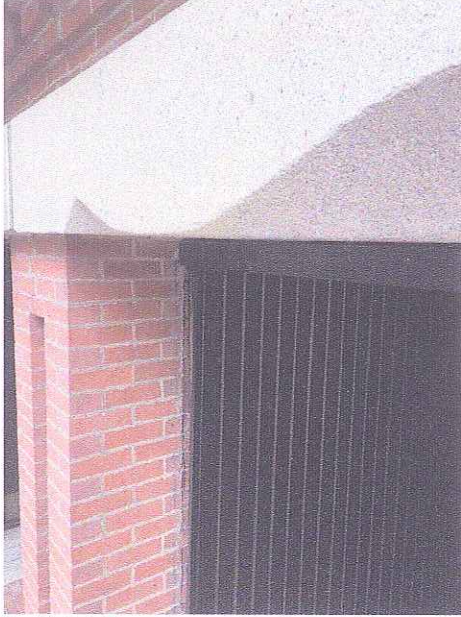
Granite Lintel Over Garage Portico at Chestnut Street
