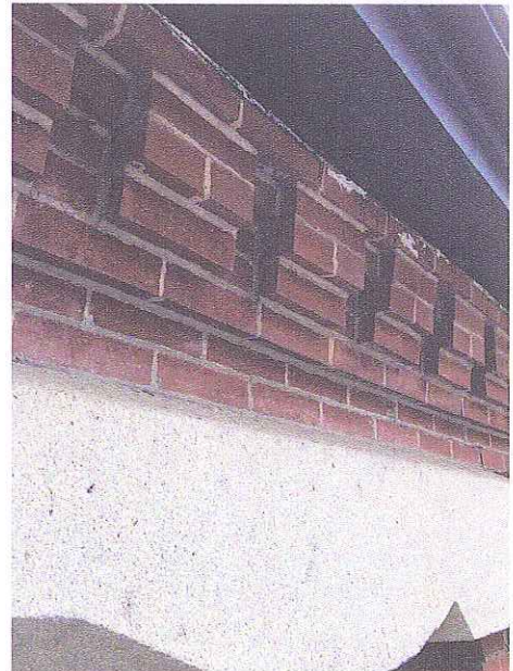
Brick Cobeling Over Granite Lintel on Chestnut Street
