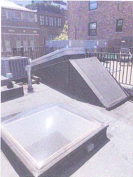
Skylight in Foreground and ACCU at Left on 57 Brimmer Street Building; Raised Hatch, Roof Deck & Air Handlers Beyond on Adjacent Building
