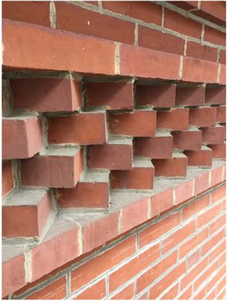
Rotated Brick Banding on Chestnut Street Facade
