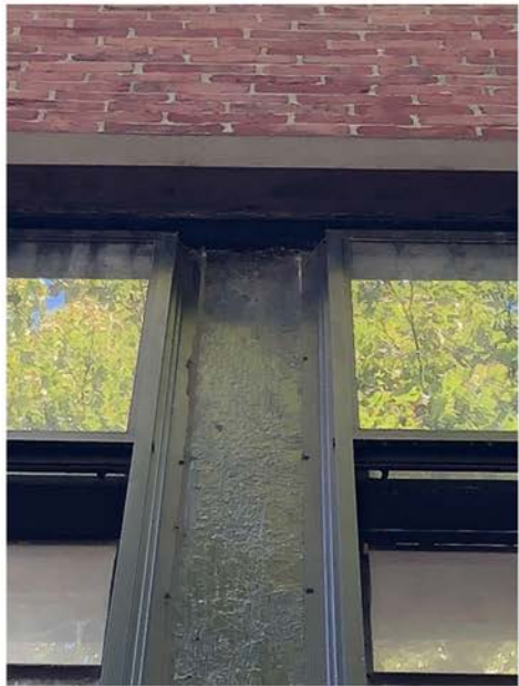
Brownstone Lintel, Wood Mullion and Exterior Storm Window at Second Floor 6-over-6 Sash
