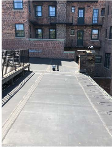
Looking West From Back Edge of Roof; Three Adjacent Properties with Same Roof Slope with Five-Story Brick Building Beyond
