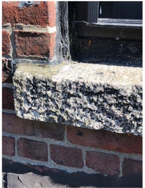
Replacement Granite Sill on North Facade of Second Floor to be Reused and Painted to Match Color of Brownstone
