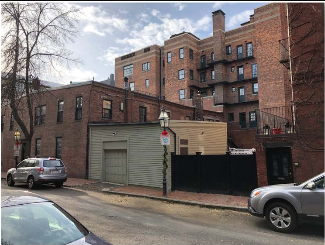
Photograph of Existing Conditions at Rear One-Story Structure
