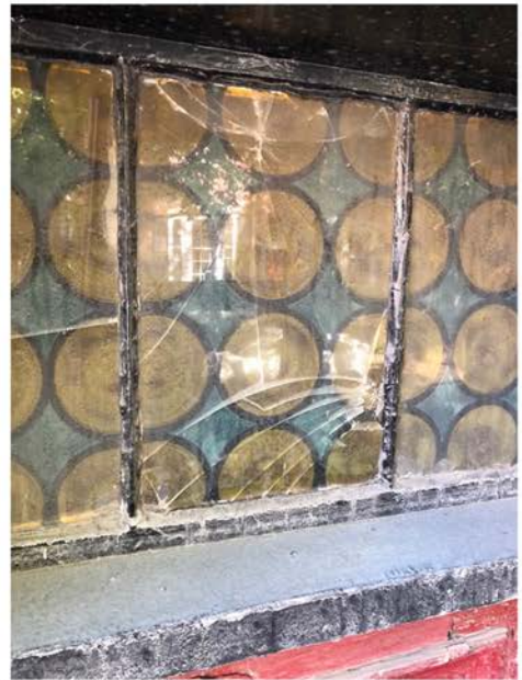
Glass Transom Sash to be Repaired; Broken Glass to be Replaced with Restoration Glass; Interior Decorative Panel of Faux Stained Glass to be Removed
