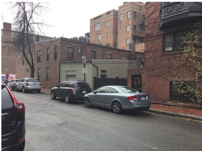
Southwesterly View of Building from Brimmer Street
