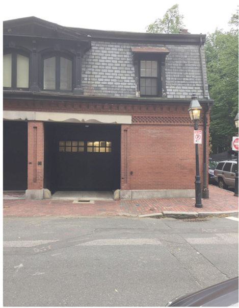
South Facade at Chestnut Street with Mansard Roof Above Brick Street Level Facade & Garage Portico; In-Kind Repair and Restoration Intended for Facade
