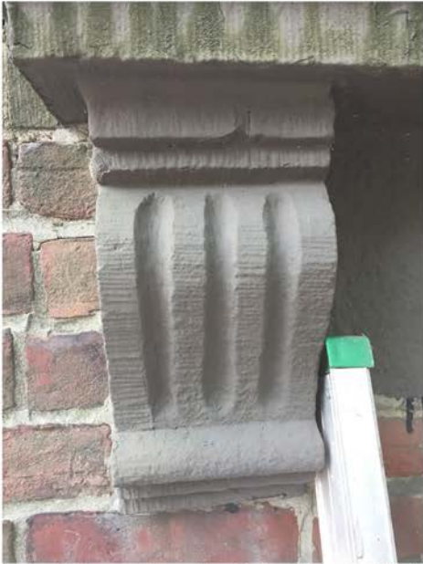
Carved Brownstone Bracket at Hooded Lintel Above 57 Brimmer Street Entrance Door
