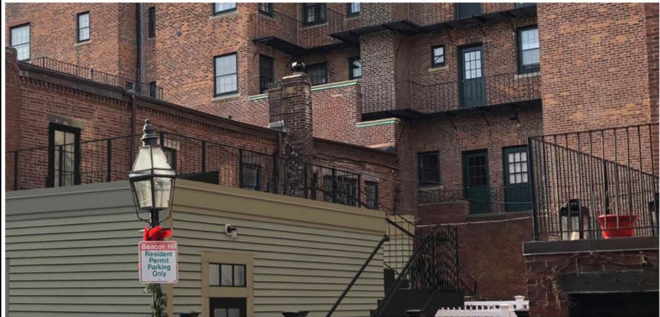
Detail of Reconstructed Rear Structure in Context of Neighborhood Features
