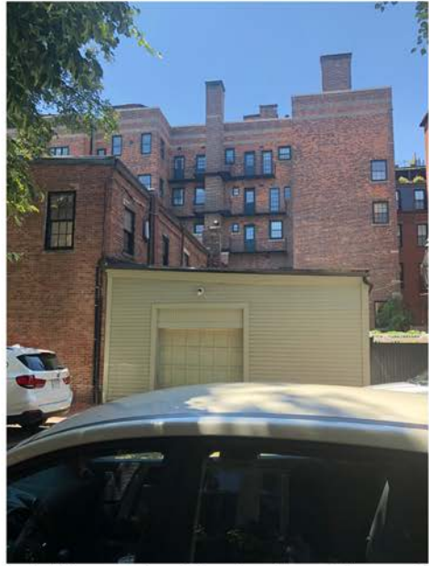
Westerly View of Rear Structure from Brimmer Street
