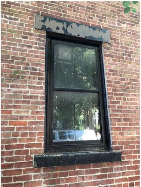
Second of Two 2-over-2 Sash on Brimmer Street Facade; Sash to be Repaired; Frame & Storm Window Replaced; Brownstone Sill & Lintel to be Re-Set and Paint Removed
