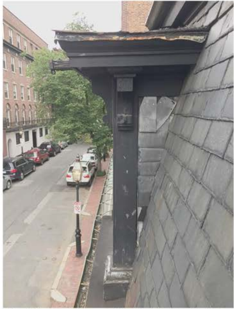
Looking West at Mansard to Gable Roofed Dormer Shared with Neighboring Twin Property; Disrupted Slates on Sidewall & Rusting Metal Roof
