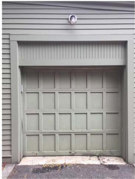
Contemporary Garage Door at One-Story Addition with Paneling above Transom Bar; Door to be Replaced with Fixed Door to Match Main Garage Door on Chestnut St; Transom Panel to be Replaced with 6-Light Glass Sash
