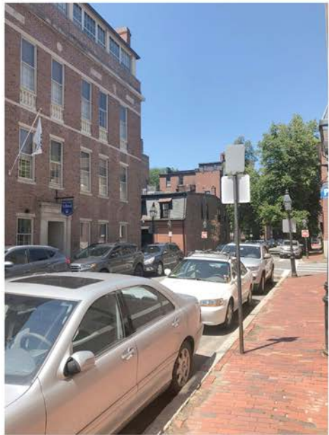
S1: View from Middle of Brimmer Street Garage; No Visible Change to Skyline From This View
