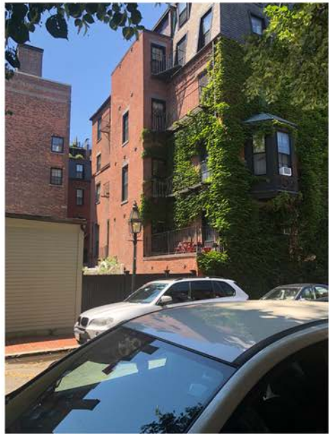
Adjacent Buildings on Otis Place Abutting 57 Brimmer Street (At Left)
