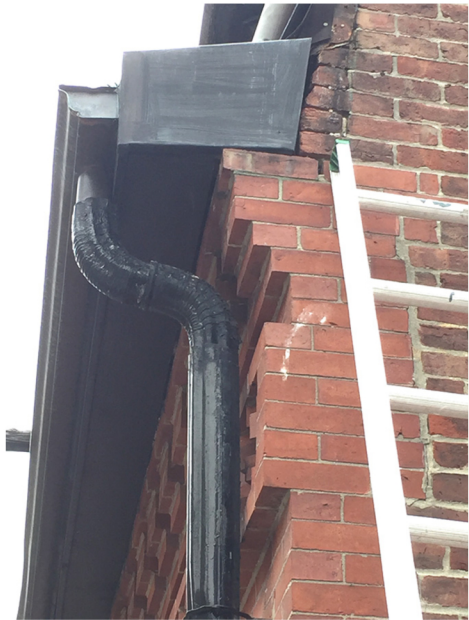
Corbeling Detail at Southeast Corner of Facade
