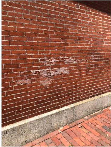
Granite Plinth and Brick Facade at Chestnut Street
