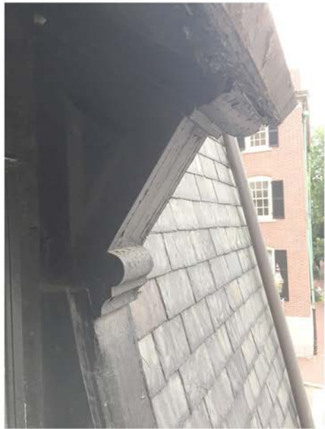
Bracket at Shed Dormer Roof with Slates Beyond
