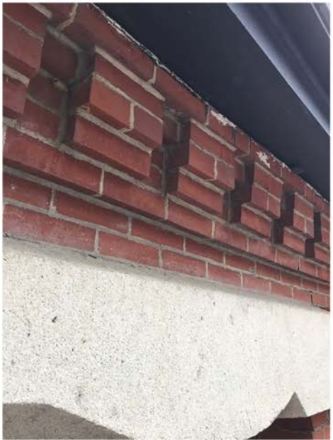
Brick Coping Over Granite Lintel on Chestnut Street
