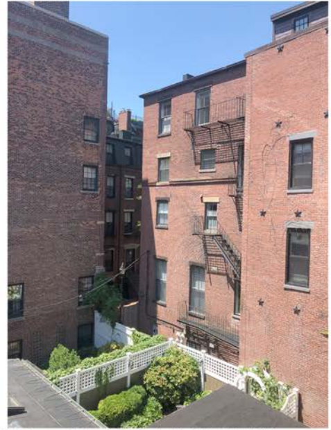
Northwesterly View of Abutting Buildings from Upper Roof of 57 Brimmer Street
