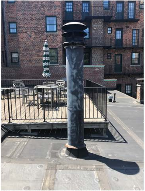
Flue and Roof Deck at Neighbor's Property
