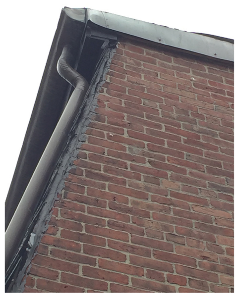
Southeast Corner Showing Transition from Mansard Roof Slope to Adjacent Brick; Roofing Cement to be Removed and Copper Flashing to be Installed
