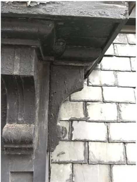
Corner Detail of Bracketed Eave at Gable Dormer
