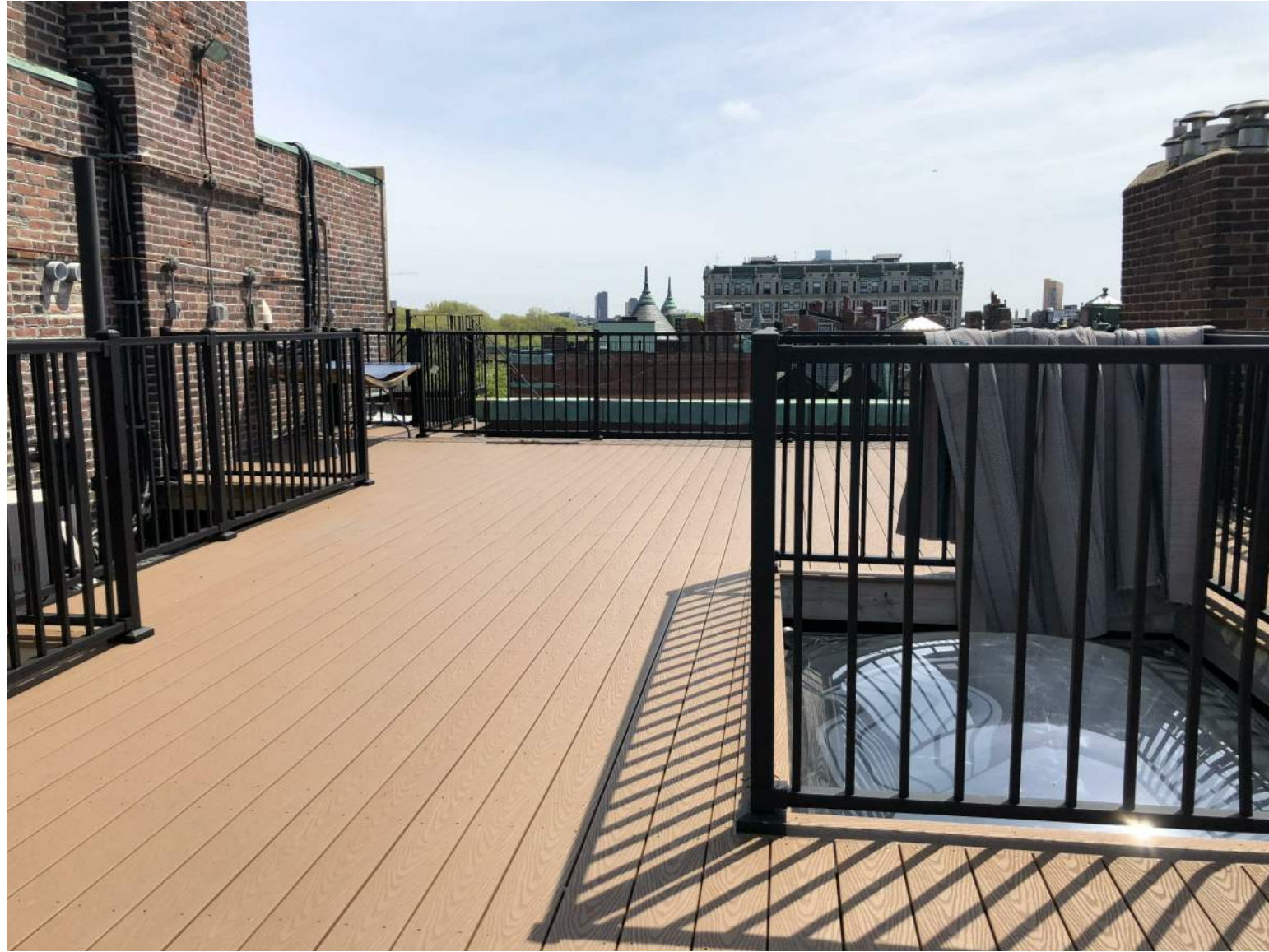
EXISTING ROOF DECK AT 7 BAY STATE ROAD
