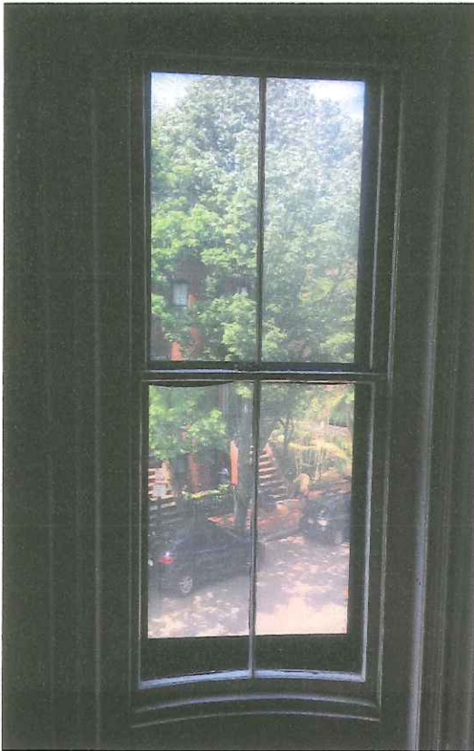
Bedroom level right window (interior view)
