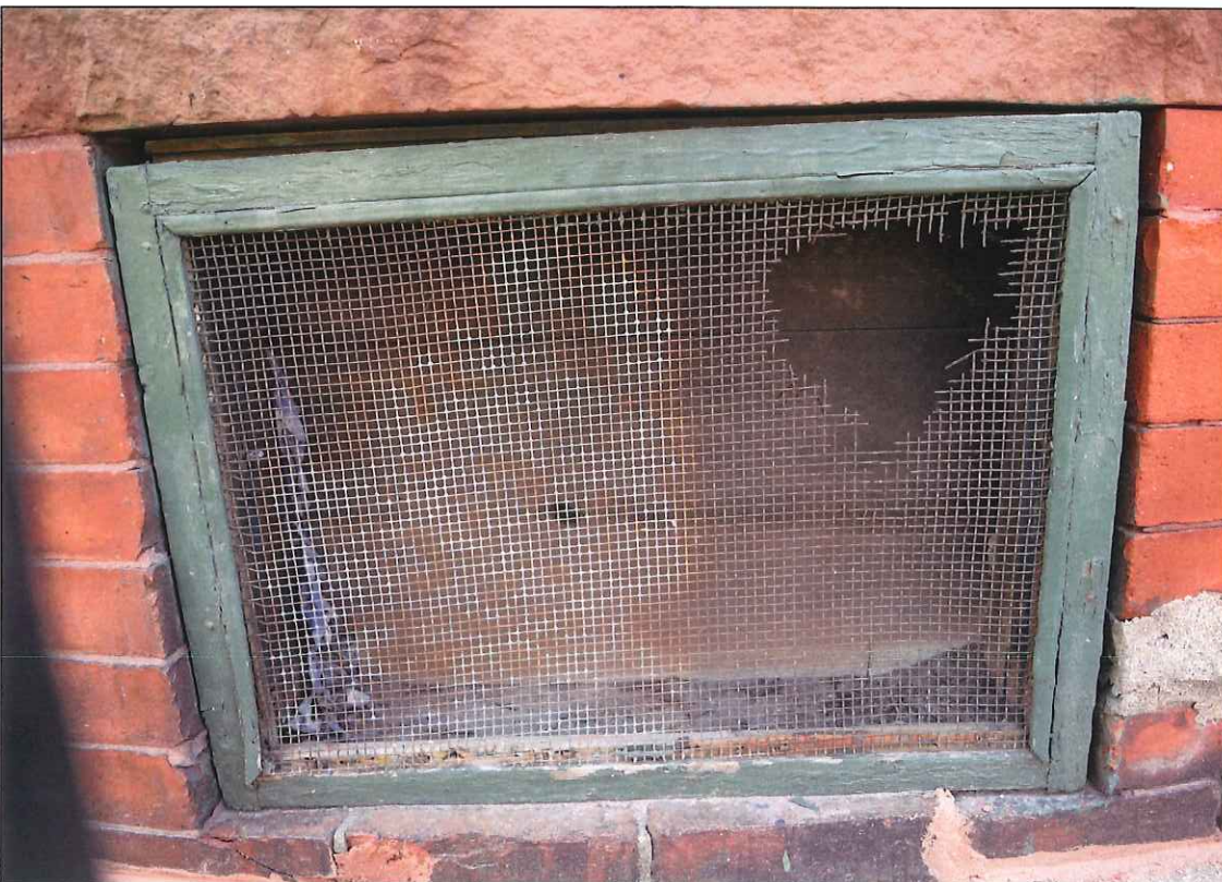
6. North elevation, basement, window 2
