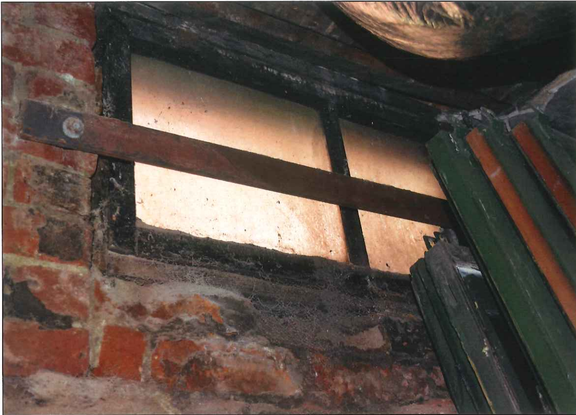
37. East elevation, basement, window 15
