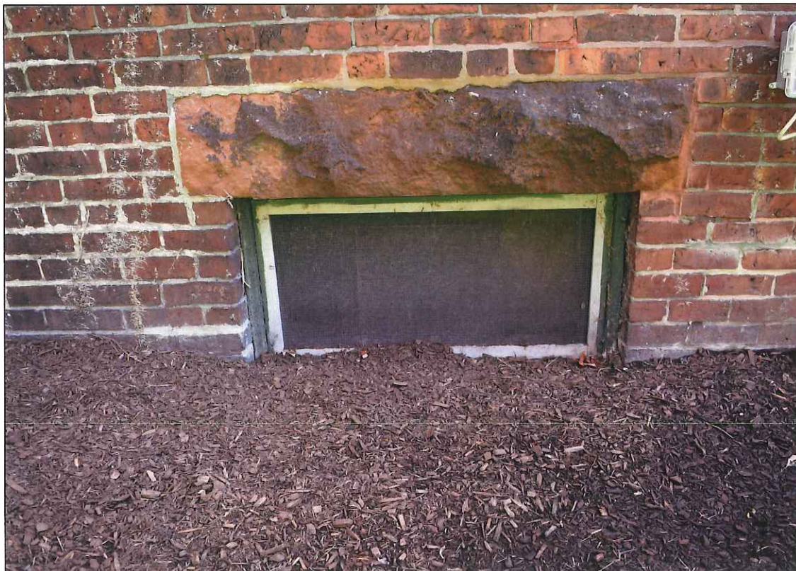
42. East elevation, basement, window 17
