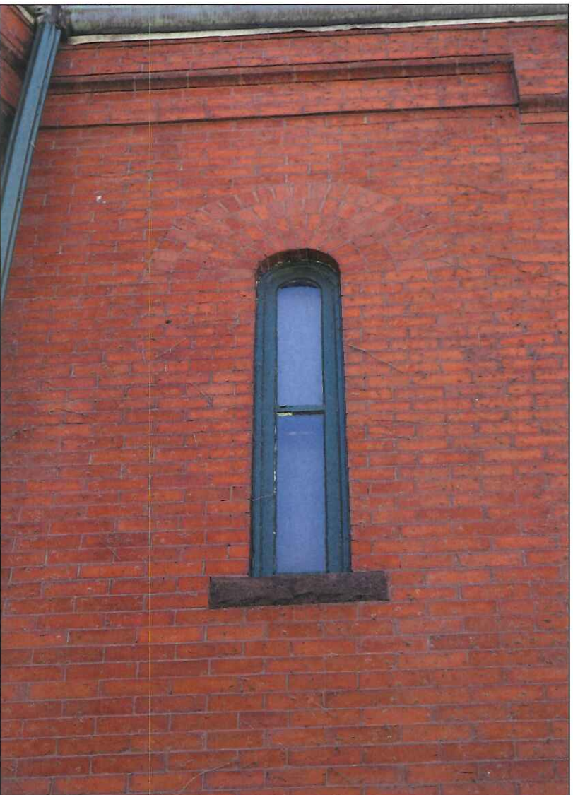
24. North elevation, second floor, window 10
