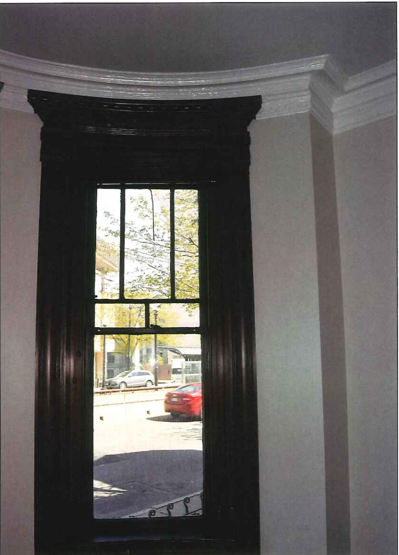
9. North elevation, first floor, window 4
