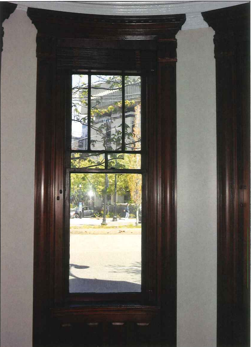
11. North elevation, first floor, window 5
