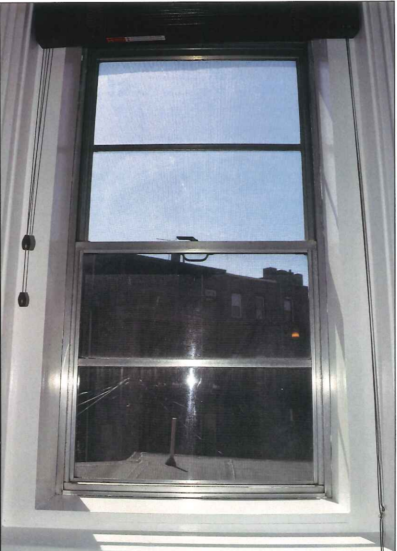
90. South elevation, second floor, window 39
