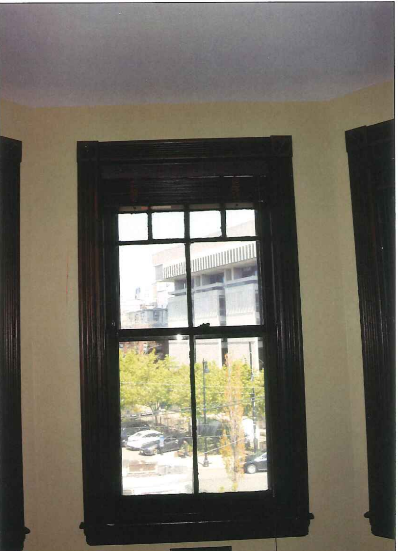
29. North elevation, third floor, window 12
