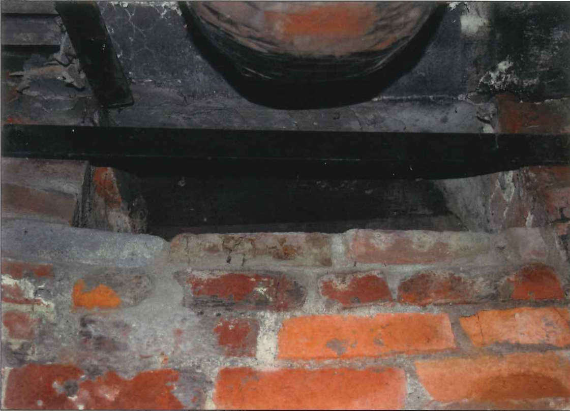
5. North elevation, basement, window 2
