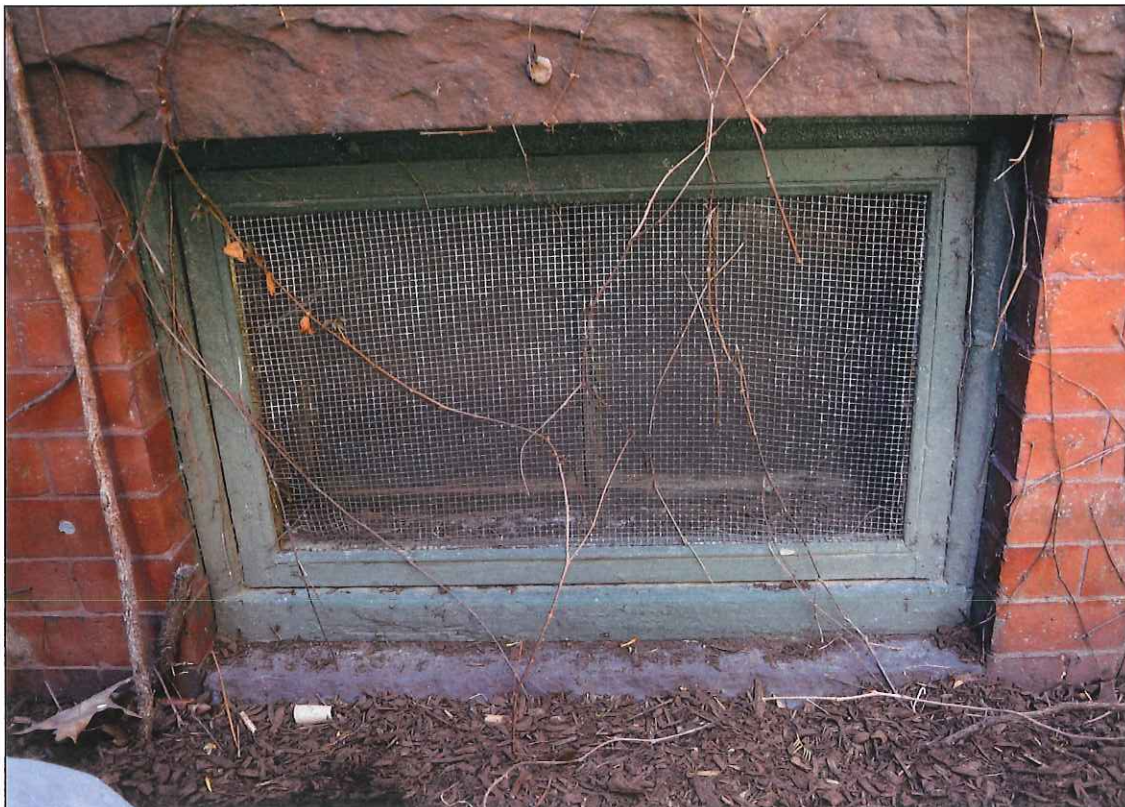
36. East elevation, basement, window 14
