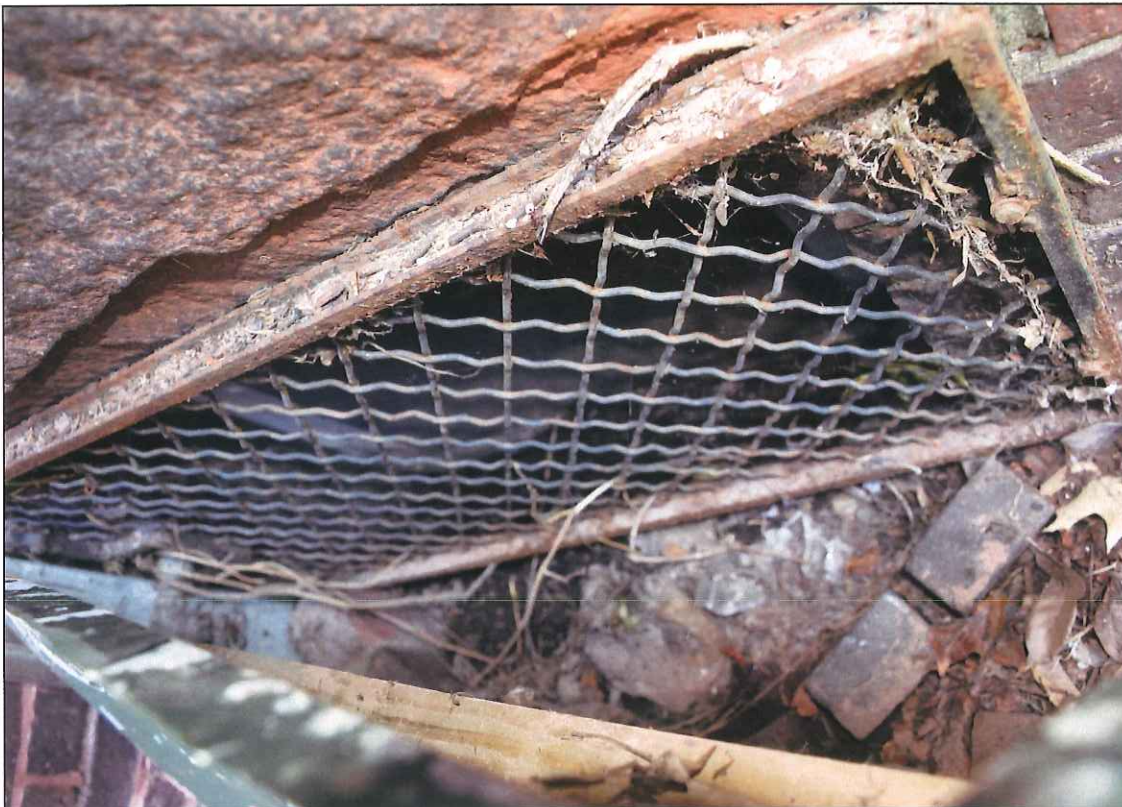
40. East elevation, basement, window 16
