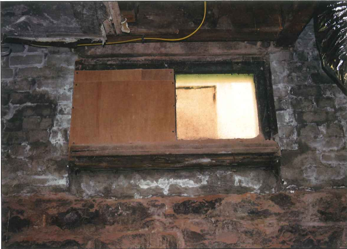
41. East elevation, basement, window 17
