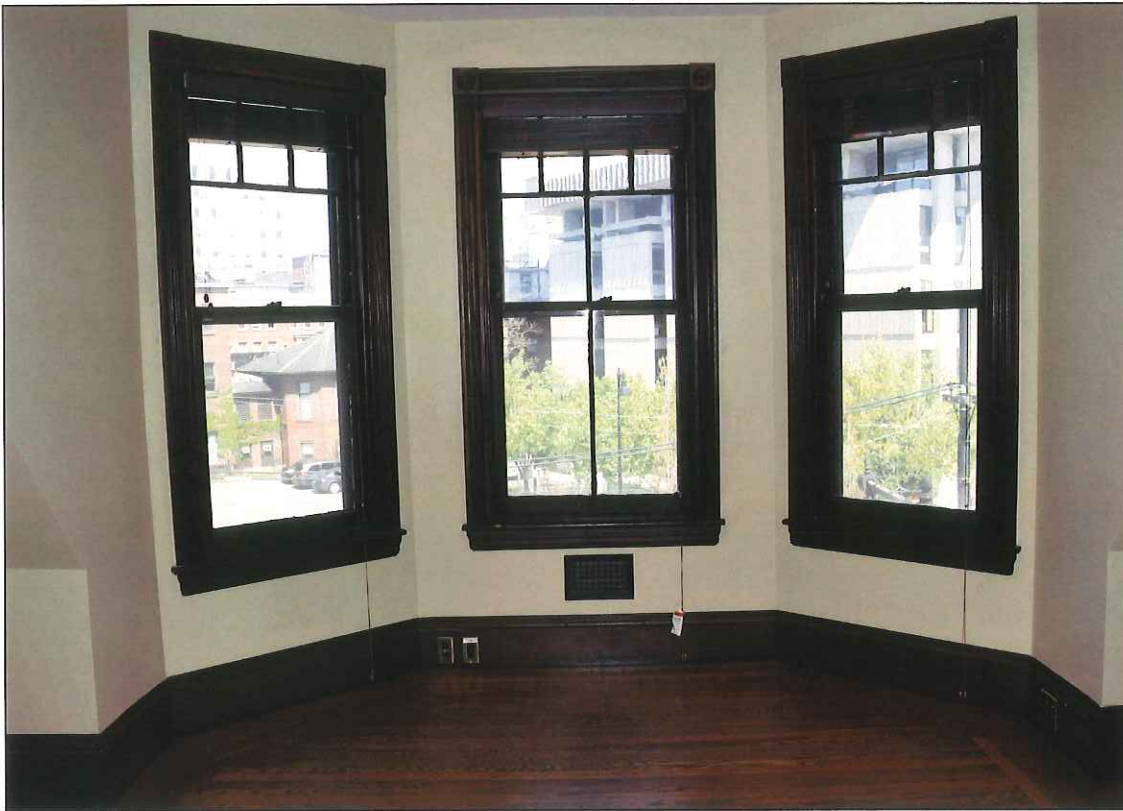
25. North elevation, third floor, windows 11-13
