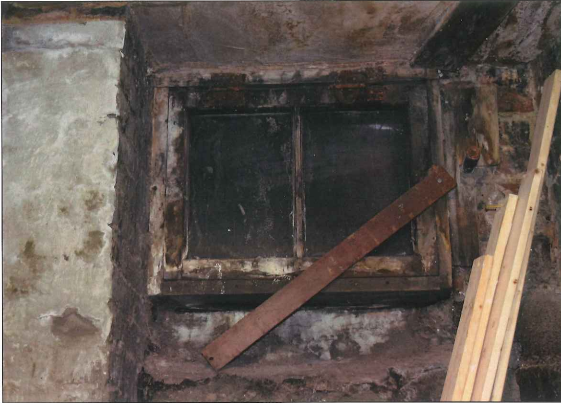
39. East elevation, basement, window 16
