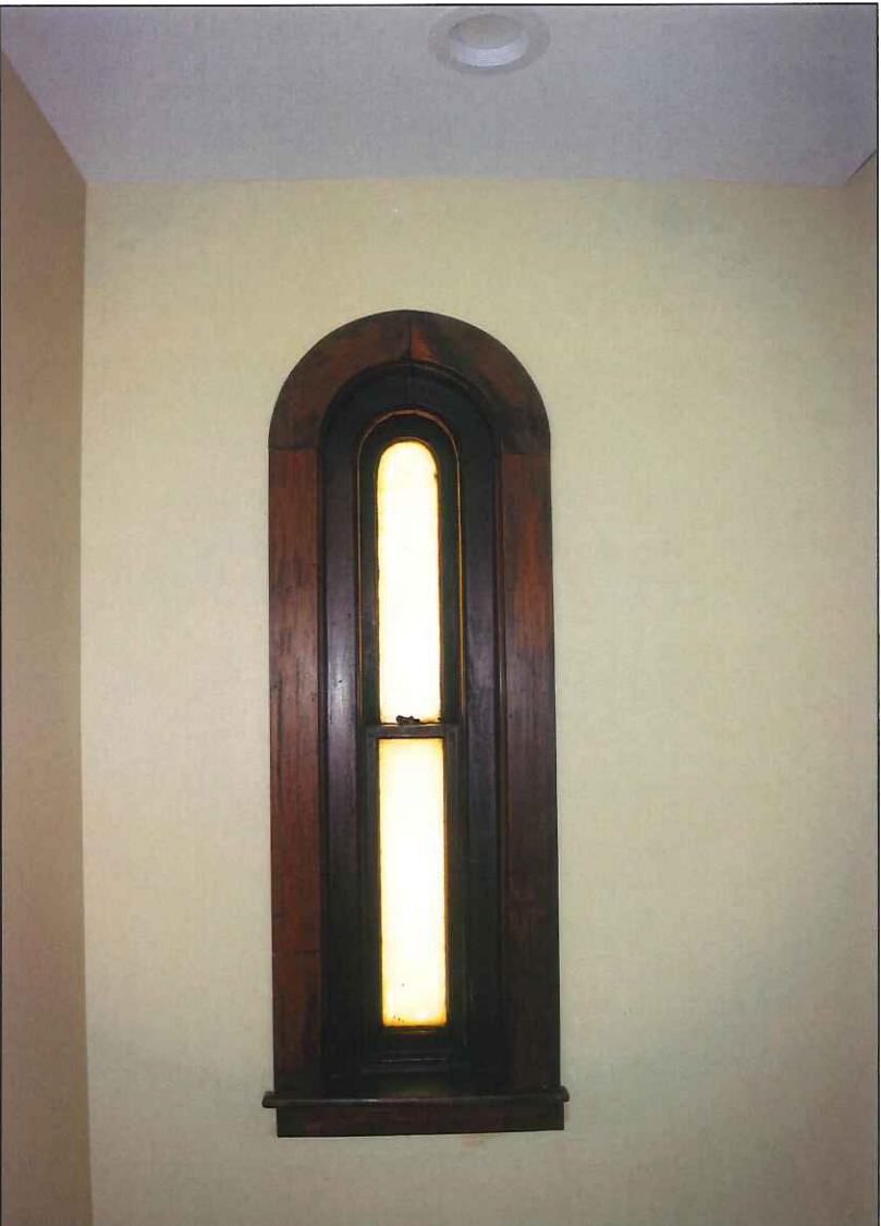
23. North elevation, second floor, window 10
