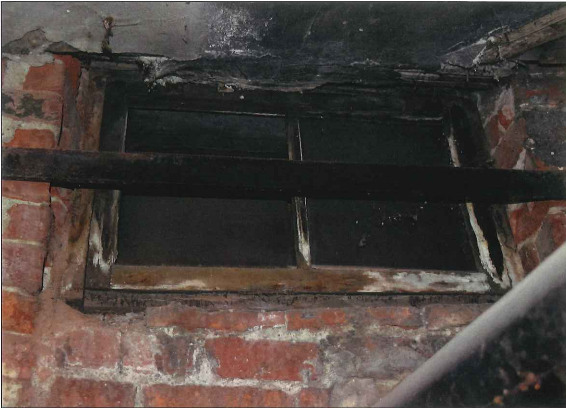
7. North elevation, basement, window 3
