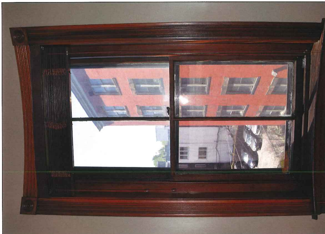
93. South elevation, third floor, window 40
