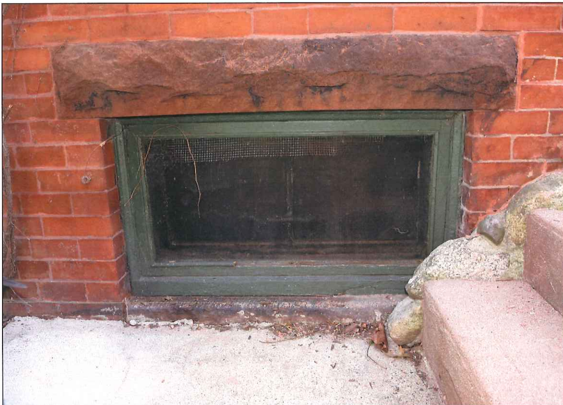
38. East elevation, basement, window 15
