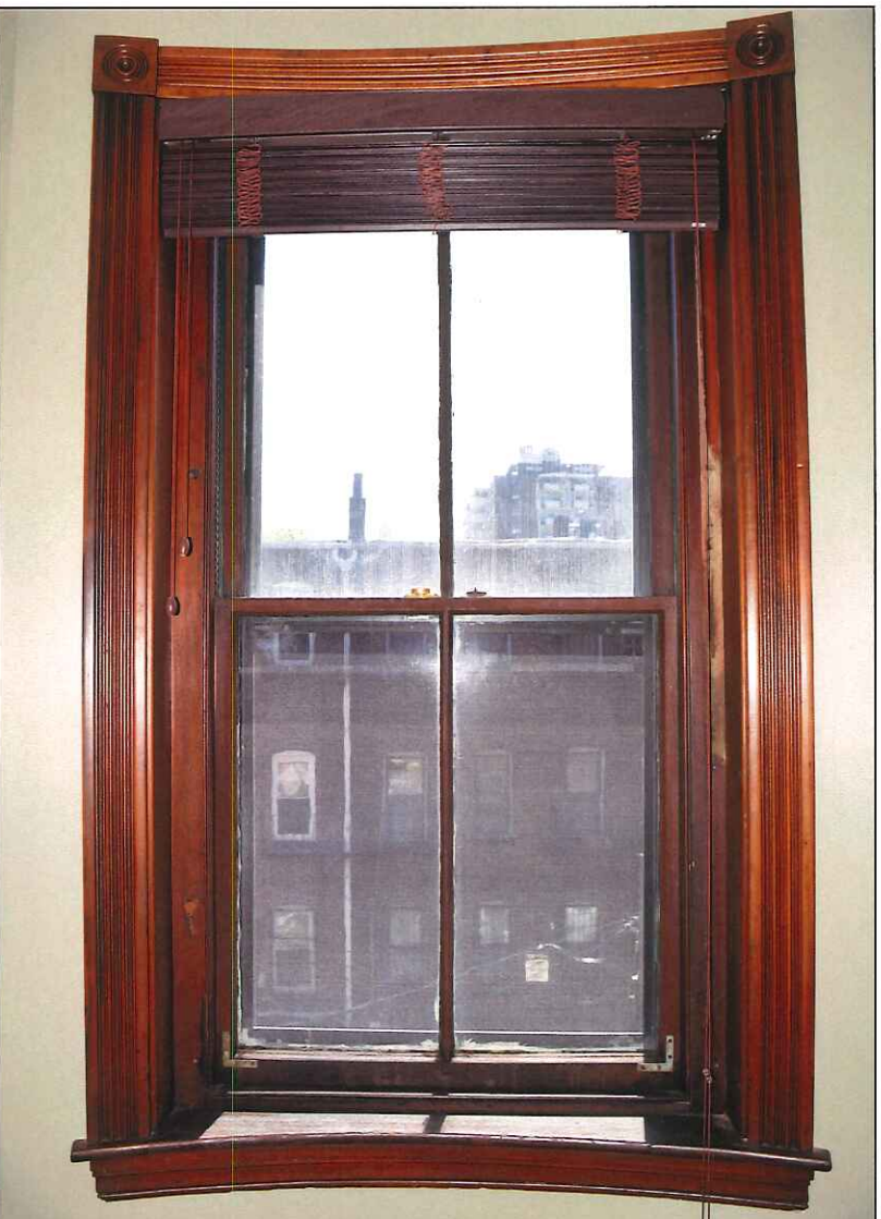
95. South elevation, third floor, window 41
