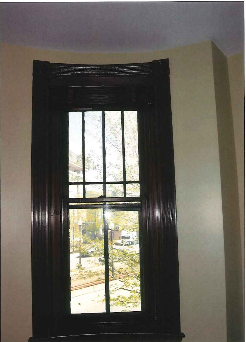
15. North elevation, second floor, window 7
