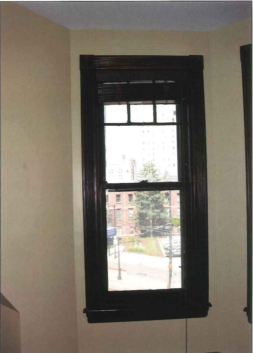
31. North elevation, third floor, window 13
