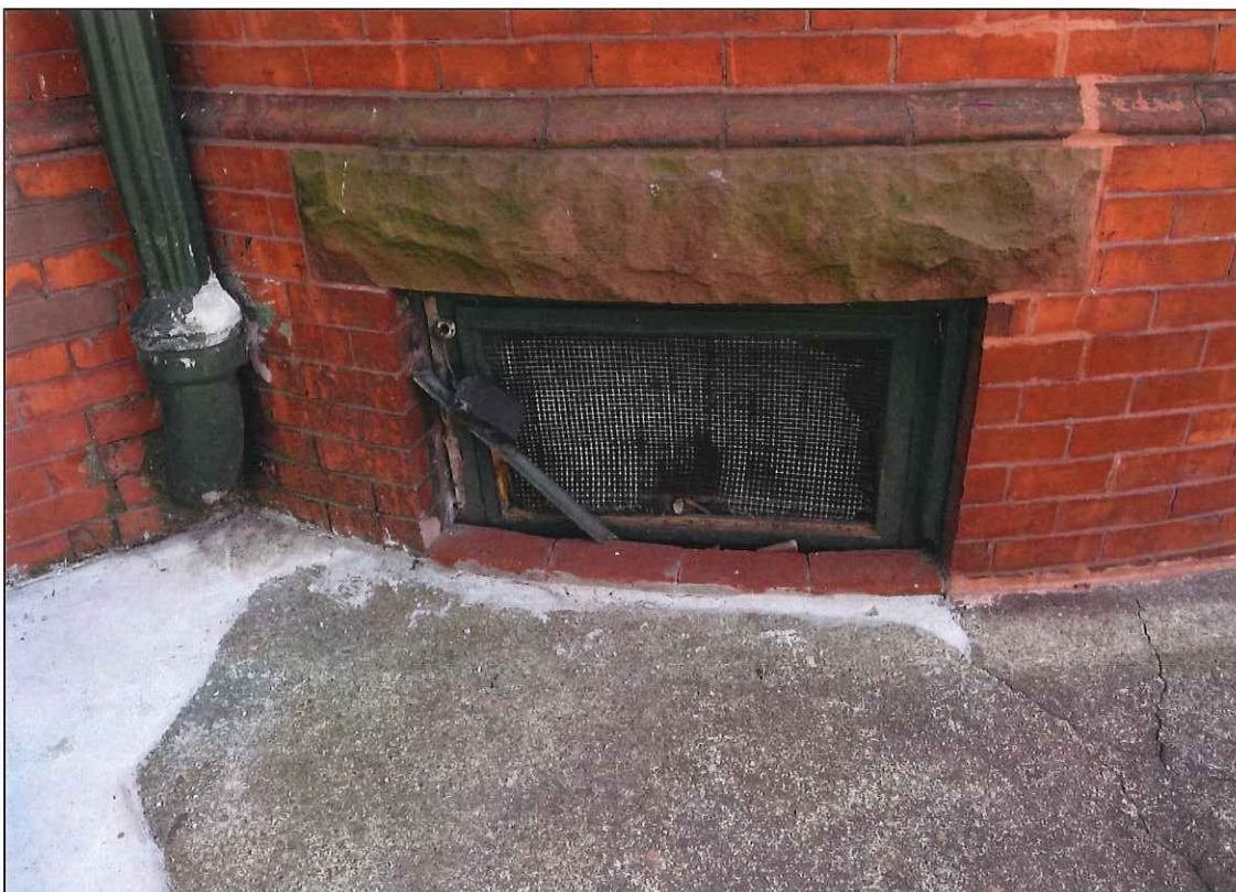
4. North elevation, basement, window 1
