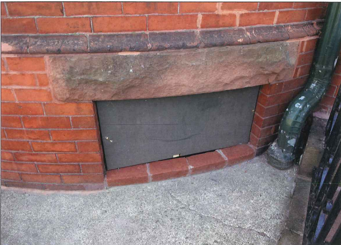
8. North elevation, basement, window 3
