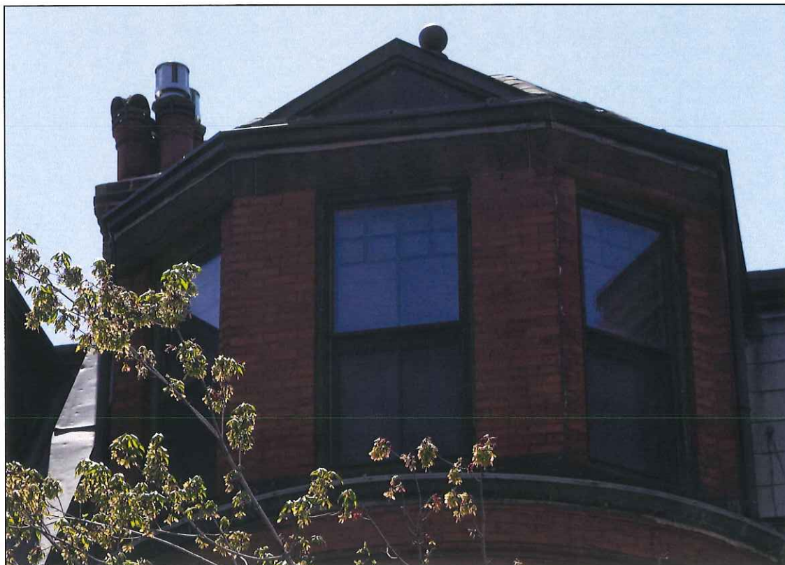
26. North elevation, third floor, windows 11-13
