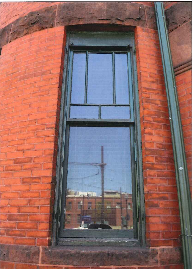
14. North elevation, first floor, window 6
