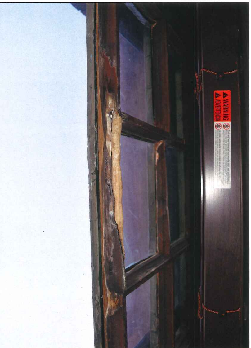
28. North elevation, third floor, window 11
