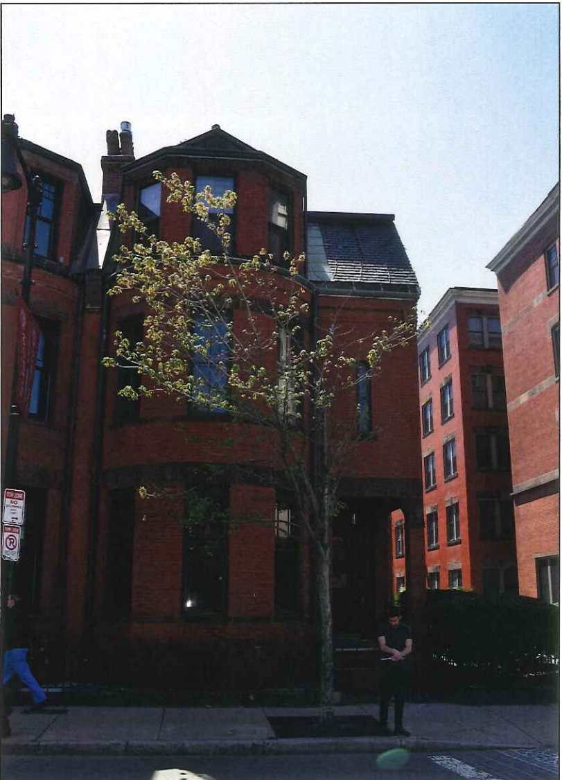
1. North elevation windows
