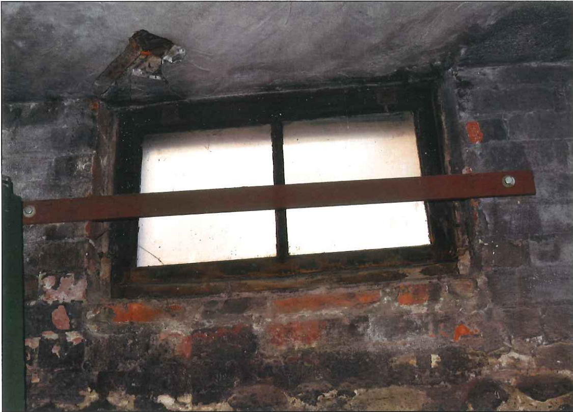
35. East elevation, basement, window 14
