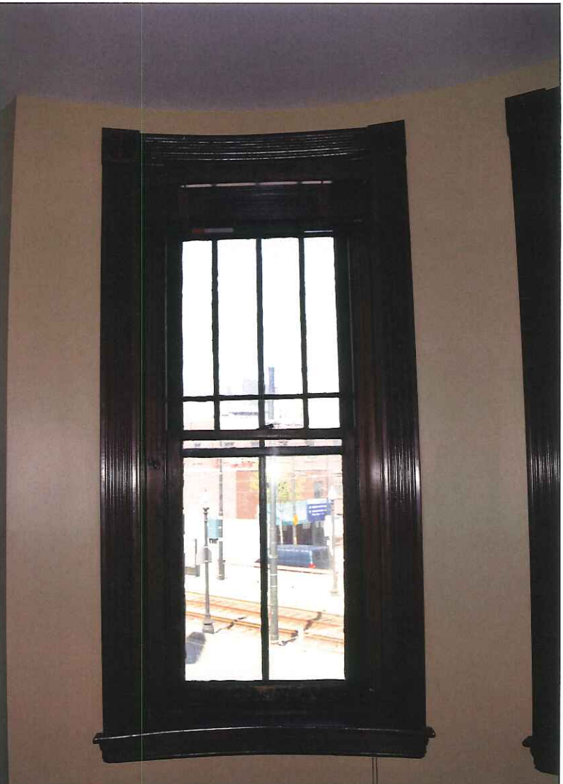
20. North elevation, second floor, window 9
