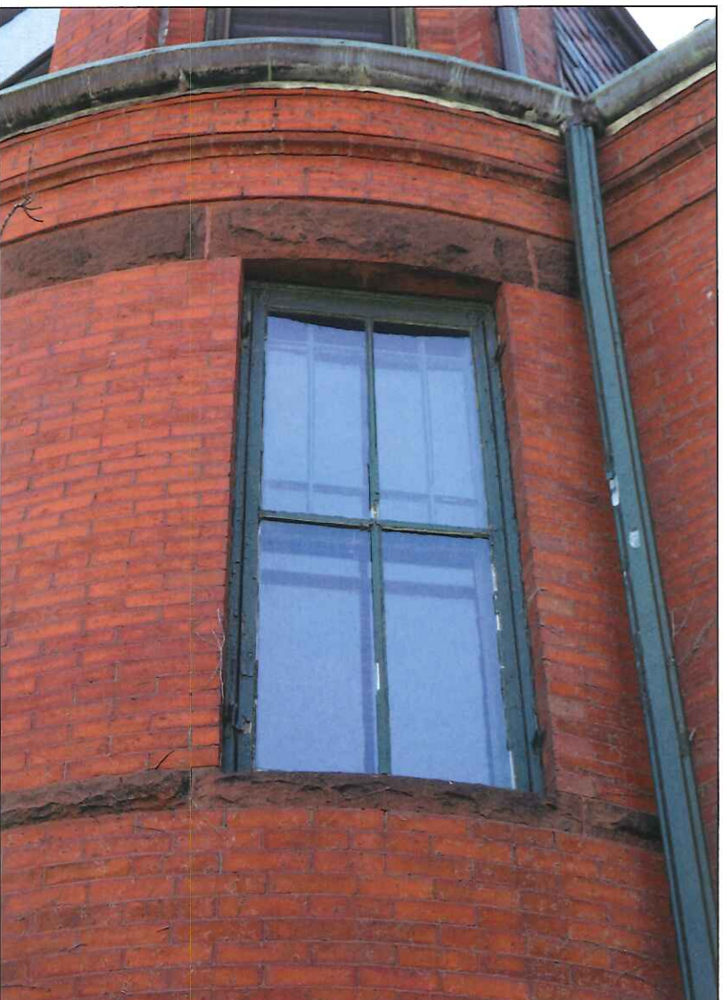
22. North elevation, second floor, window 9
