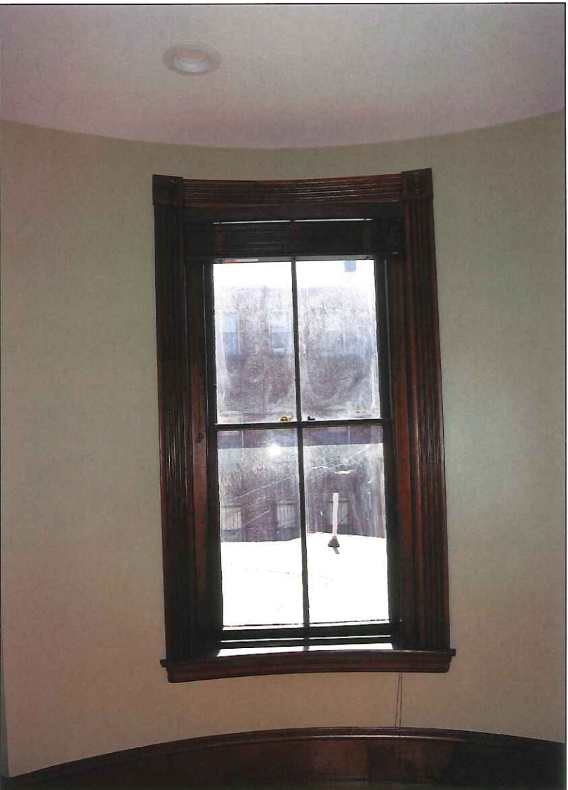
88. South elevation, second floor, window 38
