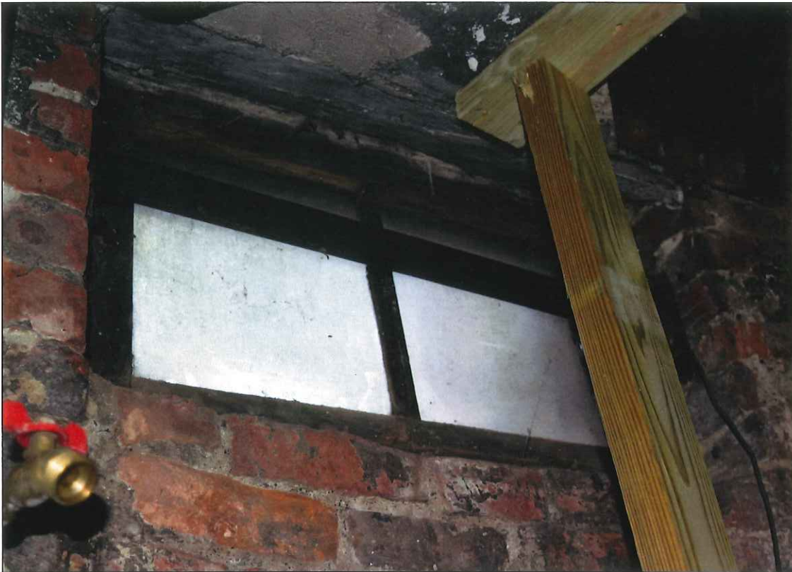
3. North elevation, basement, window 1
