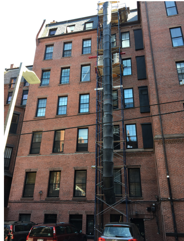
exterior - rear facade
