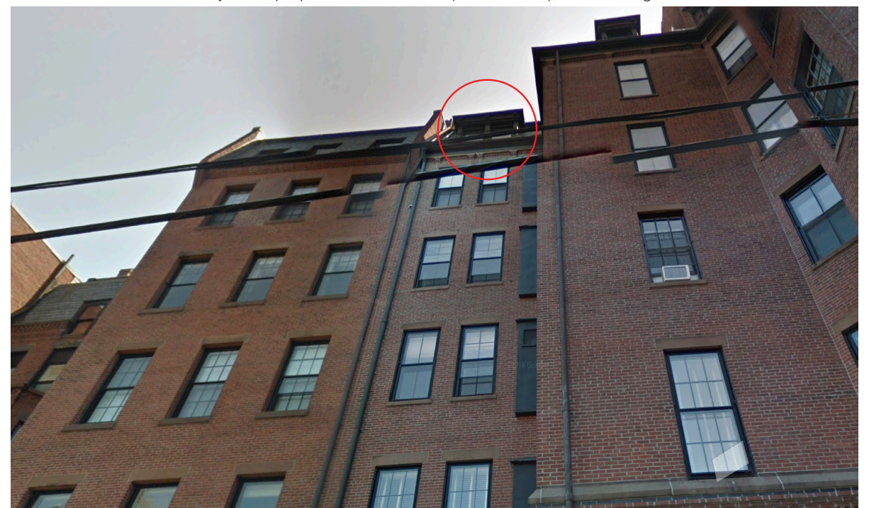
street view from Public Alley 425 - proposed Windows K1 (circled in red); see drawing
