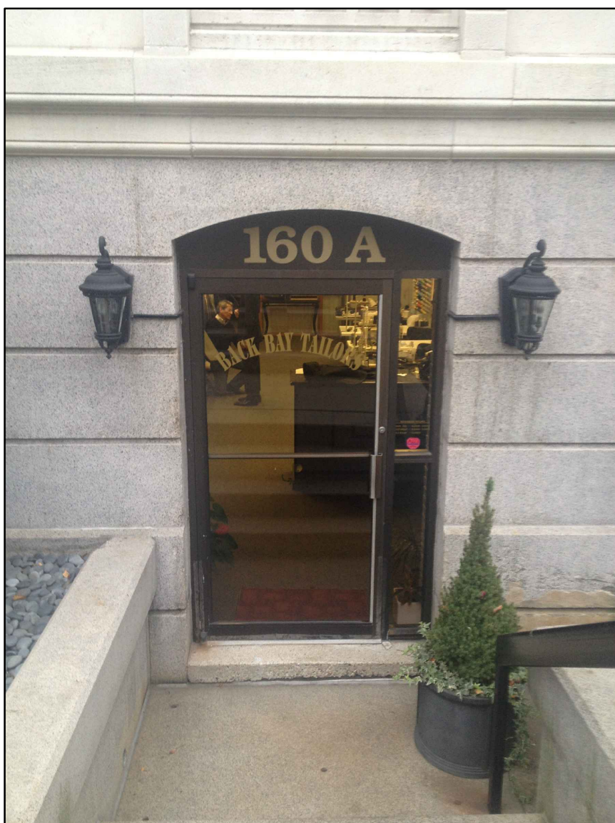
B - 160A COMMONWEALTH AVE. - EXISTING ENTRY
