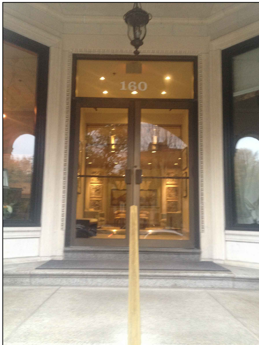
A - 160 COMMONWEALTH AVE. - EXISTING ENTRY
