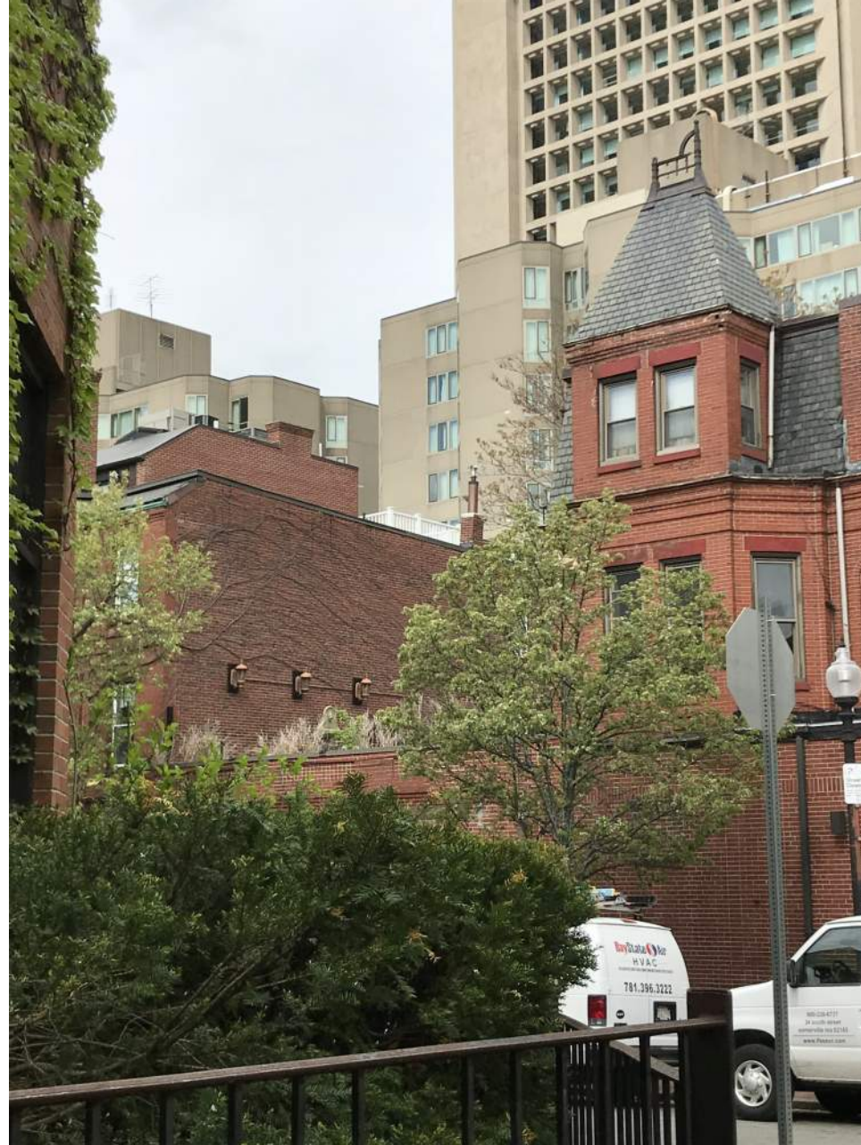
VISIBLE RAILING AT 107 ST. BOTOLPH STREET
