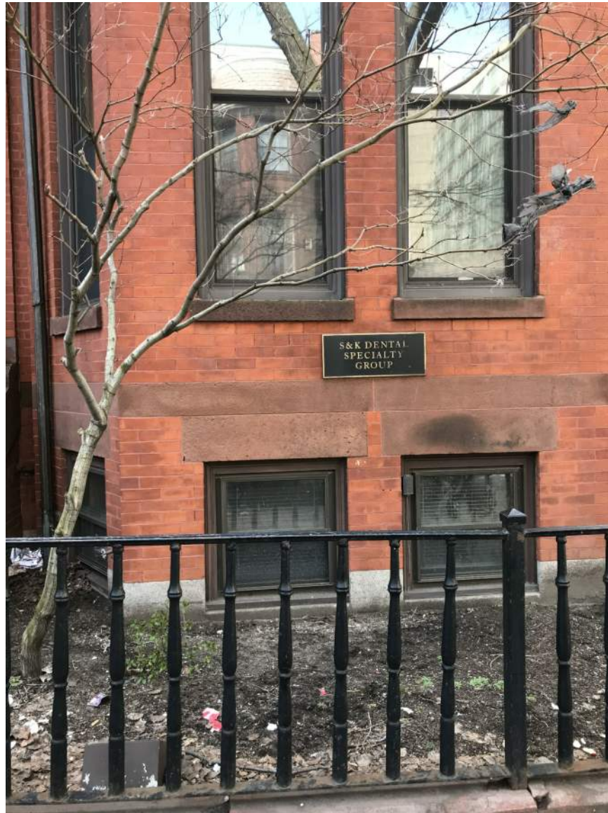
PARTIAL FRONT ELEVATION - NON-HISTORIC REPLACEMENT WINDOWS
