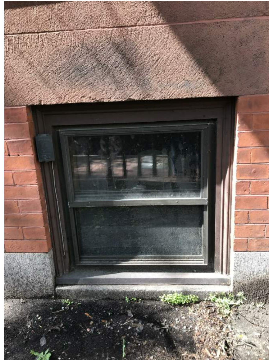
PARTIAL FRONT ELEVATION - NON-HISTORIC REPLACEMENT WINDOWS
