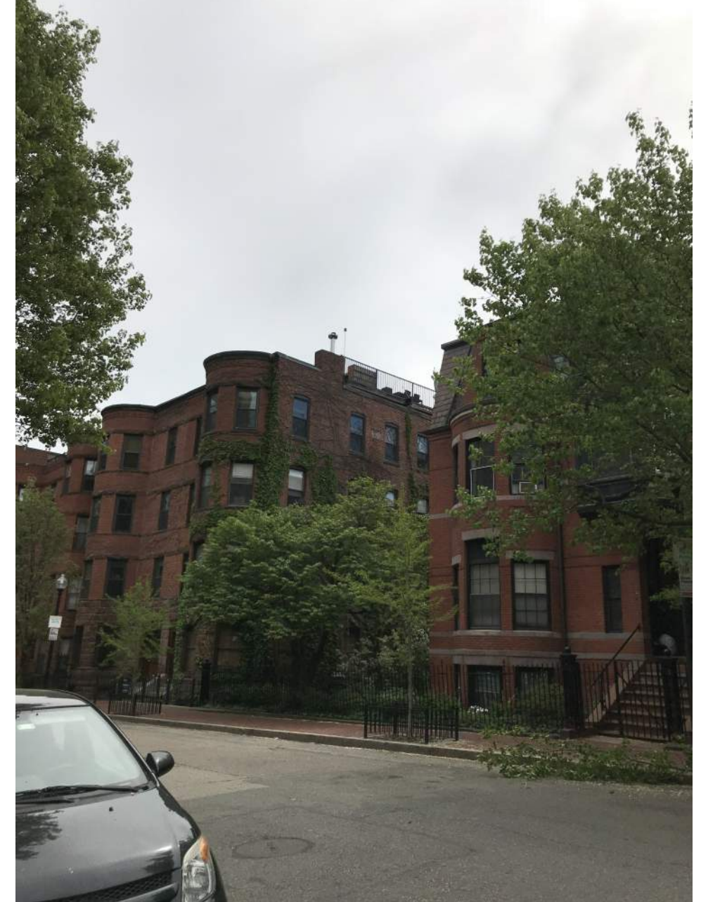
VISIBLE RAILING AT 94 ST. BOTOLPH STREET
