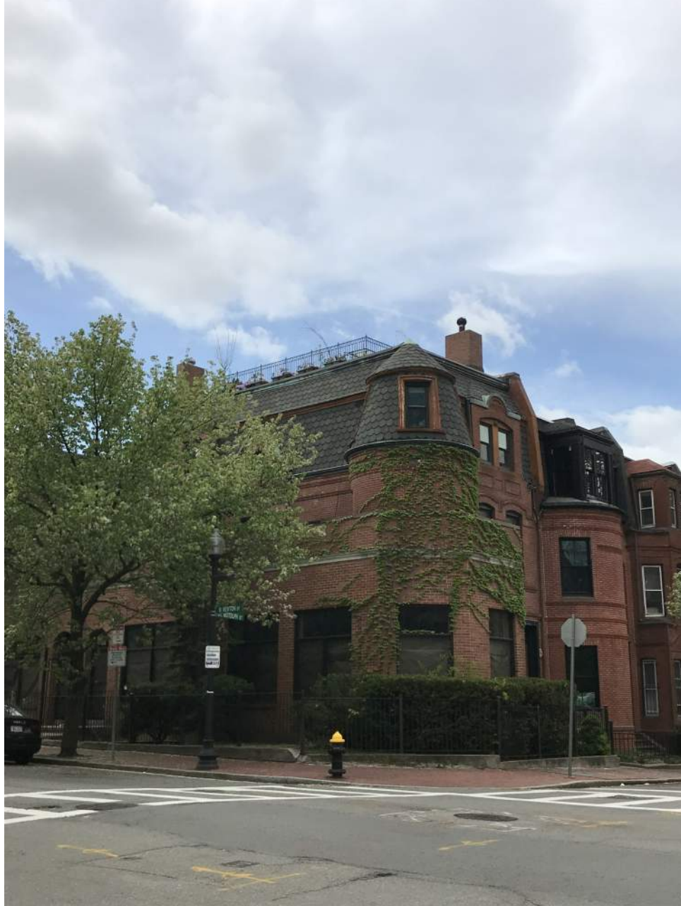
VISIBLE RAILING AT 250 W. NEWTON STREET
