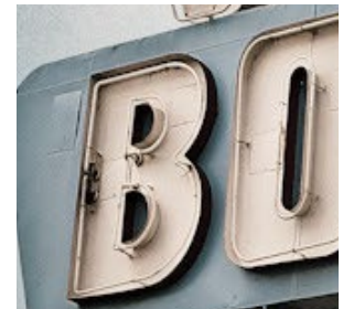
Fabricated letter with open face traced with white neon
