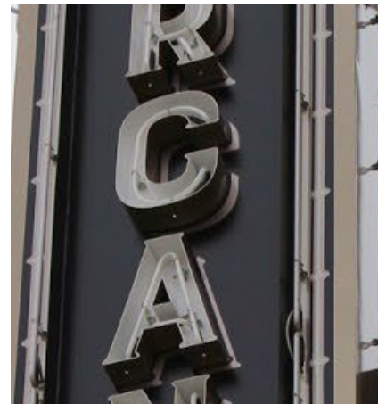
Fabricated letter with open face traced with white neon
