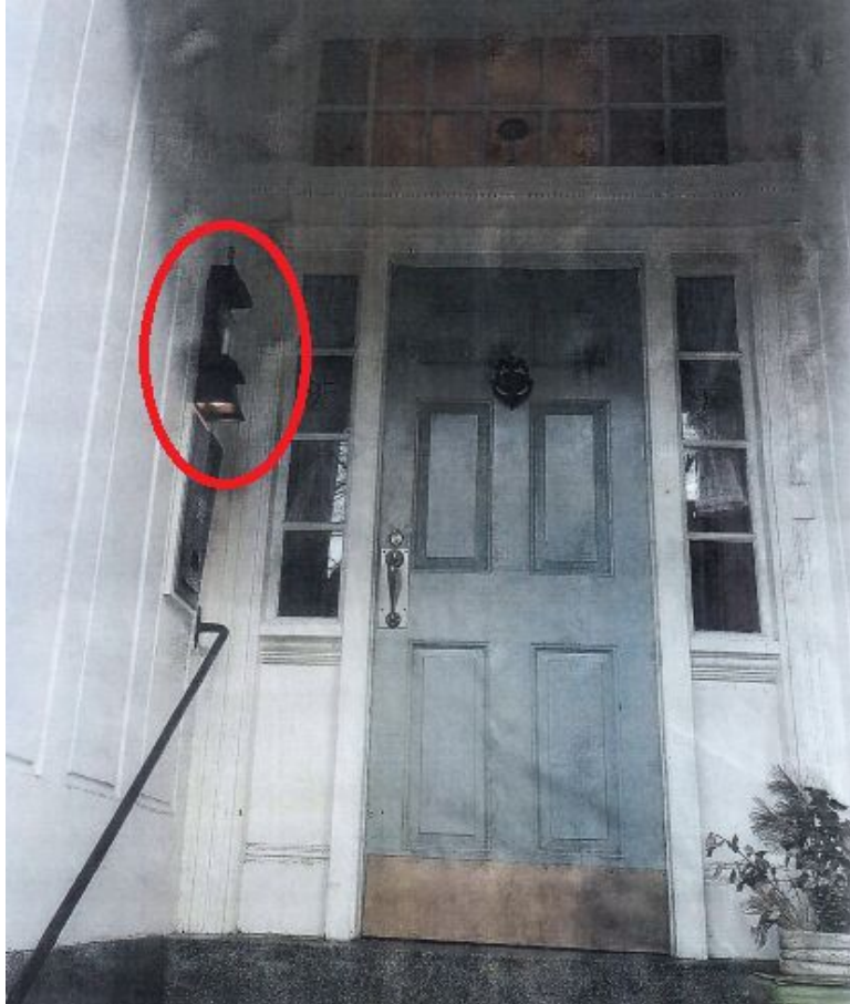
Mt. Vernon Entrance. Circle shows light to be replaced
