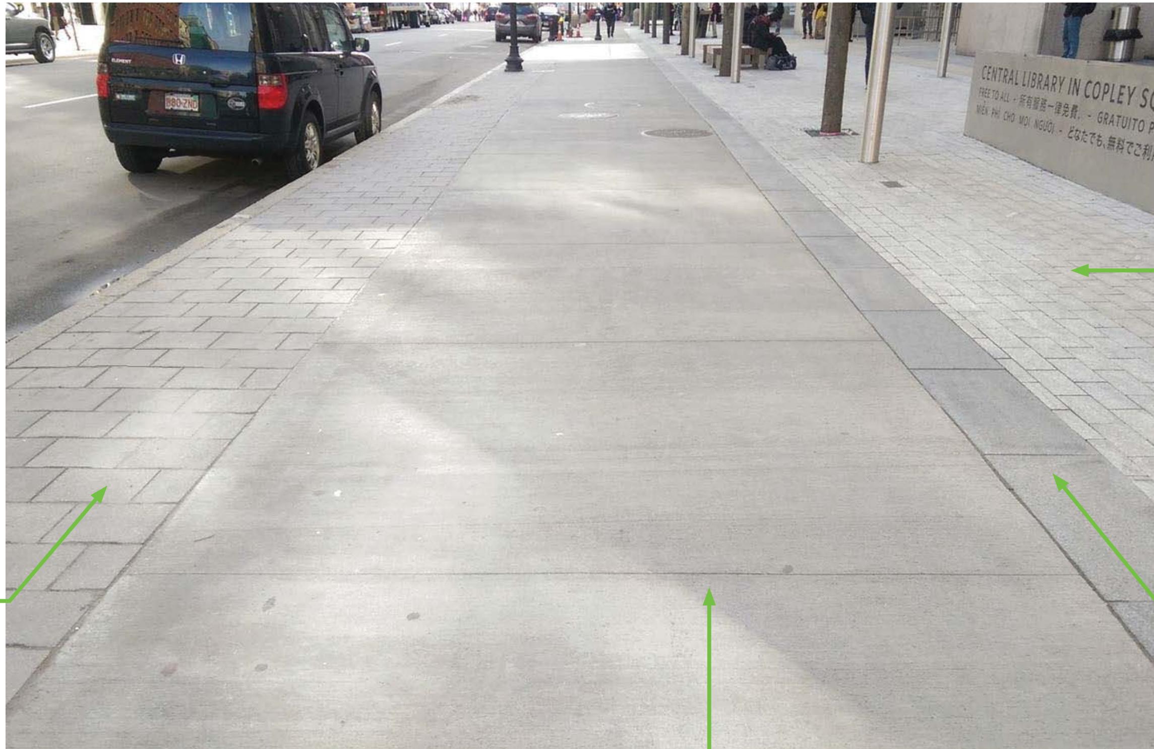
STANDARD CONCRETE SIDEWALK - PUBLIC
