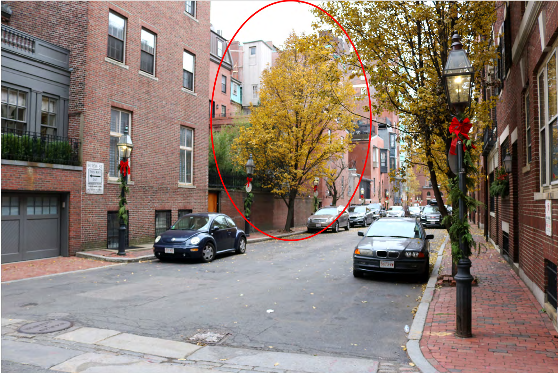
River Street - Existing Conditions
