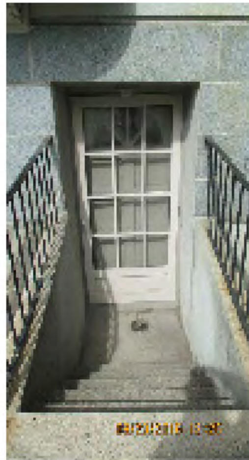
Front basement door, Beacon St.
