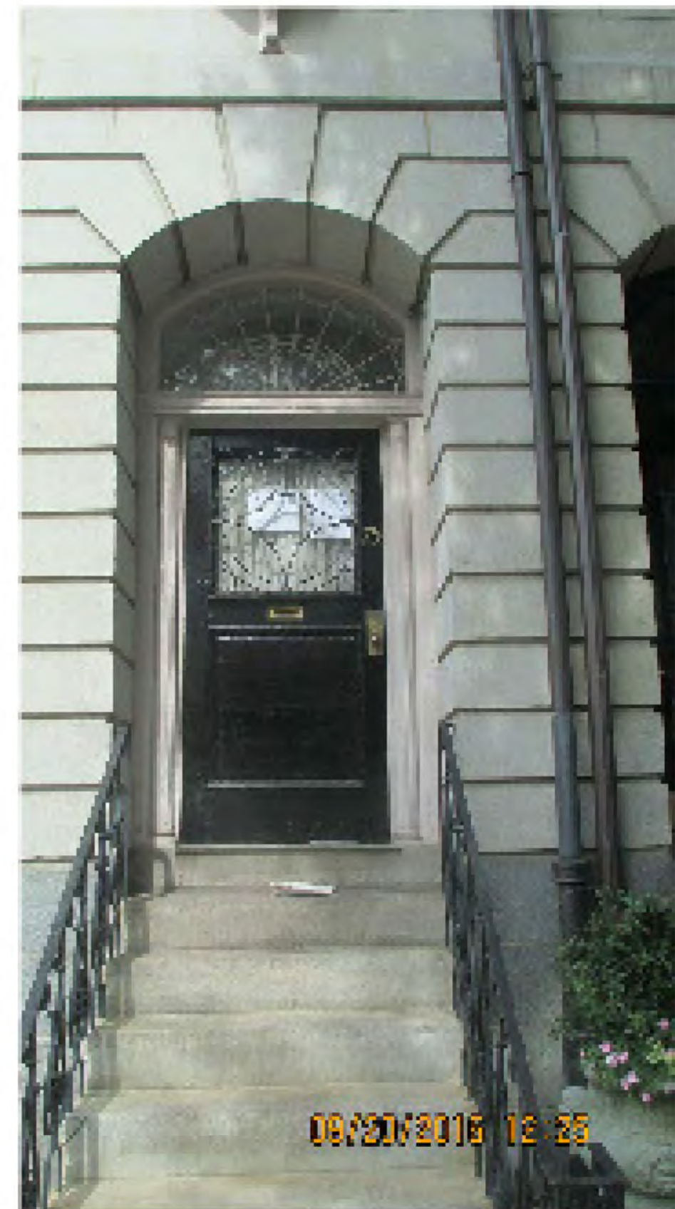
Front door, Beacon St.
