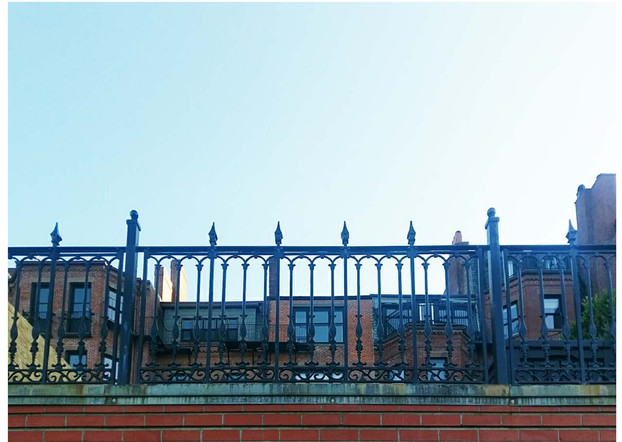
RAILING AT REAR OF 300 BEACON STREET
