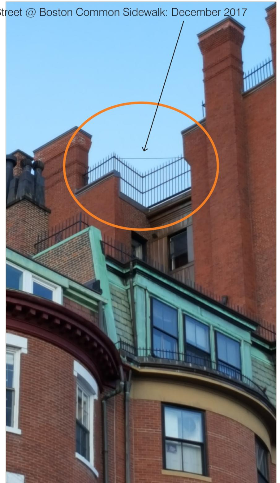
\*PLANTERS REMOVED IN JULY 2015 WITH BHAC APPROVAL FOR ROOF MEMBRANE REPLACEMENT
