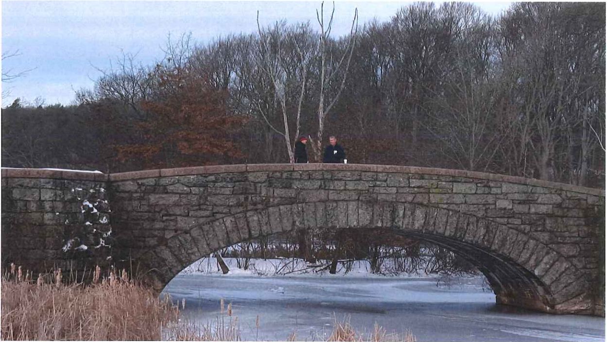
The iconic stone arch bridge. The new cart boardwalk will eliminate golf cart related traffic from this bridge and reestablish the historic bridge to pedestrian only traffic.
