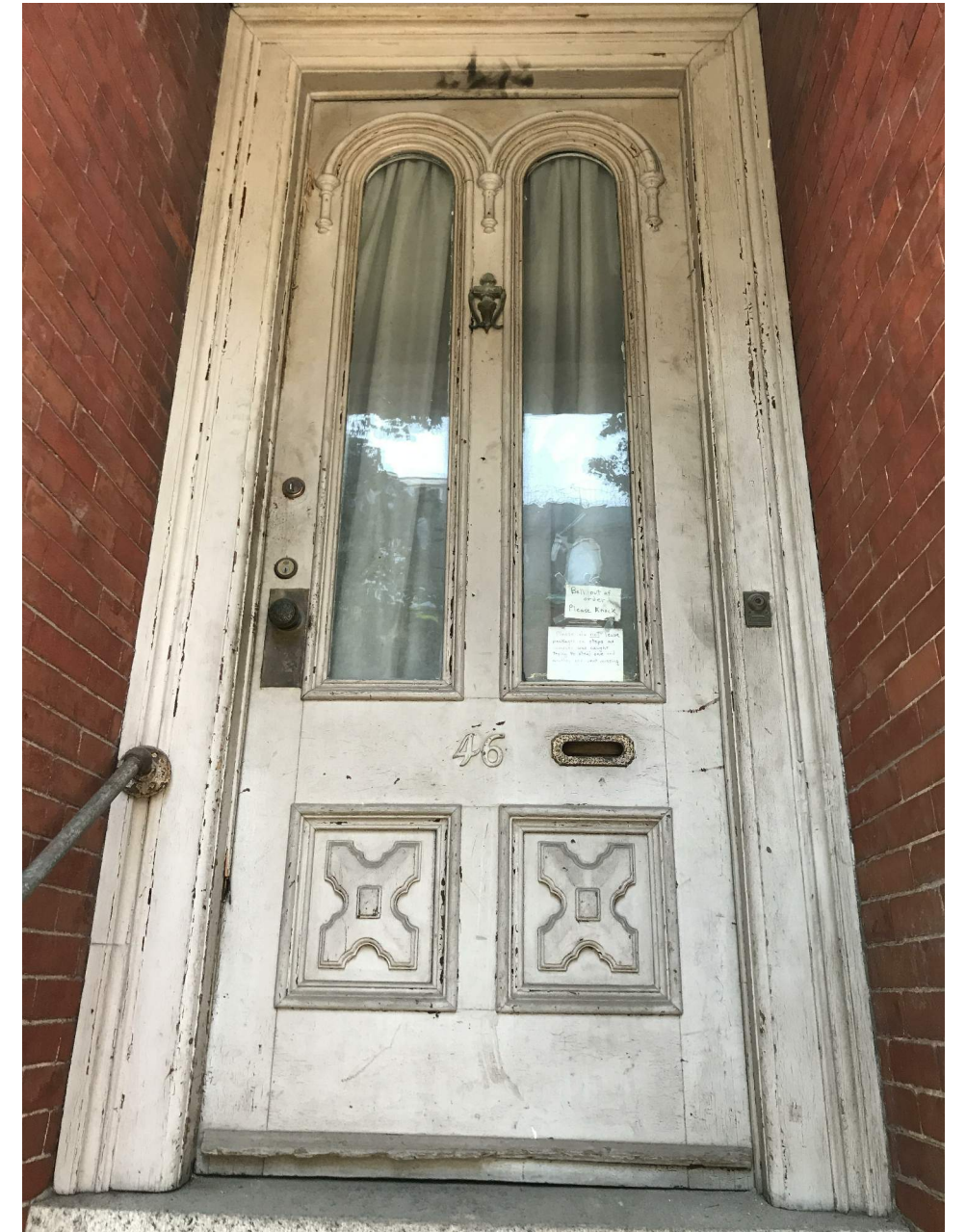
REPAIR AND RESTORE EXISTING FRONT ENTRY DOOR AND HARDWARE. INSTALL NEW PENDANT ENTRY LIGHT.
