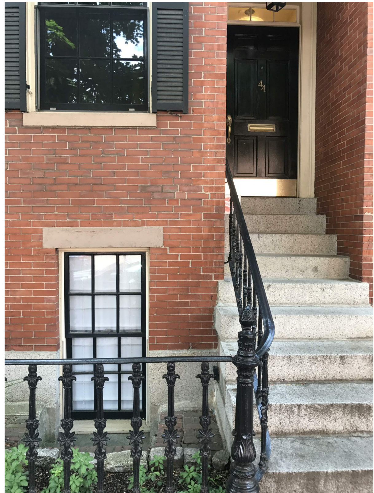
WINDOW WELL AT 44 CLARENDON STREET
