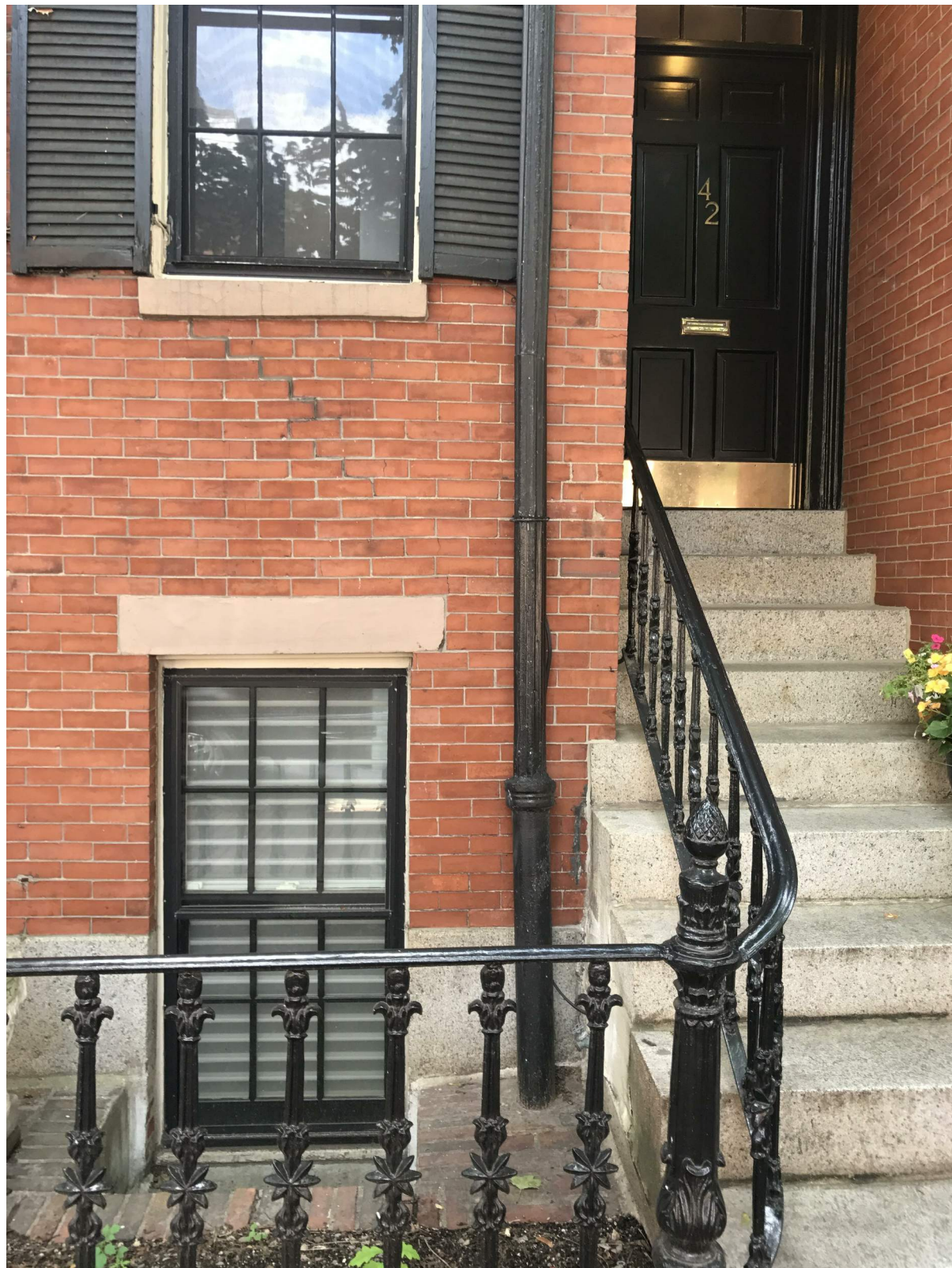
WINDOW WELL AT 42 CLARENDON STREET
