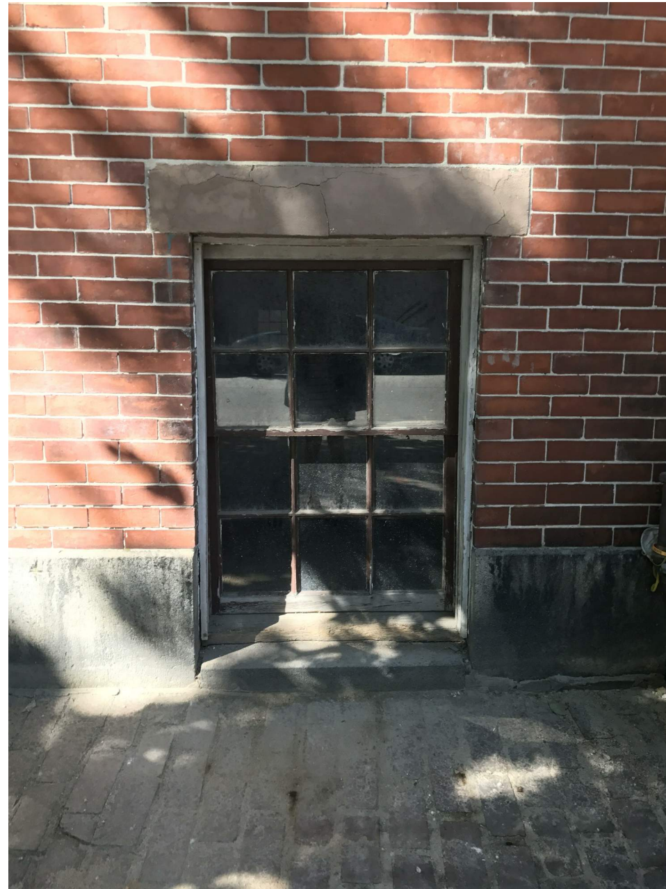
REPAIR AND RESTORE STONE SILLS AND LINTELS, AS REQUIRED. REPLACE WINDOWS WITH NEW PELLA ARCHITECT SERIES '6 OVER 6' WOOD WINDOWS CREATE NEW WINDOW WELLS TO MATCH NEIGHBORING WINDOW WELLS.
