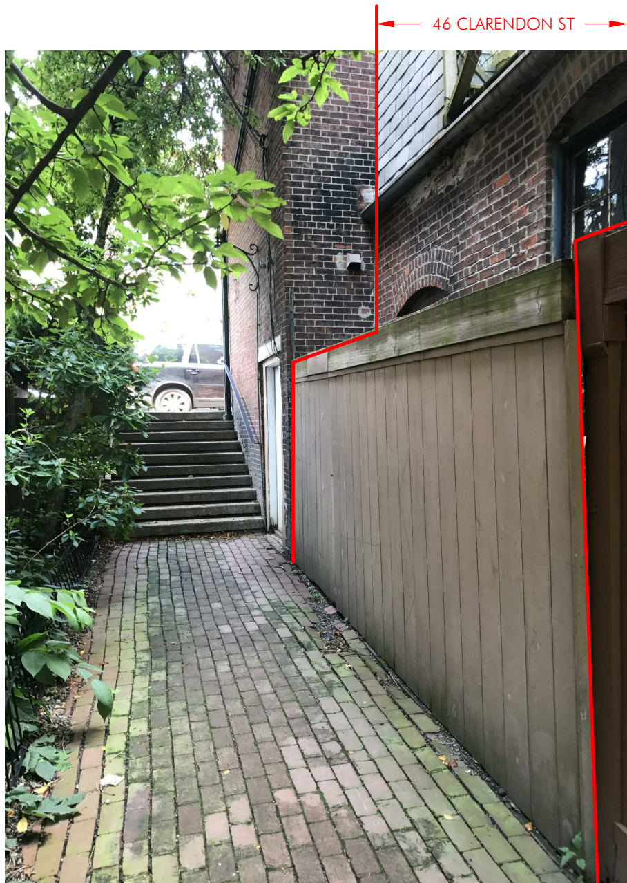
REAR ALLEY VIEW FACING APPLETON ST
