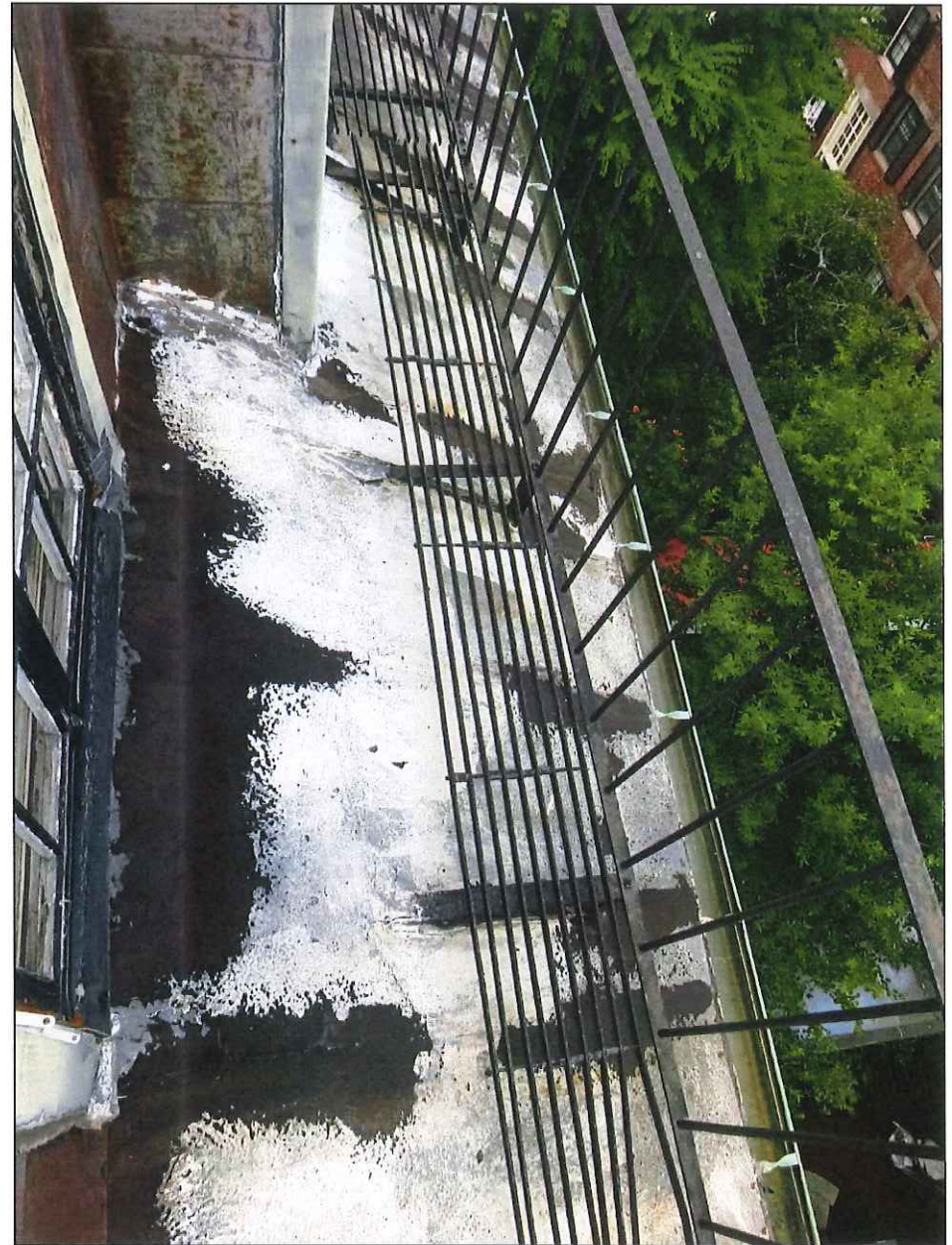
Typical sloped roof area
