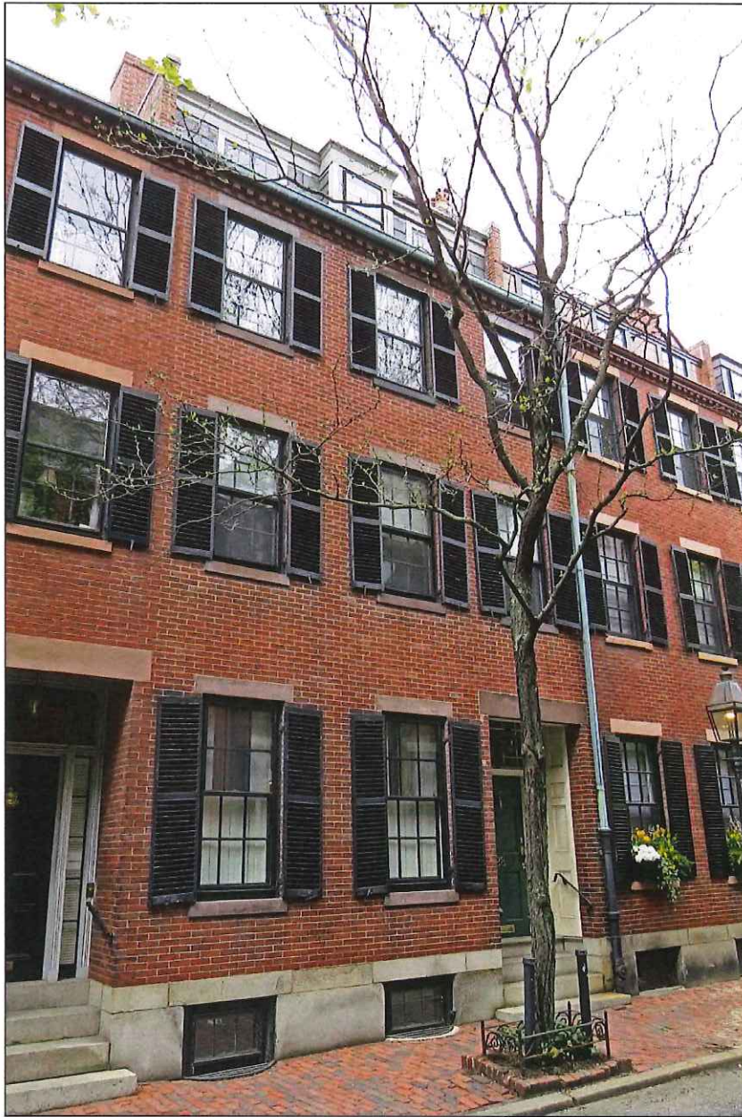
Front facade from West Cedar St.
