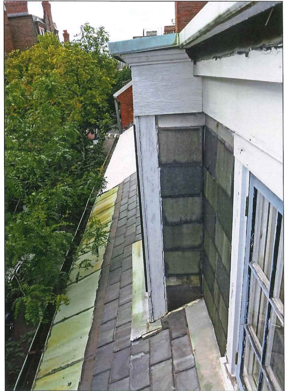
Front dormer area and center section
