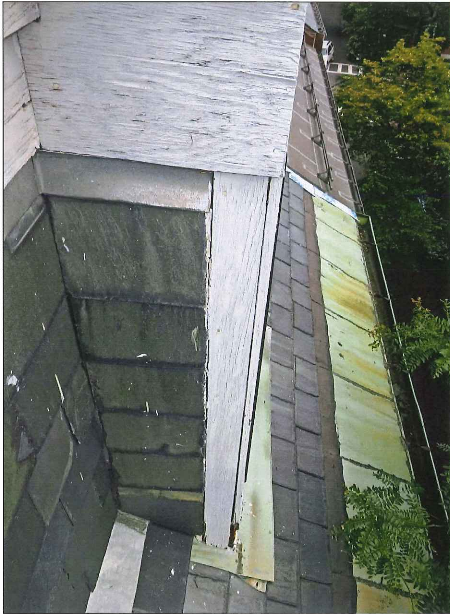
Front dormer area and center section
