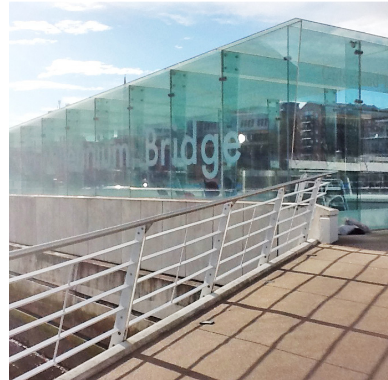
GATESHEAD MILLENNIUM BRIDGE, ENGLAND
