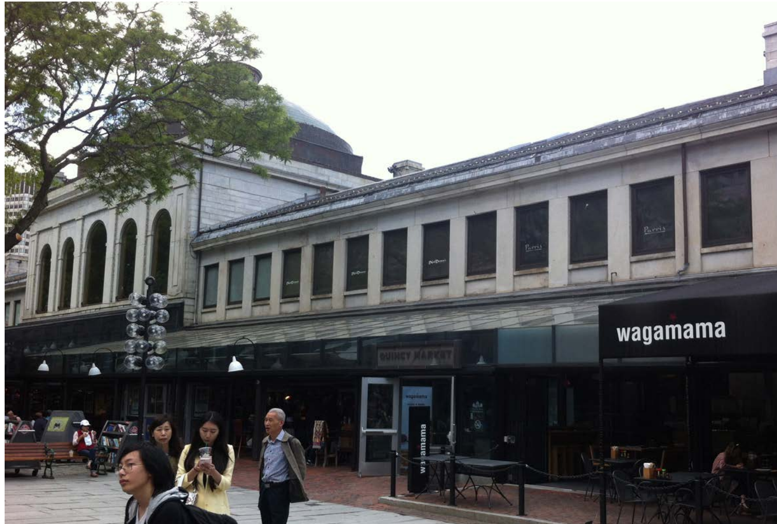
EXISTING CONDITION _ EXTERIOR _ LOOKING WEST
