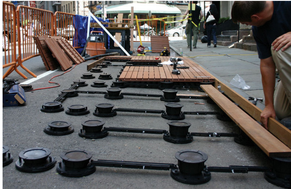
POP-UP PARK INSTALLATION
