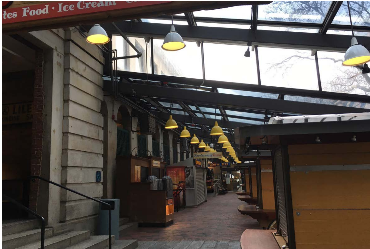
EXISTING CONDITION_ INTERIOR _LOOKING EAST
