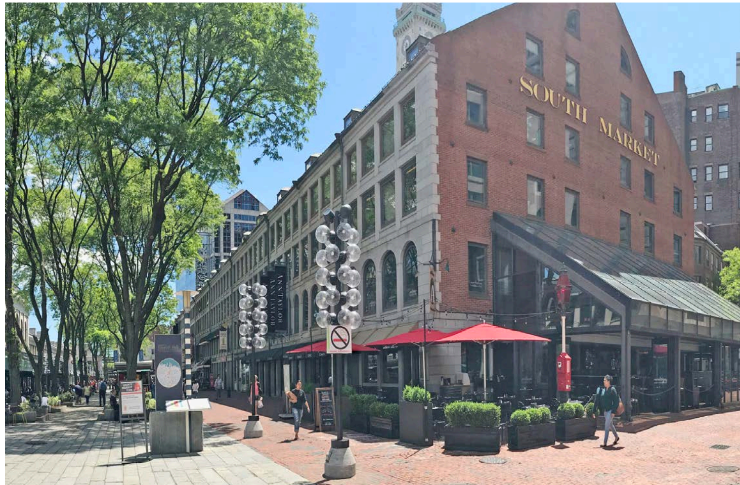
EXISTING - SITE PHOTO
