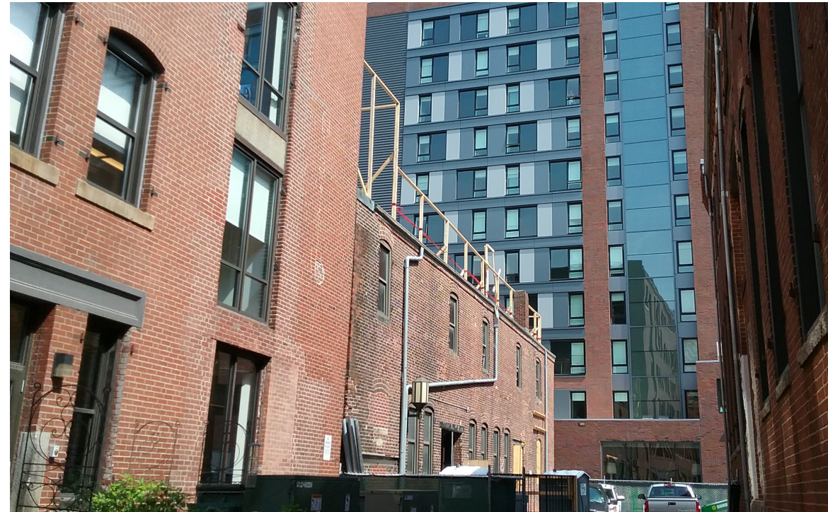
VIEW 2 - FROM PASSAGEWAY
