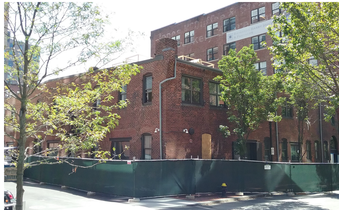
VIEW 4 - FROM STAIRS AT SEAPORT BOULEVARD
