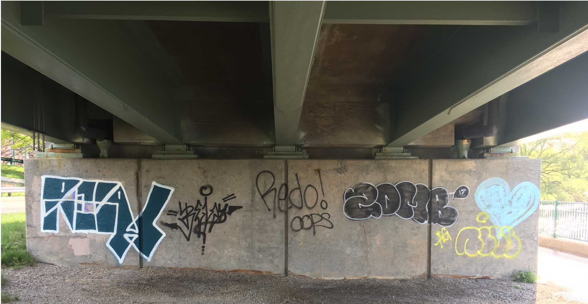
Low wall under the Storrow Drive West ramp; looking West.
