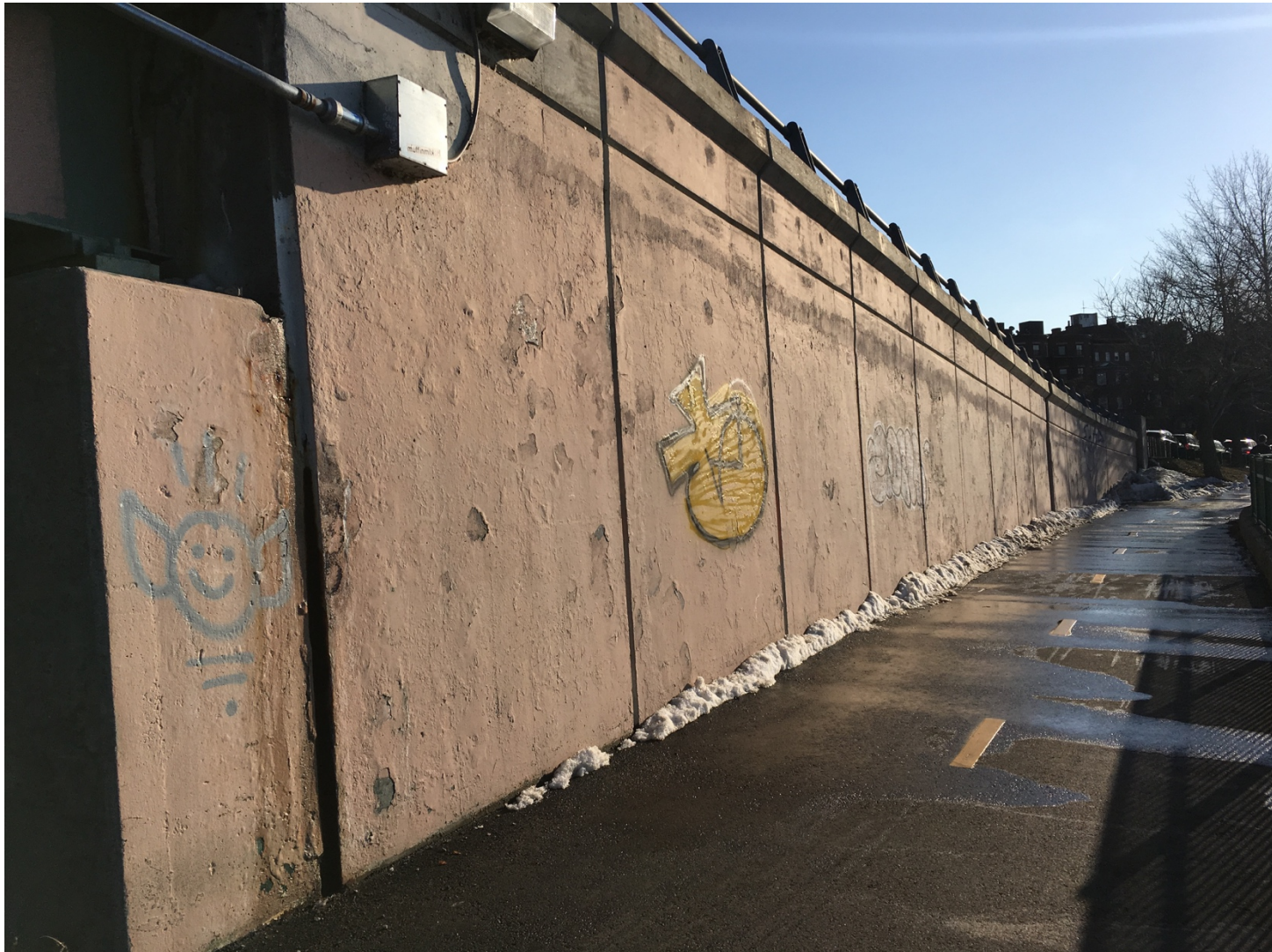
Storrow Drive West ramp wall; looking west.
