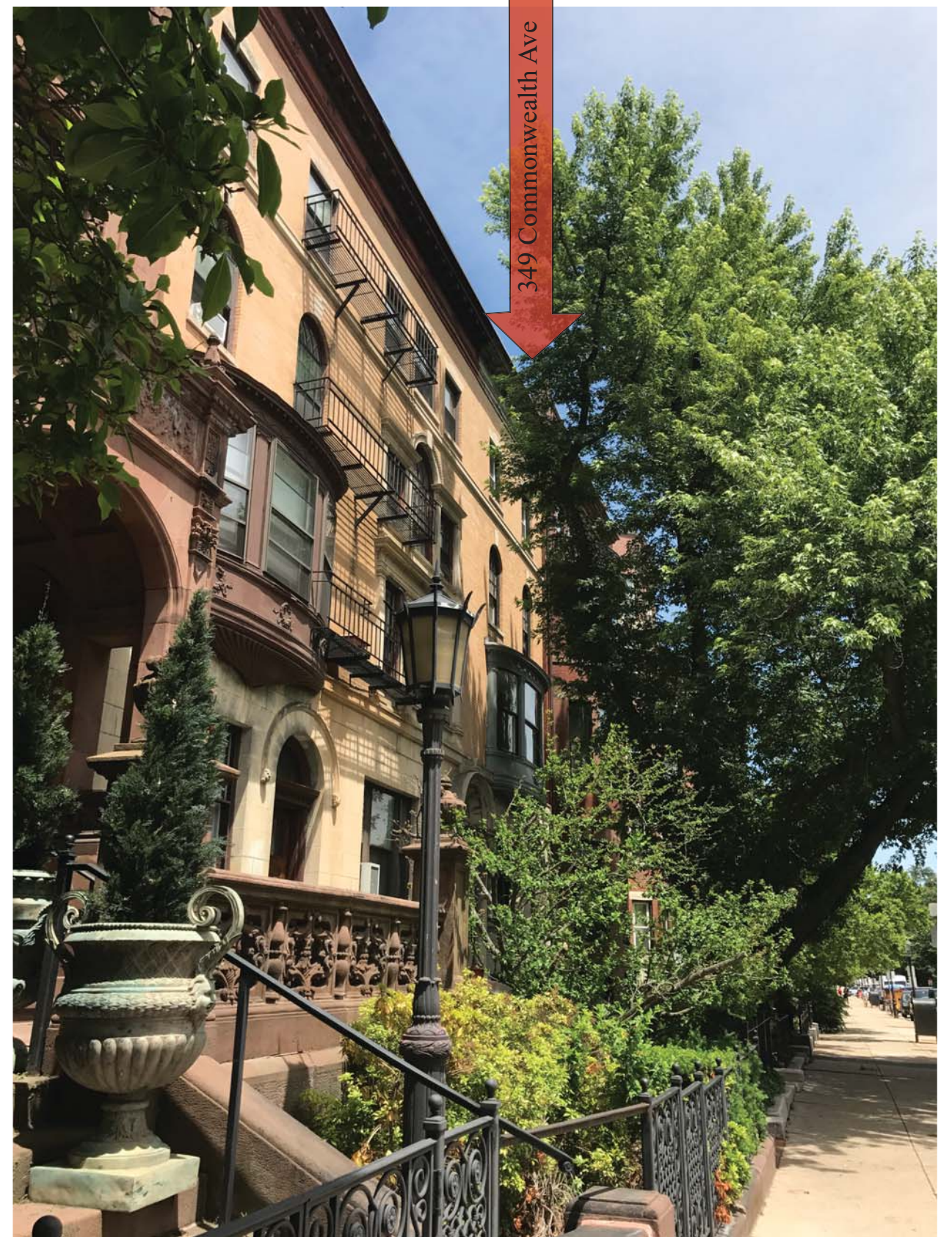
Mock-Up Looking North East on Commonwealth Ave
