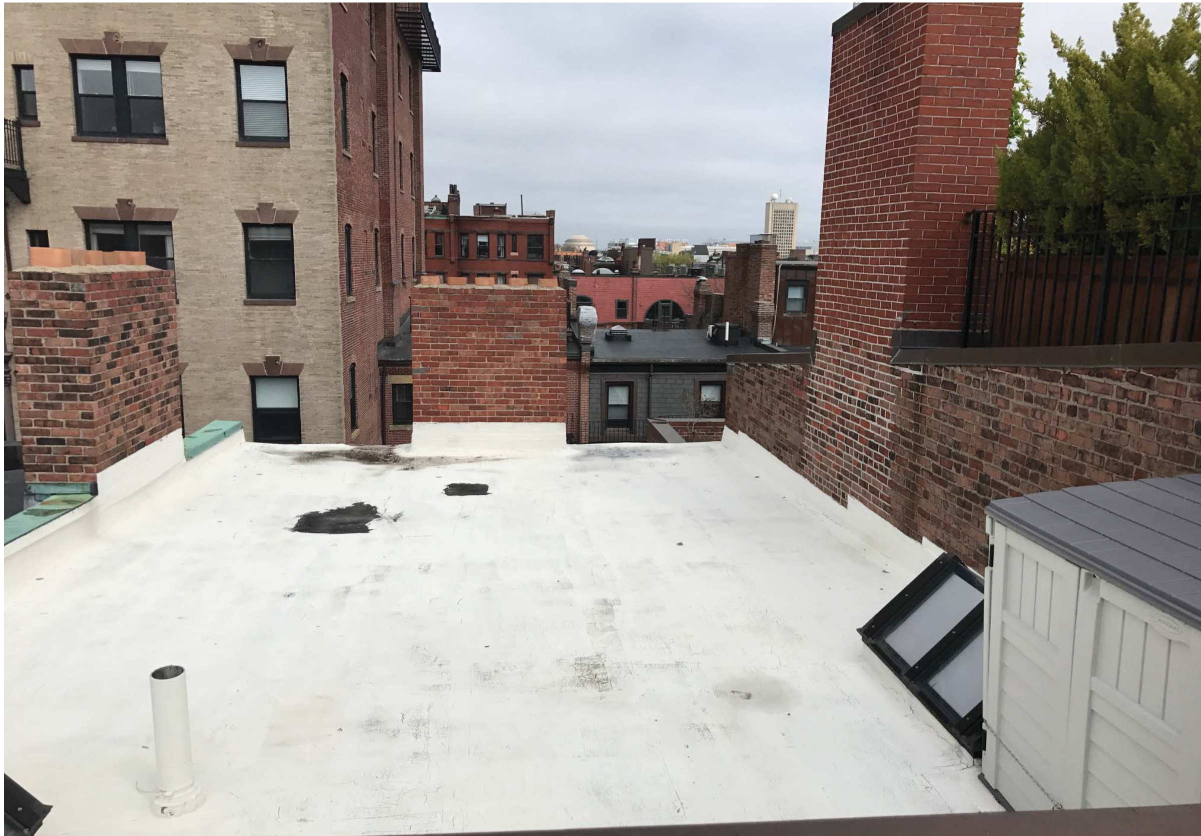
Existing Roof Looking North
