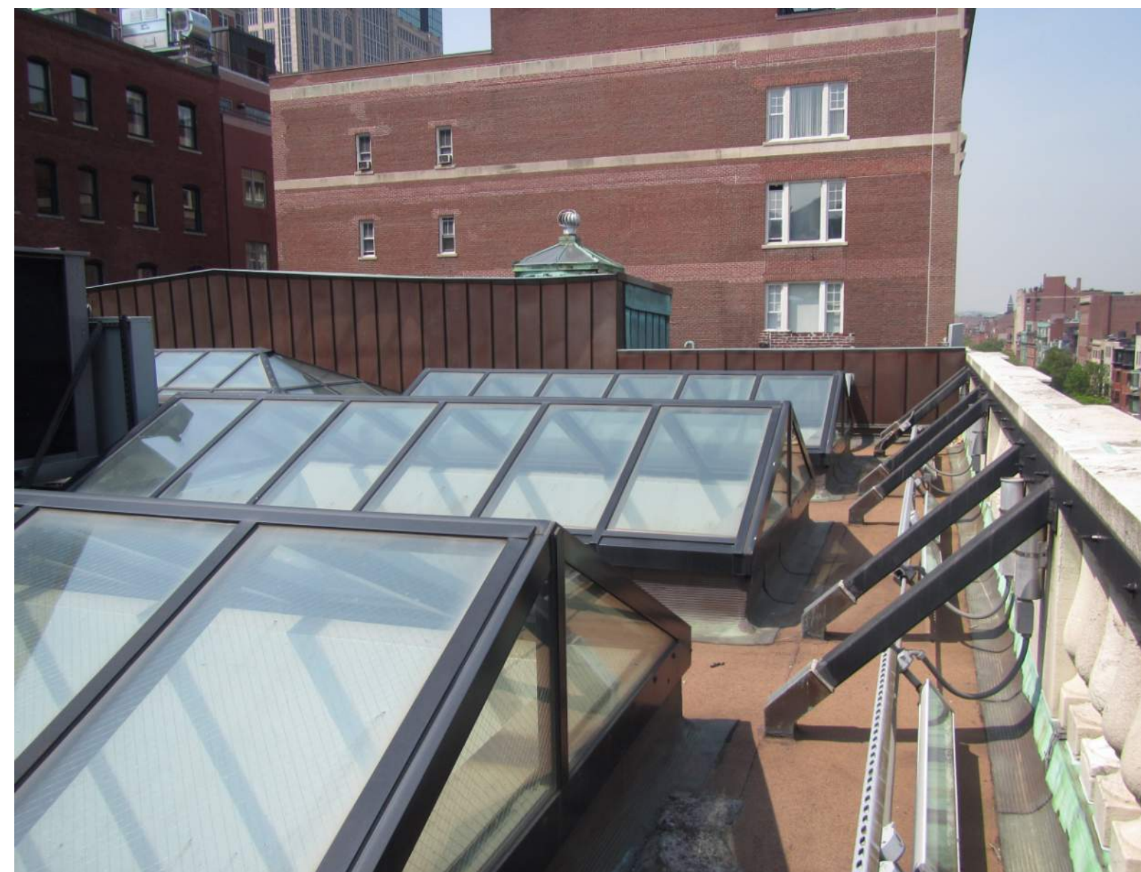
7: ROOF - EXISTING CONDITIONS
