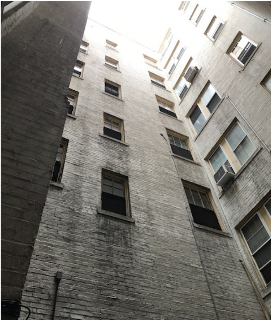
Existing wood windows - Part 2 (Above)
