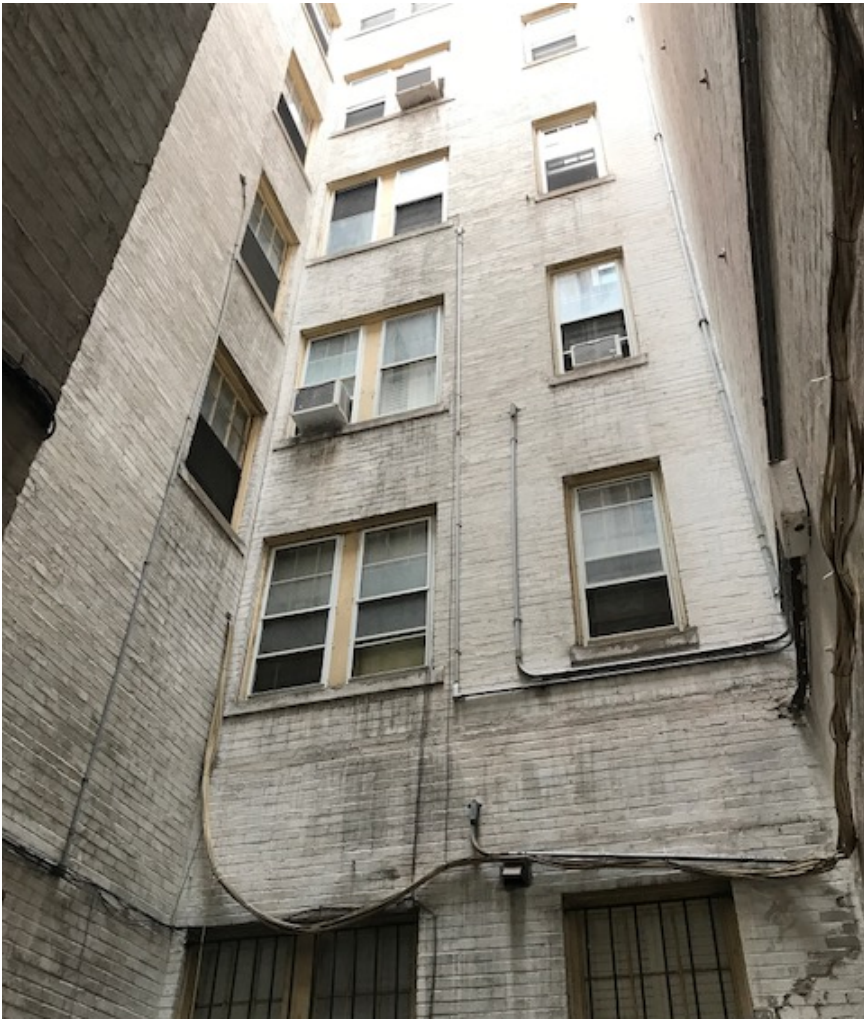
Existing wood windows (above)
