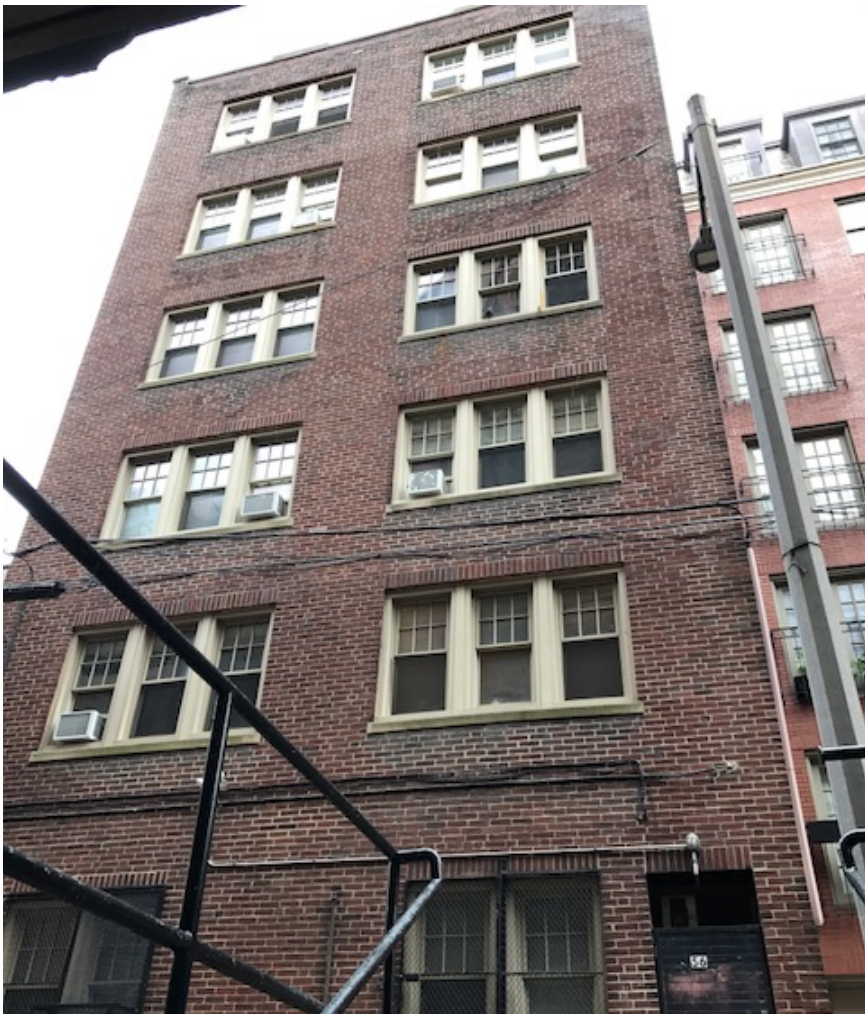
Rear of building: Also has Pella aluminum clad windows (~8 years old)
