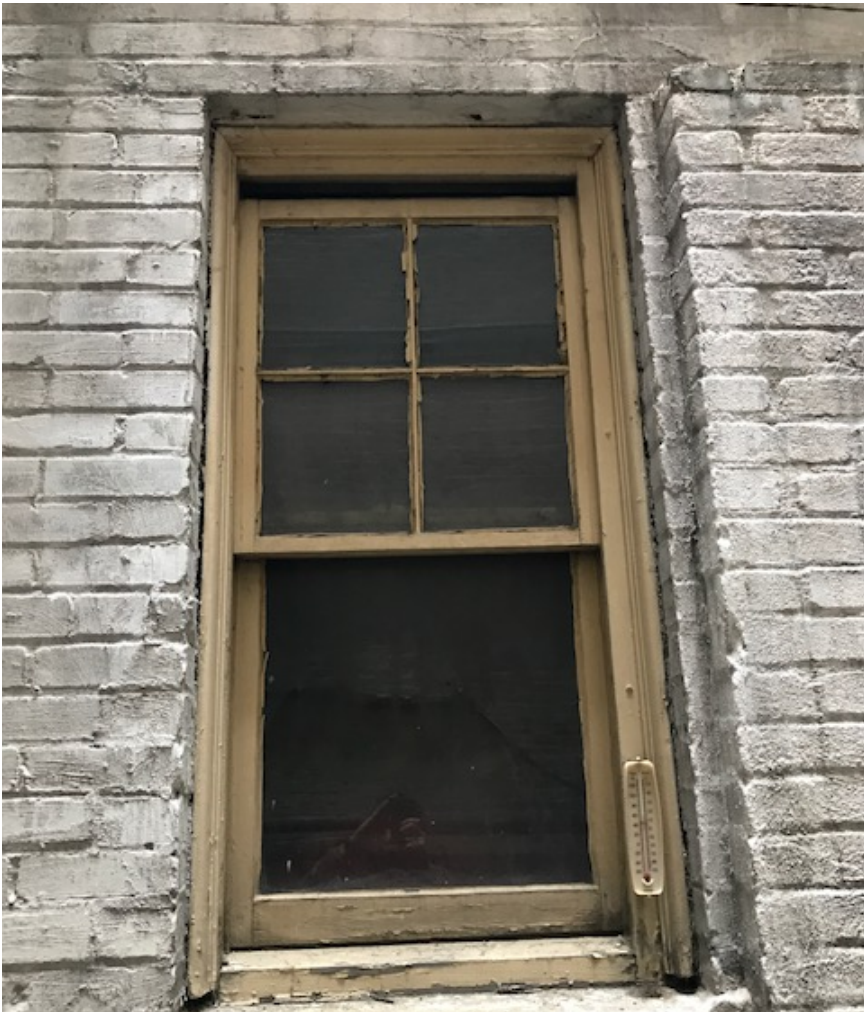
Existing wood window lite well
