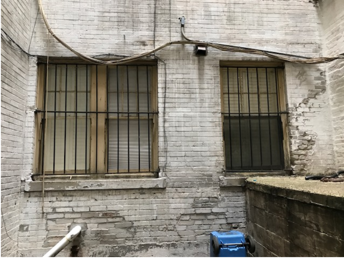
Existing wood windows in lite well
