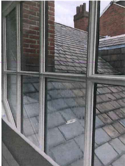
Polygon window to be replaced, interior view, roof angle.
